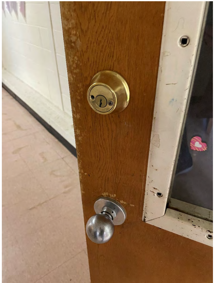
Insufficient Classroom Door Hardware – Does Not Meet ADA
