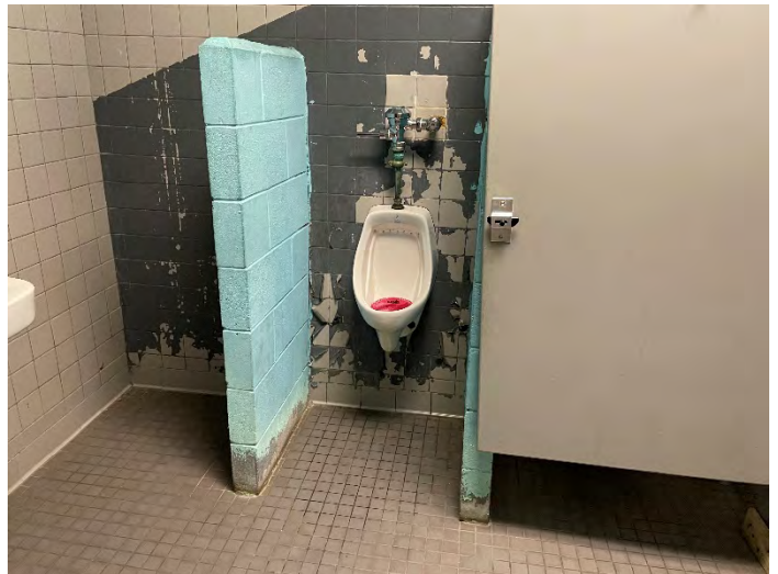
Paint Peeling In Bathroom
