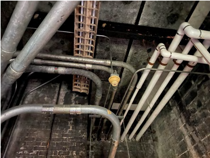
Code Violation – Smoke Detector Is Not Within 12" Of Deck Above
