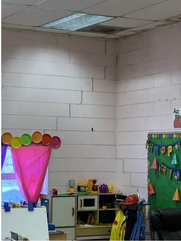
Minor Cracking of CMU Walls and Roof Leaks
