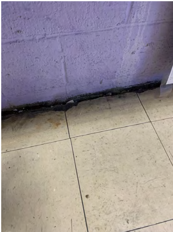
Large Gap Between Slab and Wall Adjacent to Bathroom
