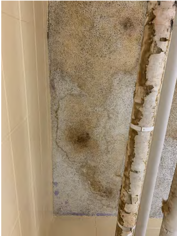
Water Staining of Tecktum Roof Decking
