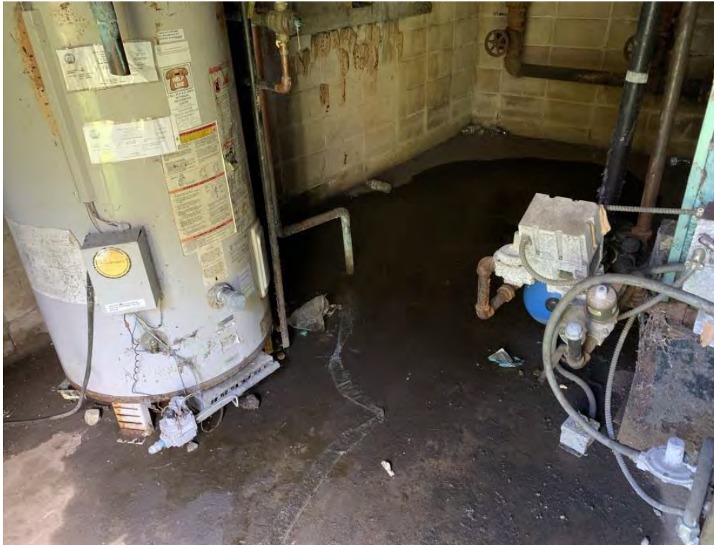
Water Ponding in Mechanical Room
