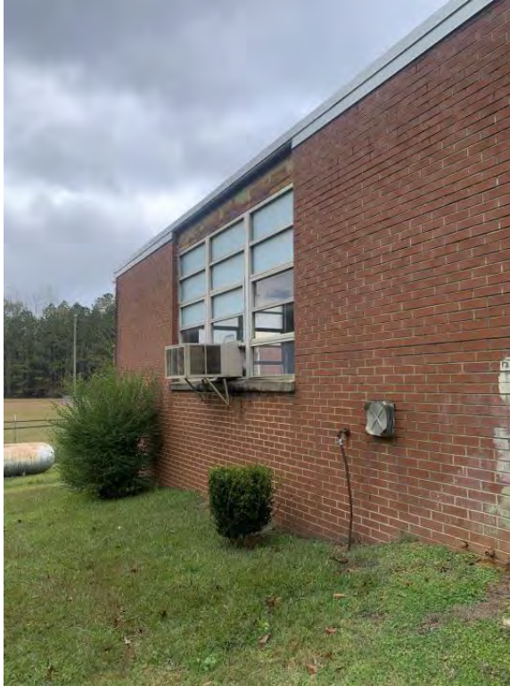
Missing Exterior Façade Over Window
