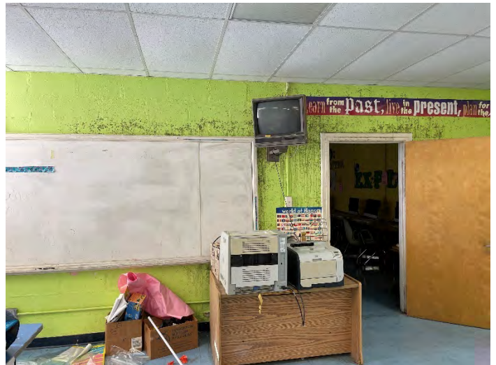
Mold Appears to Be Growing On This Wall
