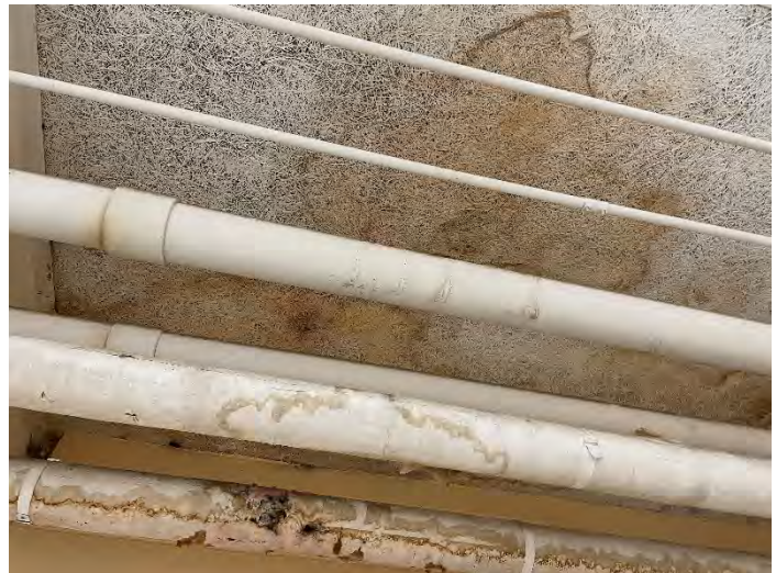
Roof Leak In Hallway
