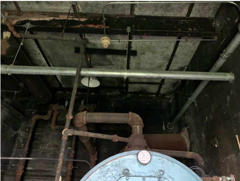
Deteriorated roof steel over mechanical room
