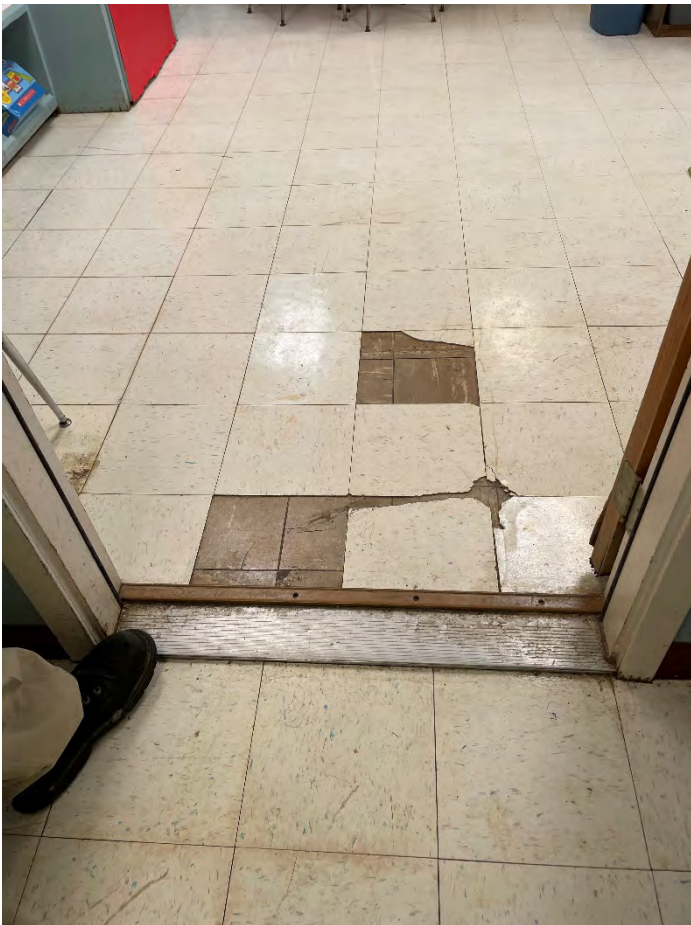
Example of Aged / Damaged Flooring That Causes Trip Hazard
