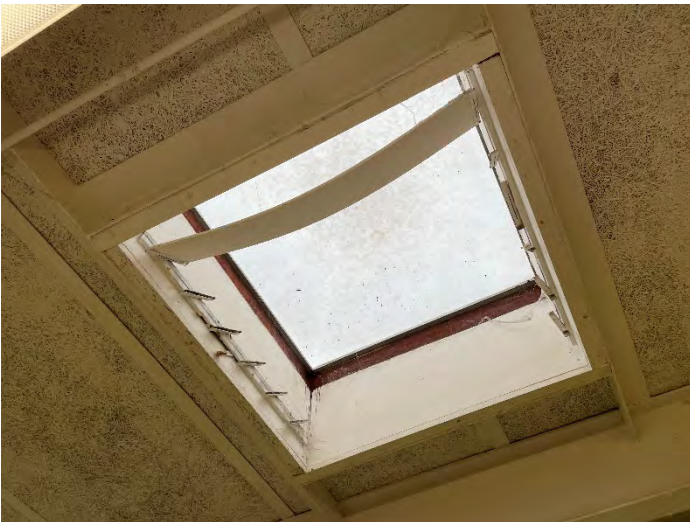
Old Skylights Showing Evidence of Moisture
