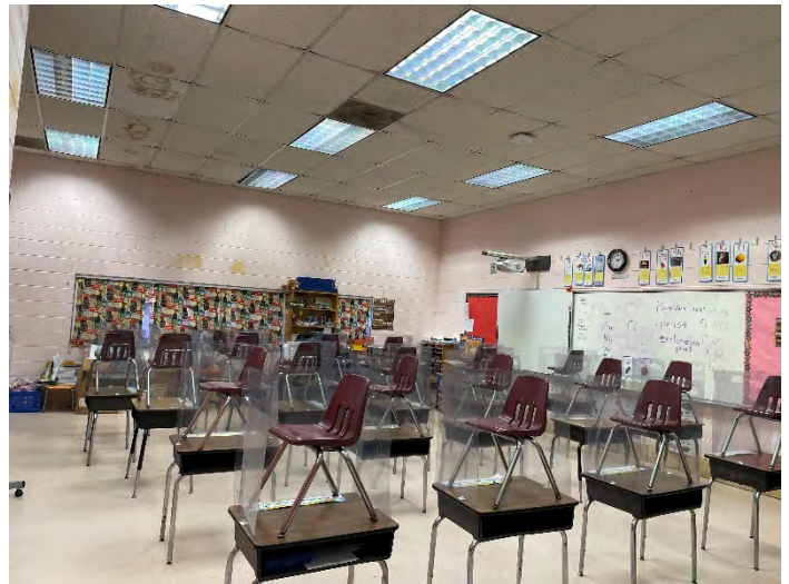
Dated Finishes & Evidence of Roof Leaks
