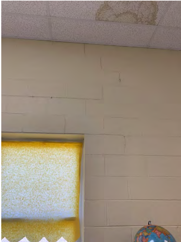
Minor Cracking in CMU Walls
