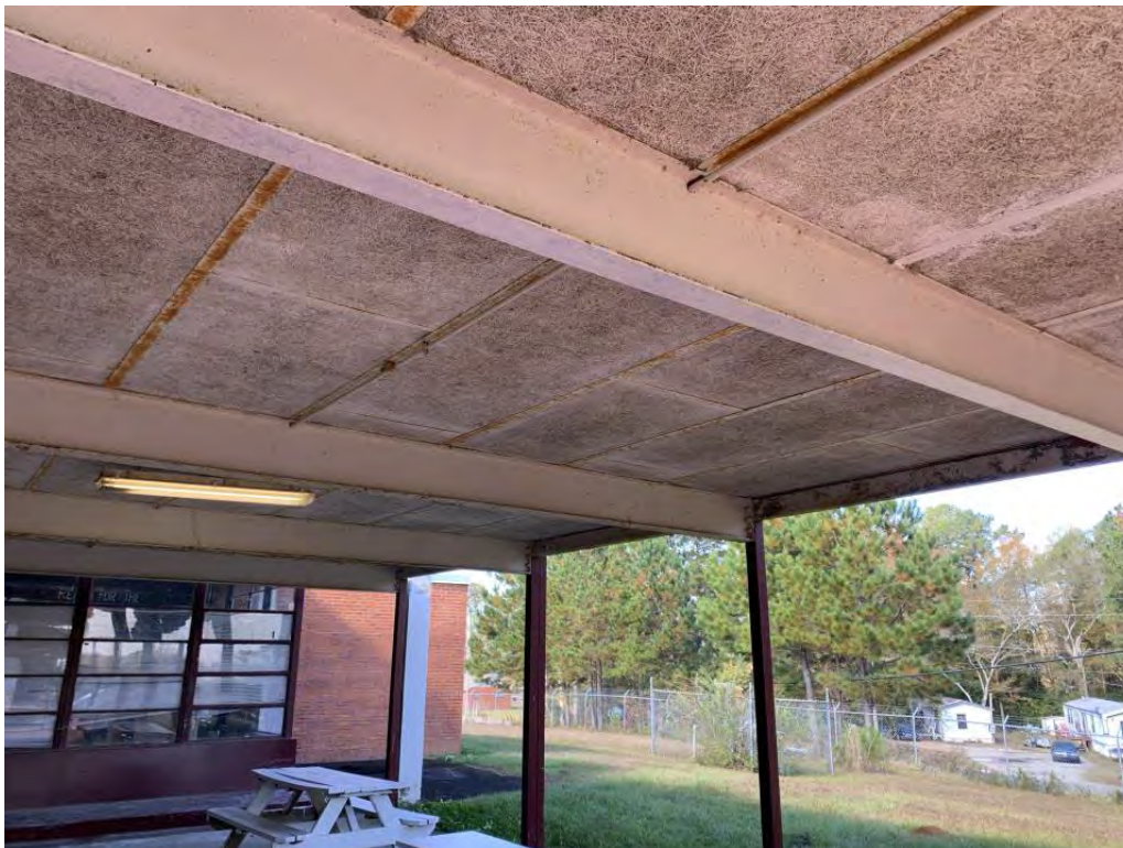
Minor Rusting of Exterior Roof Tees and Beams
