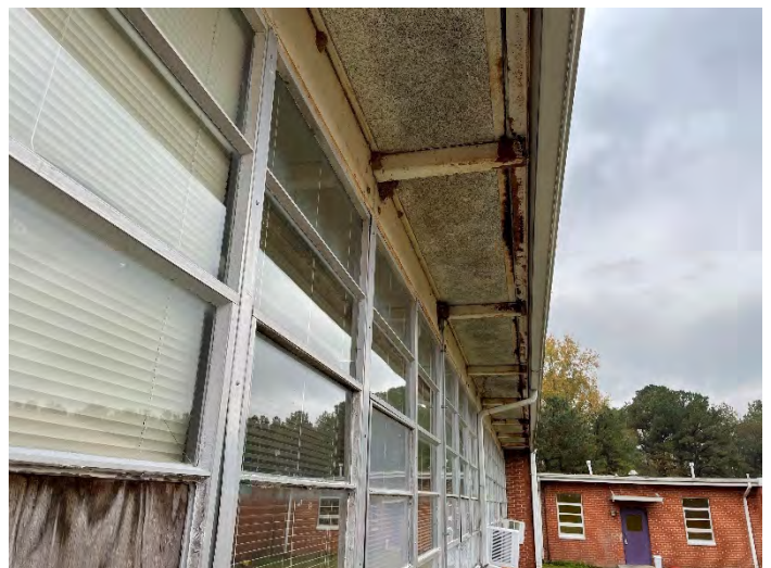
Aluminum Windows Are In Disrepair – Recommend Replacement
