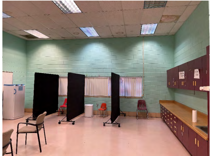
Dated Finishes & Evidence of Roof Leaks
