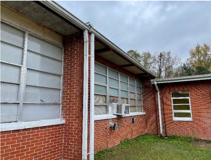
Tecktum Roof Deck Appears Damaged – Multiple Roof Leaks Observed
