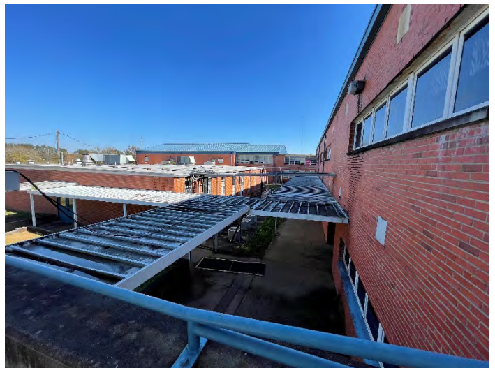
Canopies May Be Holding Water On Top
