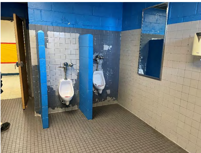
Example of Deteriorating Restroom Finishes
