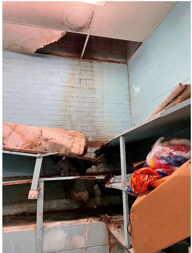
Water Damage From Extreme Roof leak In Band Room – Mold Is Evident – SAFETY HAZARD
