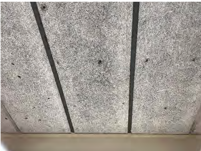
Areas That Have Been Re-Roofed Have Toggle Anchors Exposed
