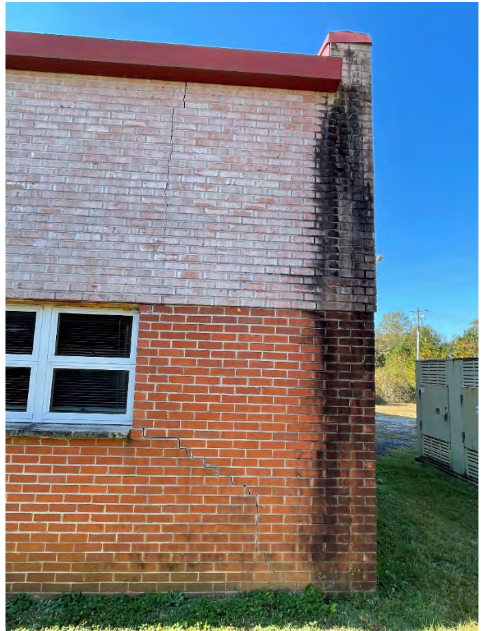
No Drainage in This Courtyard
