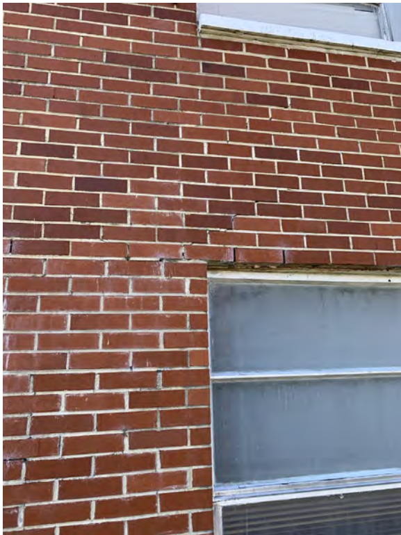
Minor Cracking in Exterior Brick Facade
