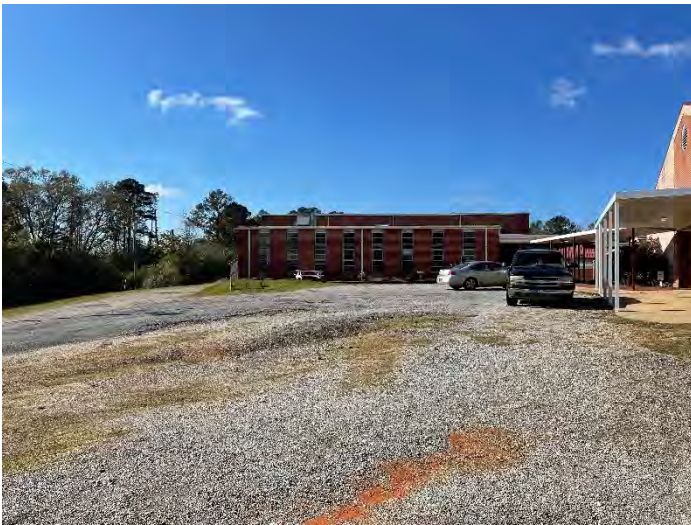
Example of Ruts / Washing In Gravel Lot
