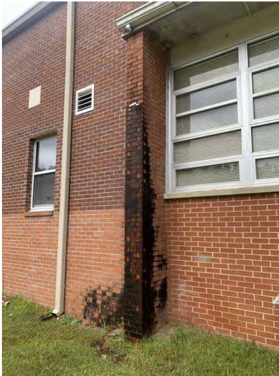
Gutters and Splash Guards Missing
