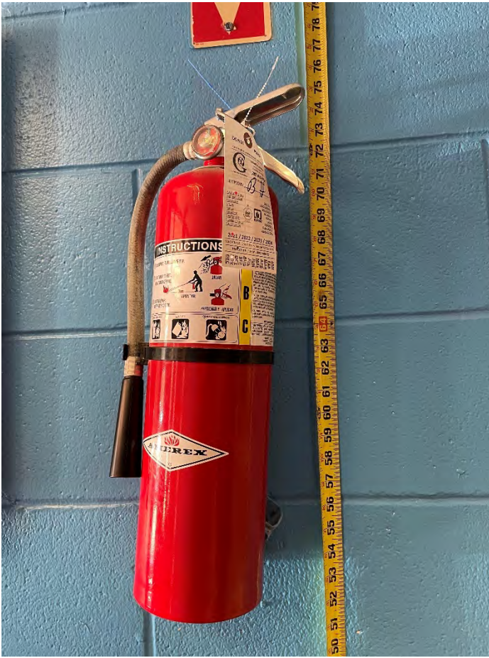
Example of Pull Stations, Light Switches & Fire Extinguishers Above 48"
