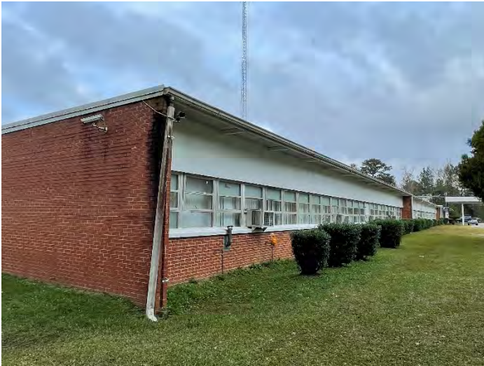
Grade Holds Water Against Building In Some Locations
