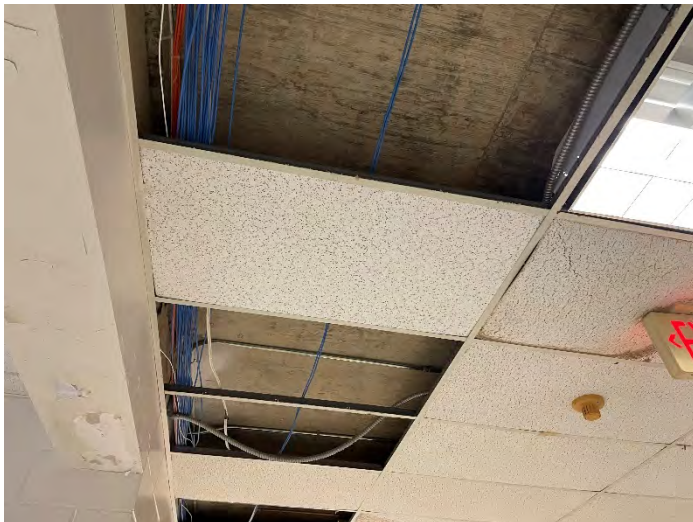
Ceiling Tiles Out – Leaks Reported
