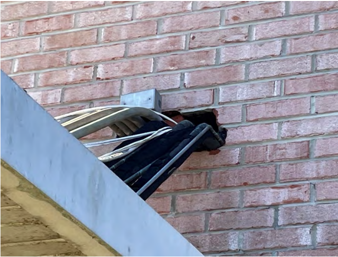
Example of Unsealed Penetration
