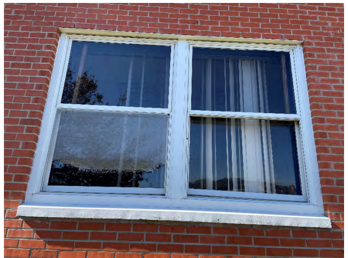
Broken Glass at Front Elevation
