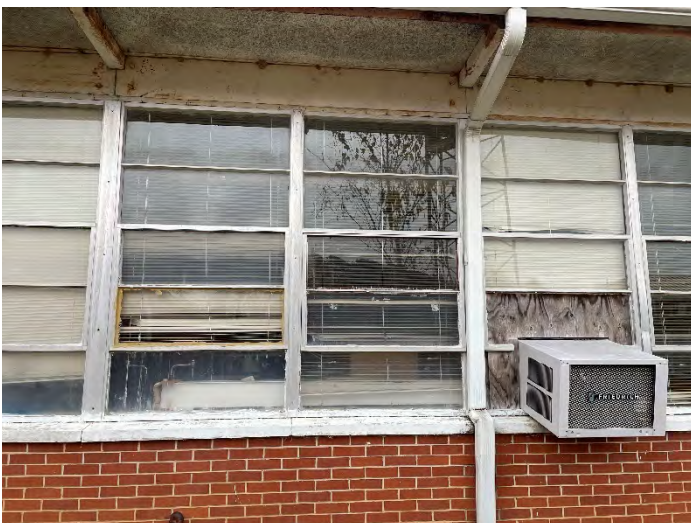
Aluminum Windows Are In Disrepair - Recommend Replacement
