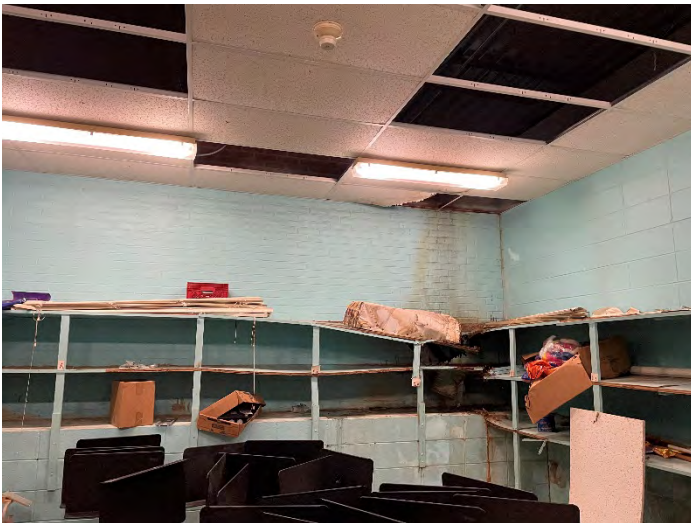
Water Damage From Extreme Roof leak In Band Room – Mold Is Evident – SAFETY HAZARD
