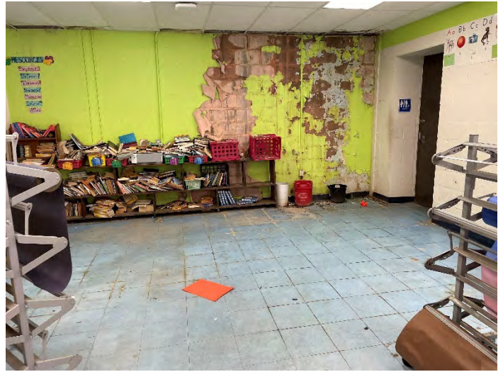
Roof Leak Causing Water Damage & Mold
