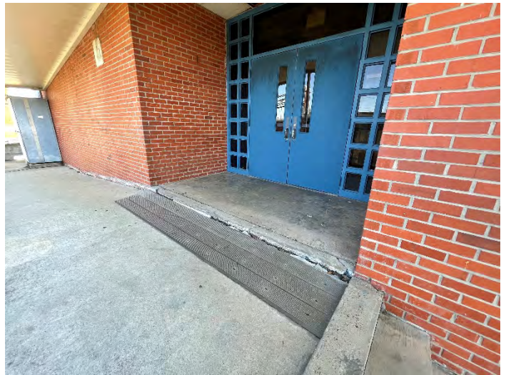
Example of Trip Hazard at ADA Egress Door
