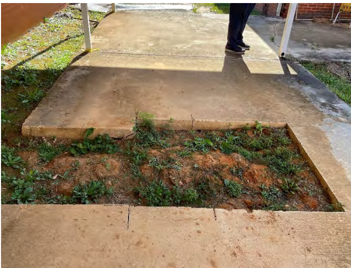
Example of trip Hazard at Exterior Walkway
