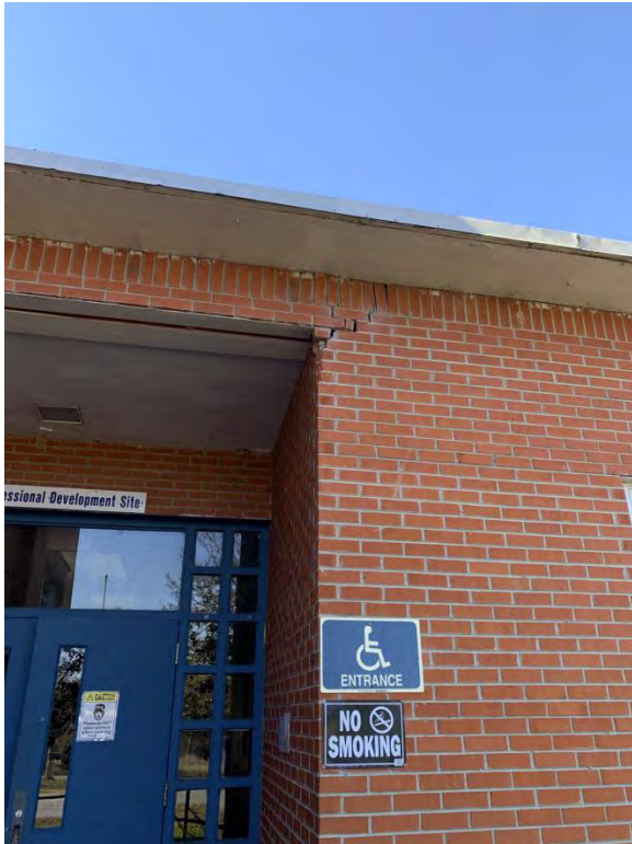
Cracking of Brick Façade at Front Entry
