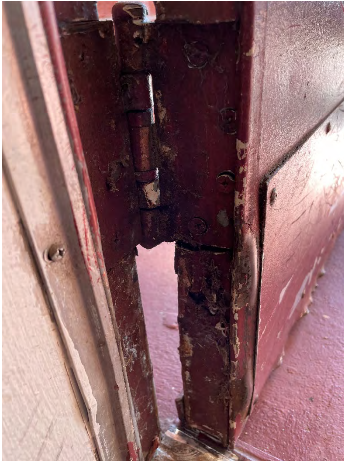
Example of Aging Door Hardware
