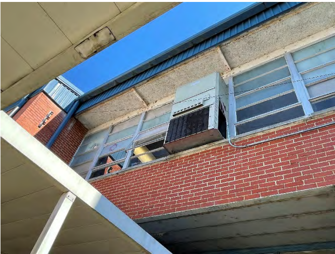
Bard HVAC Units Are 30 Years Old & In Disrepair
