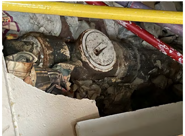
Maintenance Rep Reports Deteriorating Sewer Pipes
