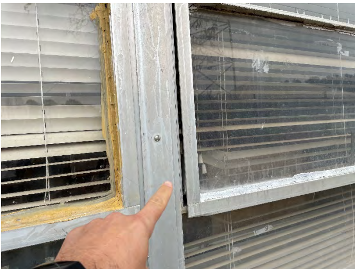
Aluminum Windows Are In Disrepair - Recommend Replacement
