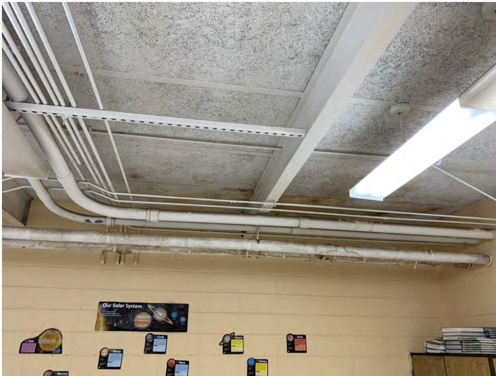
Water Staining of Tecktum Roof Decking
