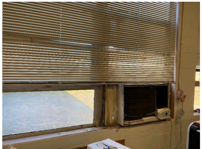
Air Conditioning is Achieved By Older Window Units
