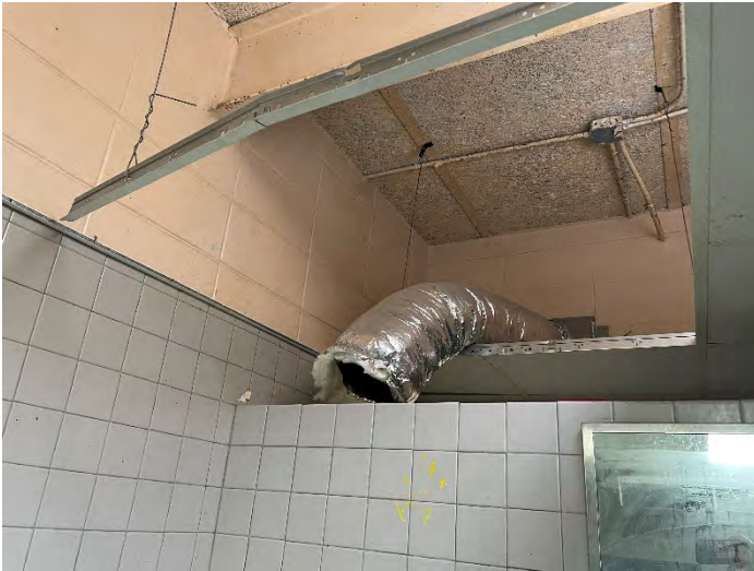
Ceilings / Duct Work Have Been Disassembled
