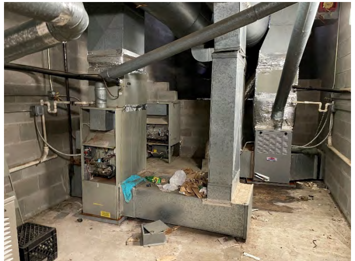
Covers Off HVAC Units on Mechanical Mezzanine Needs Cleaning
