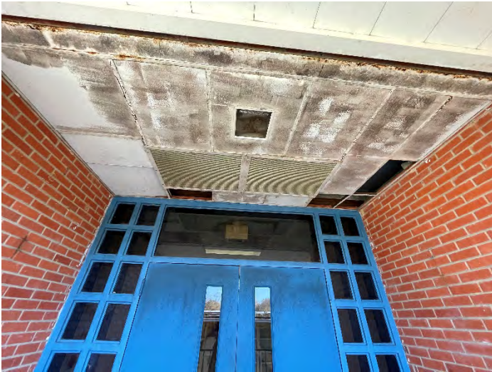
Exterior Soffits Such As This Need New Tiles
