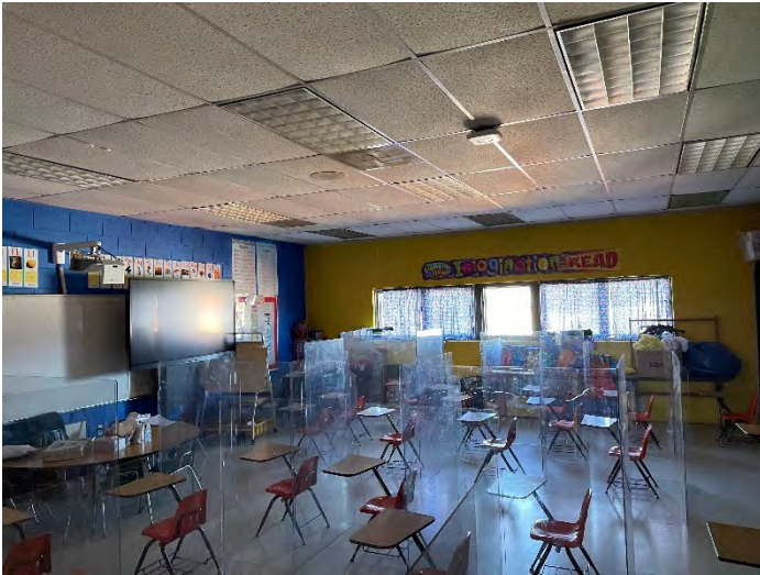
2 x 4 Ceiling Tiles are Starting to Sag
