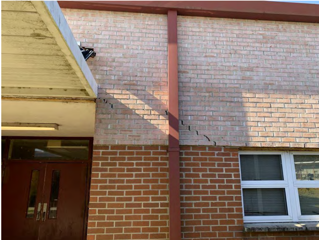
Cracks in Exterior Brick Façade
