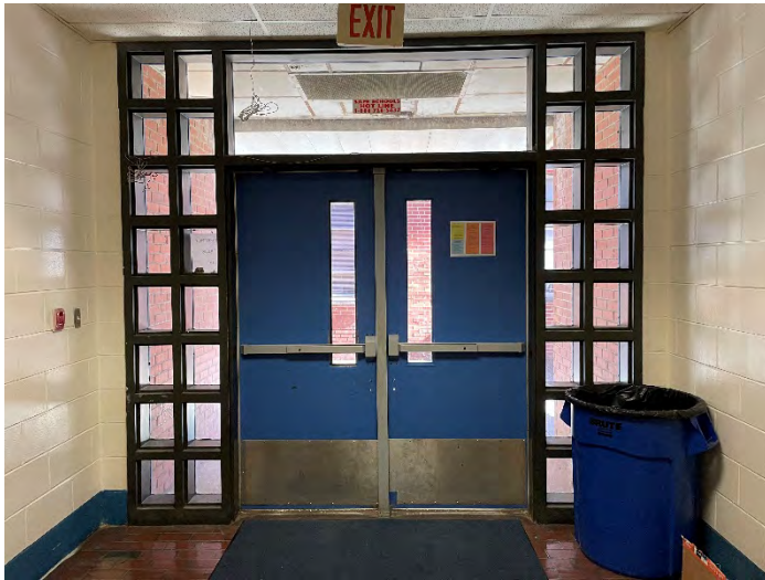
Most Egress Doors Require Adjustment
