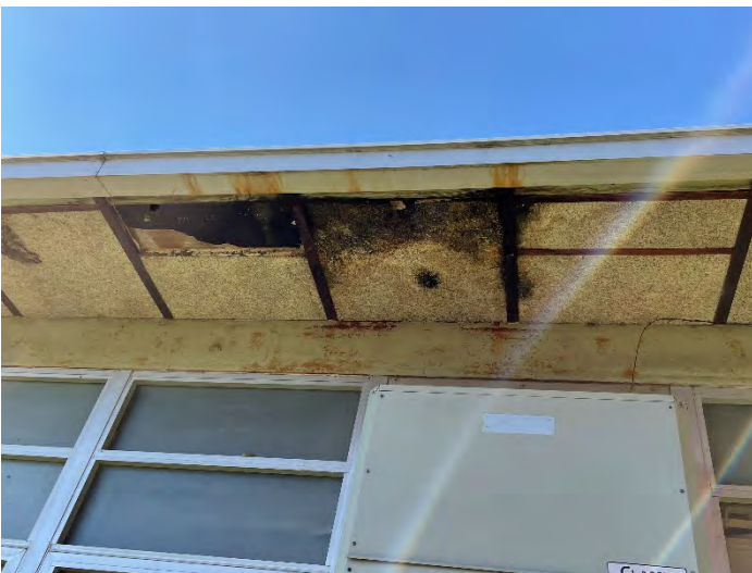
Example of Deteriorating Tecktum Deck
