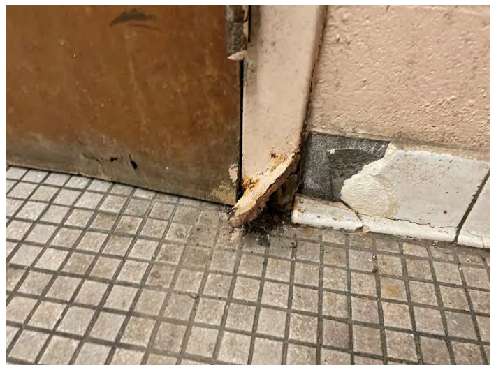
Example of Metal Door Frames Rusting On Bottom
