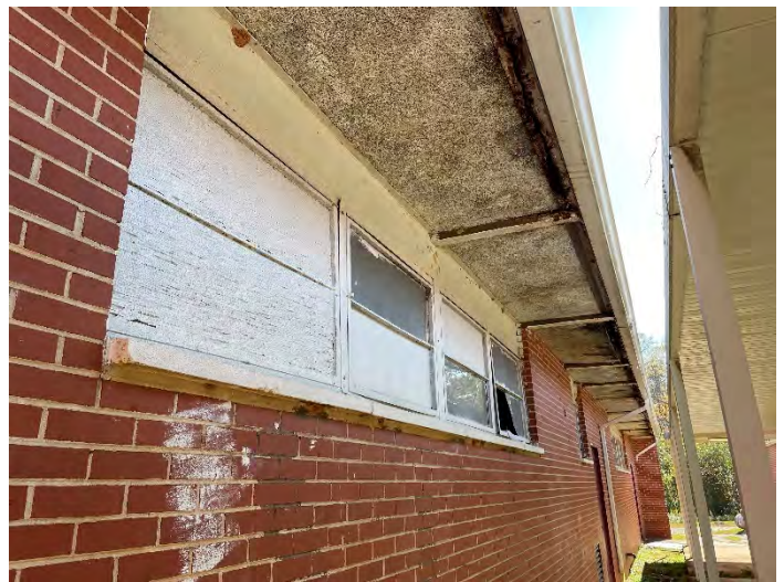
Tecktum Deck Deterioration At Perimeter
