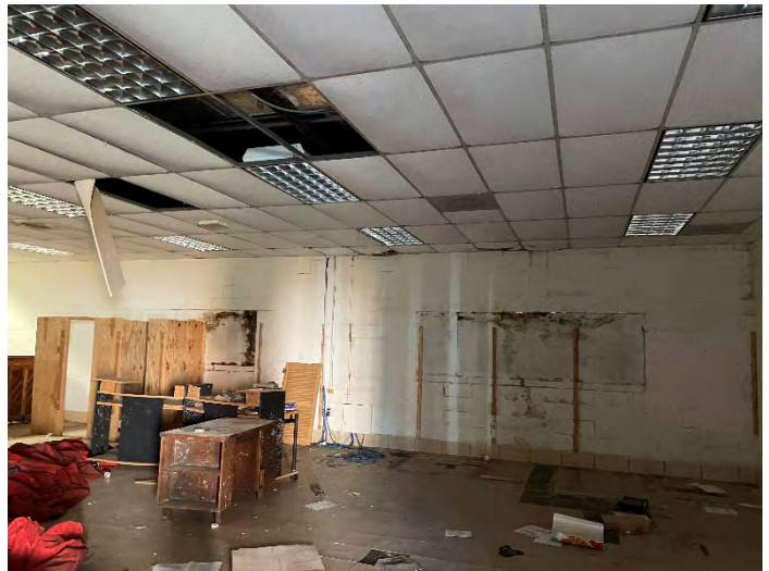
Dilapidated Shop Building – Mold Evident
