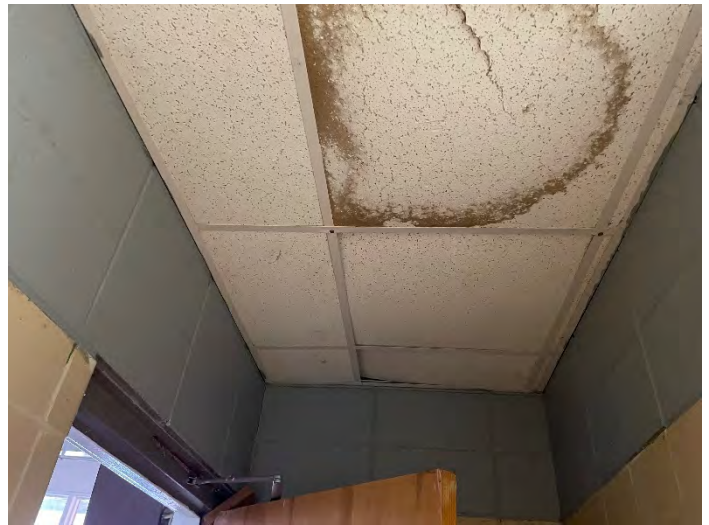
Example of Roof Leaks Throughout Campus
