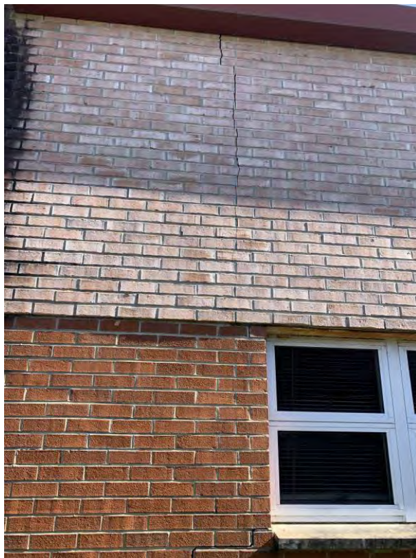
Cracks in Exterior Brick Façade
