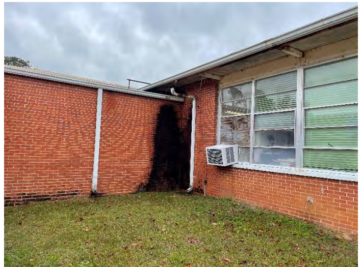
Most Gutters / Downspouts Are In Disrepair
