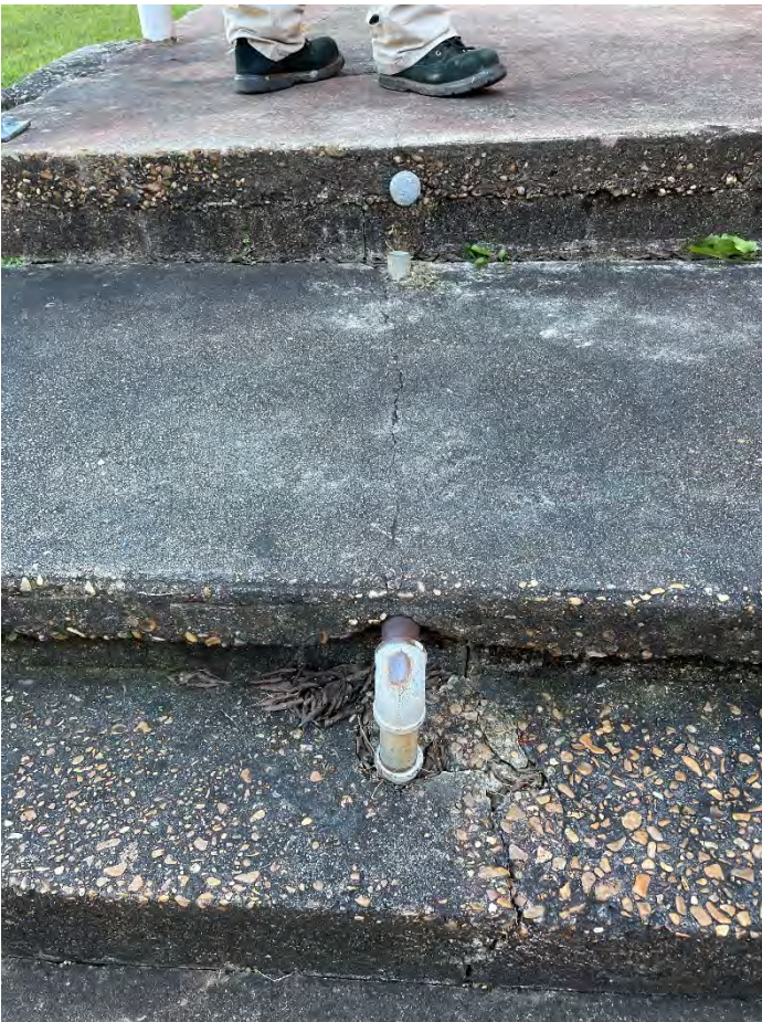
Steps On Grade Are Tripping Hazard & Not ADA
