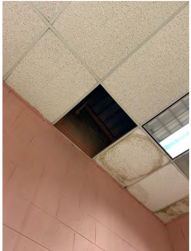
Water intrusion at Gable end walls
