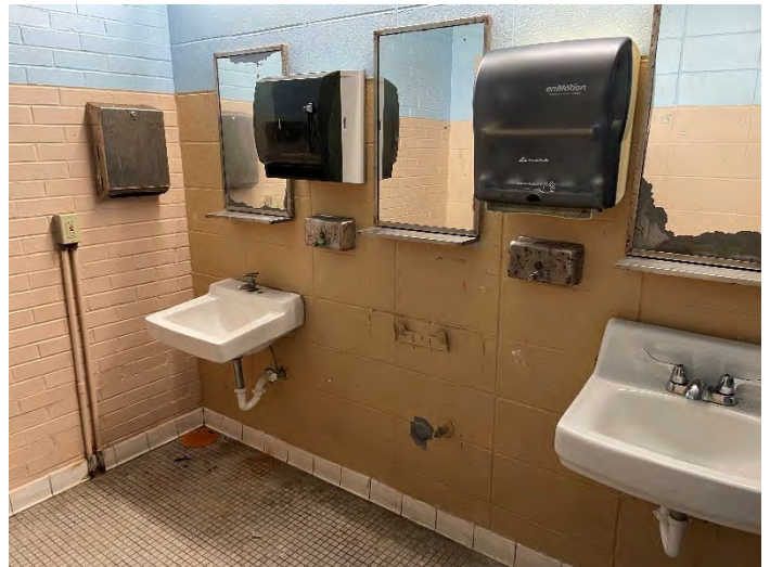
Sinks Do Not Meet ADA – Rusted Accessories & Dispensers Above 48"
