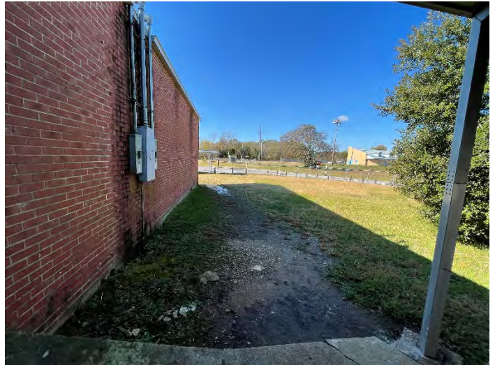
Example of Standing Water On Grade Close To The Structure
