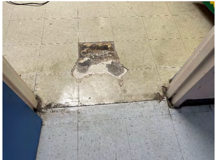
Example of Damaged Flooring – Trip Hazard
