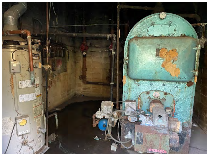
Mechanical Room Is Open & Holding Water
