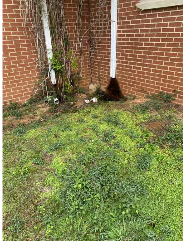
Gutters and Splash Guards Missing
