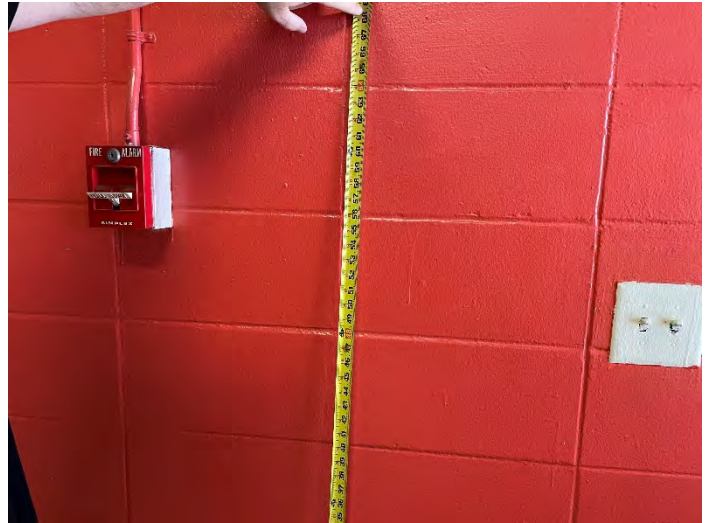
Example of Pull Stations, Light Switches & Fire Extinguishers Above 48"
