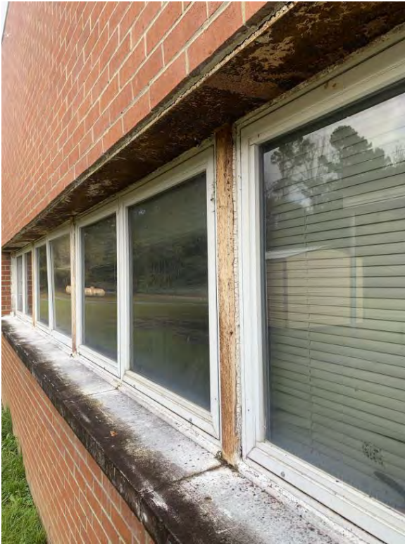
Deterioration of Steel At Exterior Window
