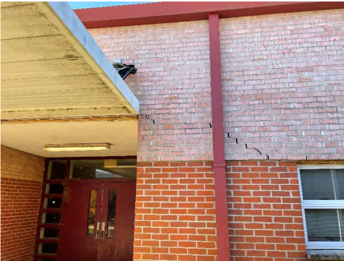
Masonry Separation. Possibly Due To Absence of Control Joints
