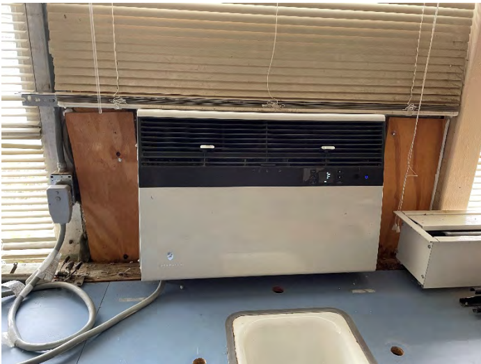
Most All Air Conditioning Comes From Window Units Units Secured With Plywood
