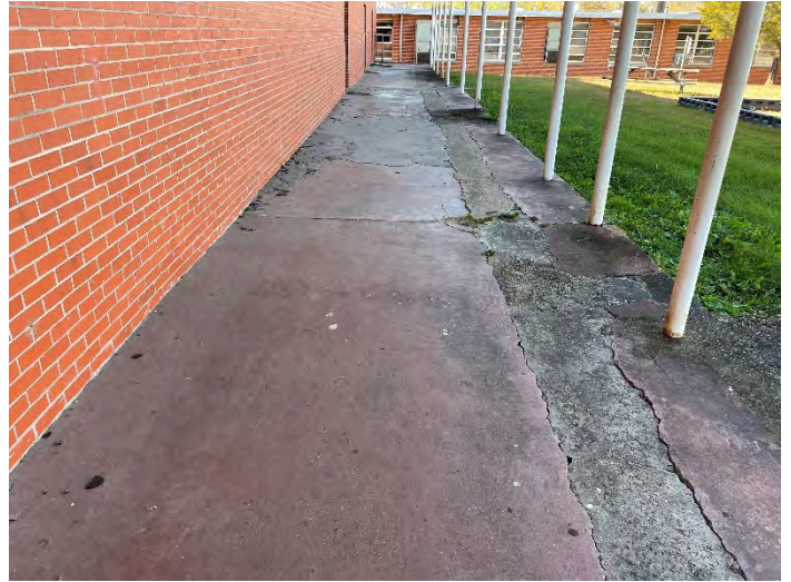
Walkways Are Damaged & Do Not Meet ADA
