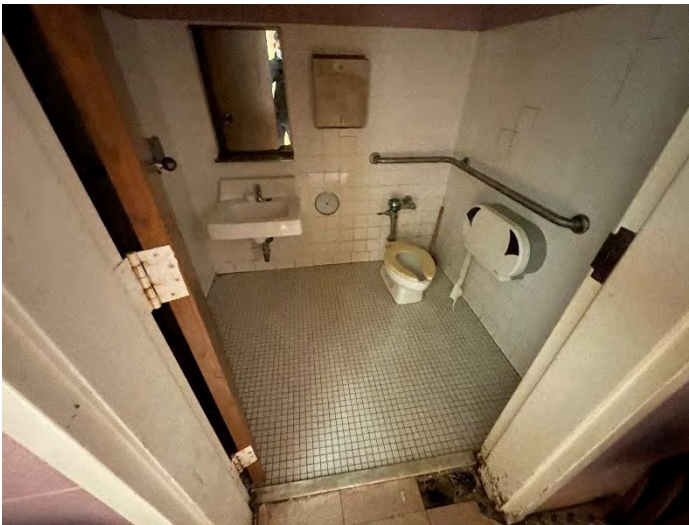
Example of Hard Tile In "Fair" Condition if Cleaned Note Rusty Door Frame & Hinges
