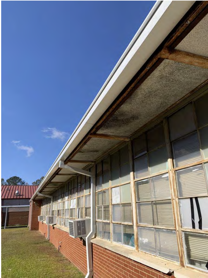
Rusting of exterior Window Jambs, Roof beams and deterioration to Roof decking
