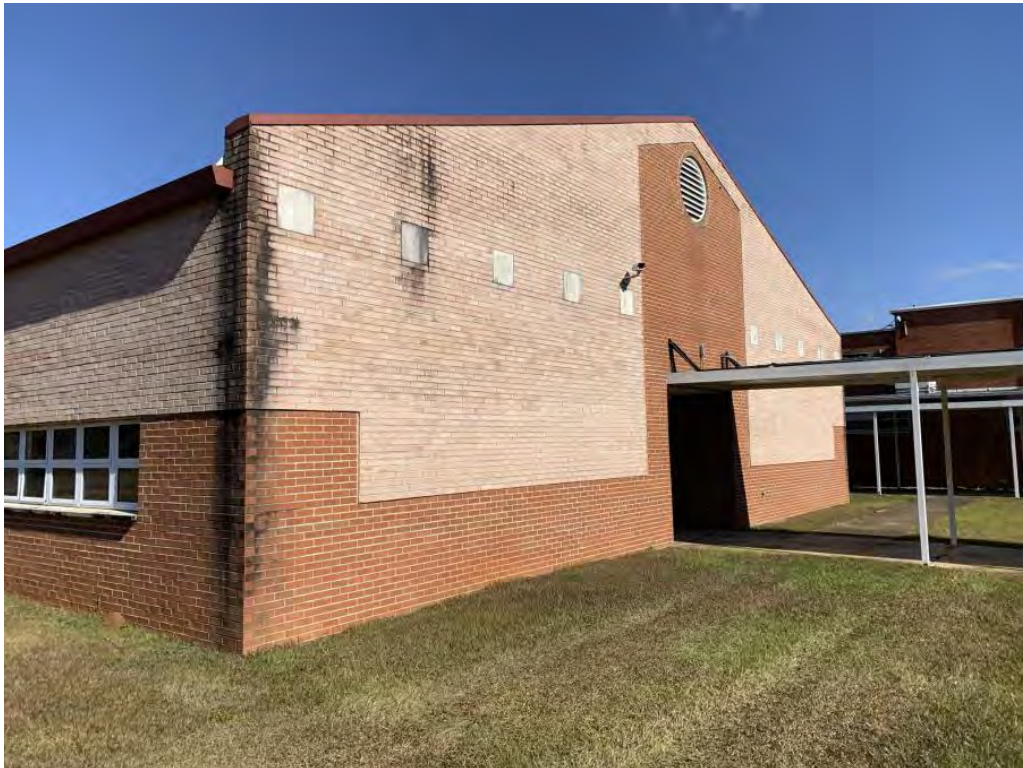
Missing or Damaged Gutters and Splash Guards
