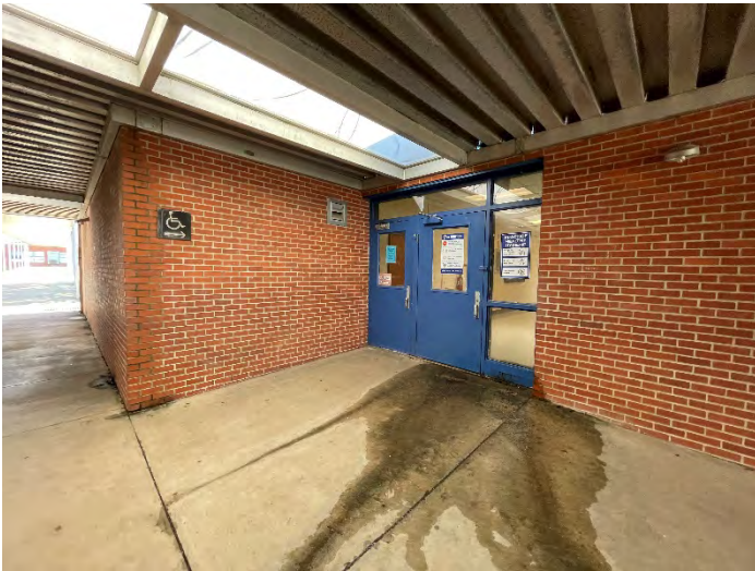
Canopy Leak Close to Egress Door
