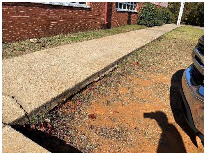
Example of Damaged Sidewalk – Trip Hazard
