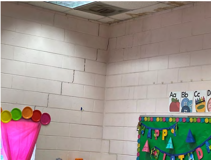
Observed Crack in CMU & Evidence of Roof Leaks
