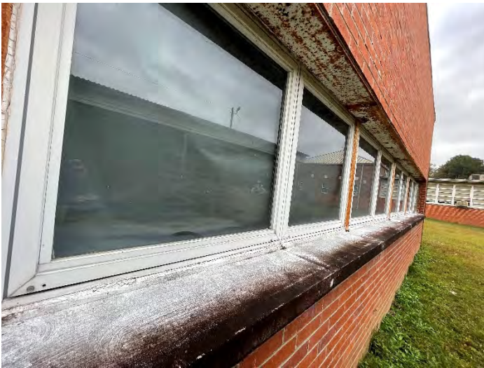
Steel Brick Lintels Are Rusty & Need To Be Repainted
