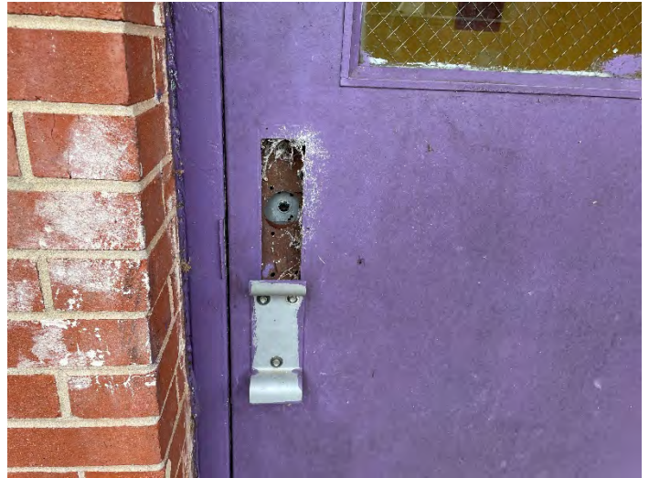
Insufficient Door Hardware At Side Egress
