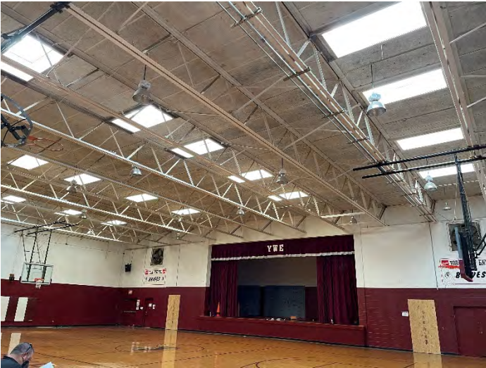
Skylights In Gym Are Aging & May Begin To Leak
