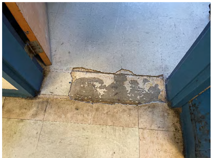
Example of Deteriorated / Damaged Floor at Doorway Causing Trip Hazard
