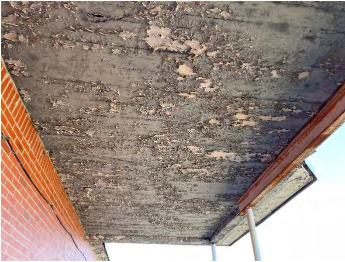
Paint Is Peeling on Concrete Canopy
