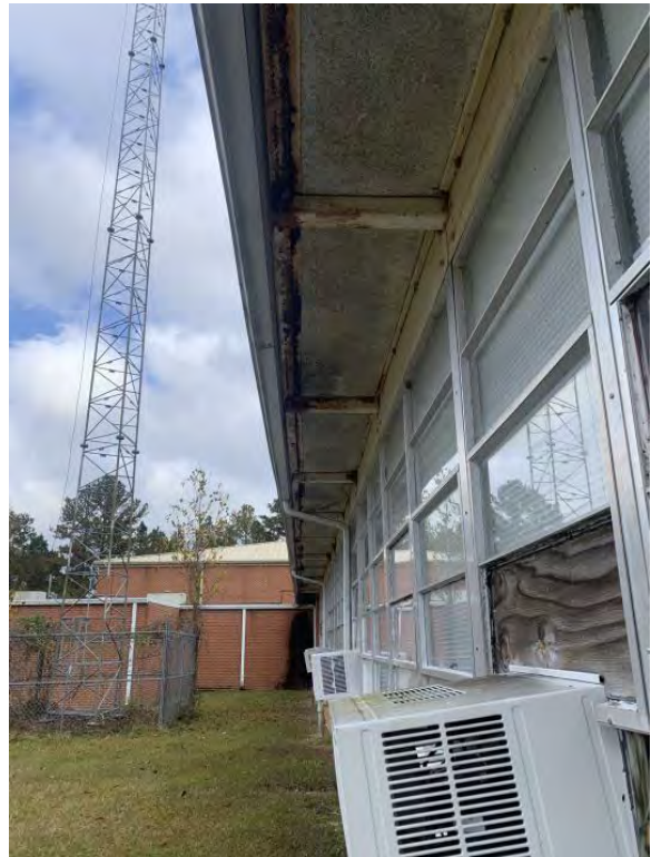
Deterioration of Exterior Eave Steel
