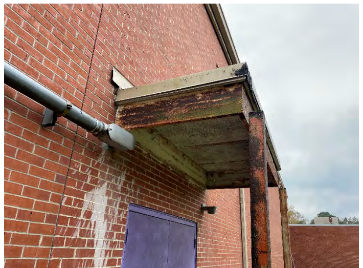
Small Canopy On Back Is Unsupported & Is A Safety Hazard
