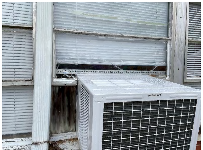
Aluminum Windows Are In Disrepair - Recommend Replacement
