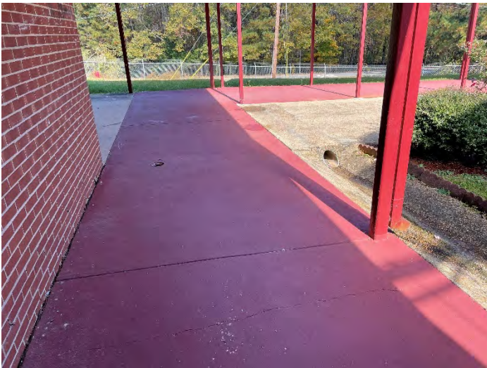
Coated Concrete Walks Appears to Be In "Fair" Condition
