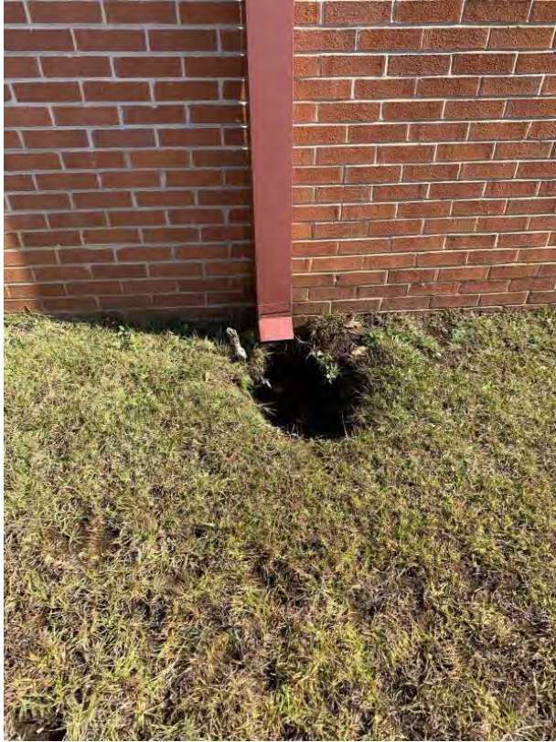
Missing or Damaged Gutters and Splash Guards
