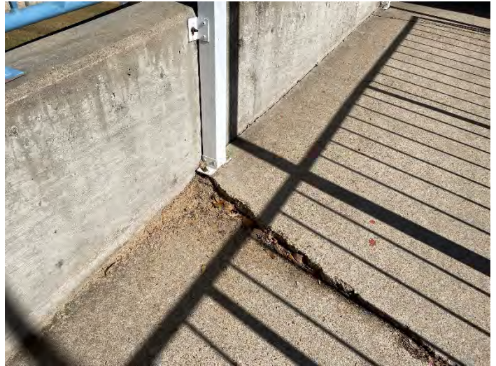
Concrete Failure at Canopy Support – Trip Hazard
