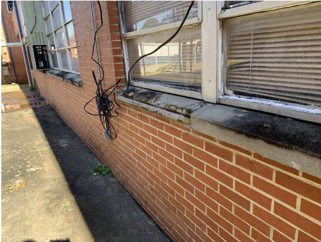
Deterioration of Precast Window Sills
