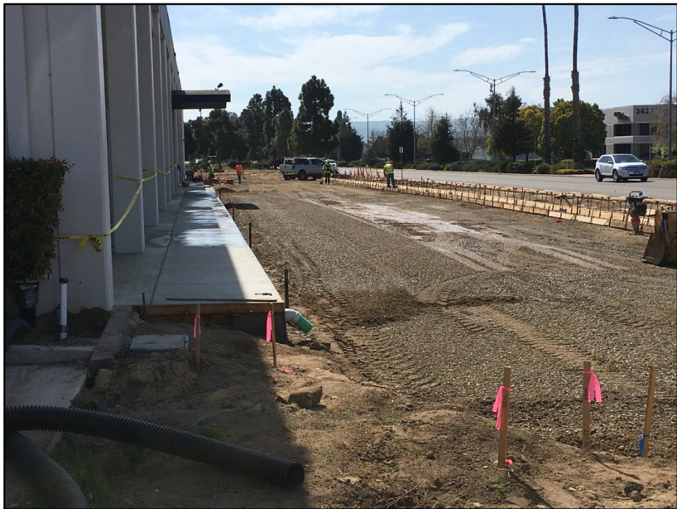
SSC West Parking – Main Parking Area at Finish Grade with Road Base in Place
