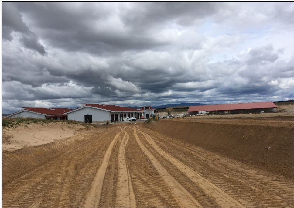
CTE Ag Center – Rough Graded Road View of the Campus
