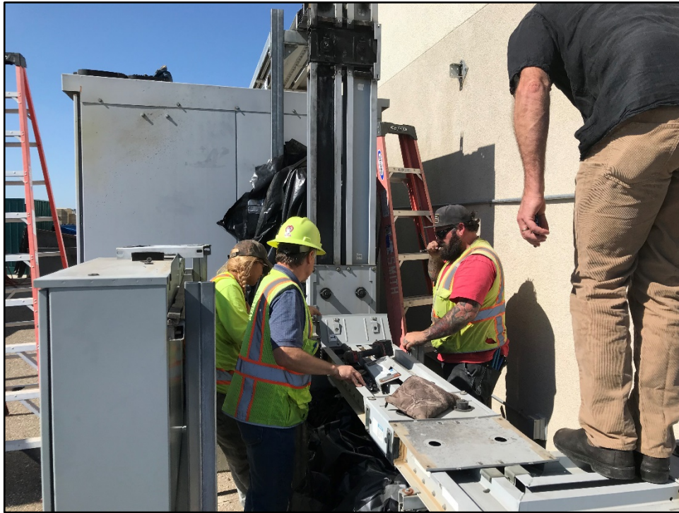
PVHS – Electricians Disassemble the Damaged Electrical Power Distribution Buss Duct
