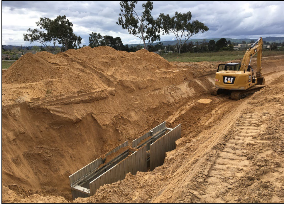
CTE Ag Center – Utilities Installation Under the New Road is Underway
