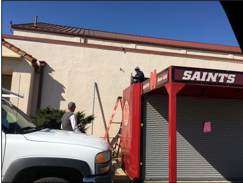
SMHS – Electricians Supply Power to the Quick Café Satellite Food Serving Station
