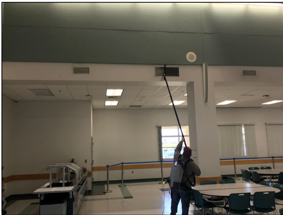
PVHS – Paul Alvarez Cleans HVAC Ducts in the Cafeteria
