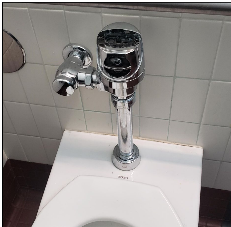
SMHS – Vandalized Toilet Flush Valve Required Replacement
