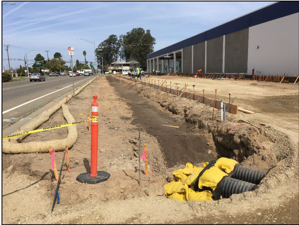
SSC West Parking – Bioswale and Concrete Curb in Progress
