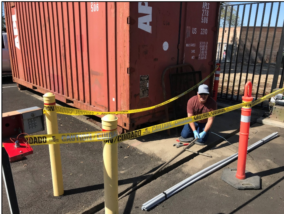
ERHS – Bernie Rayner Repairs the Gate Controls in the Student Parking Lot
