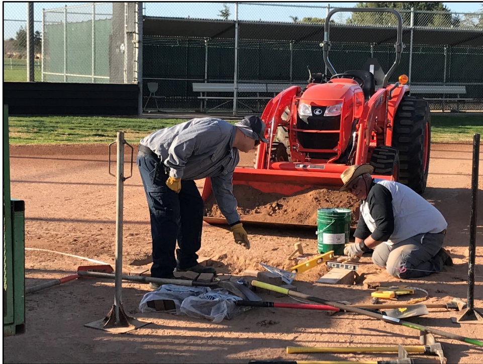
PVHS – Greg Gentile and Matt Schlereth Rebuild the Pitchers Circle at Varsity Softball
