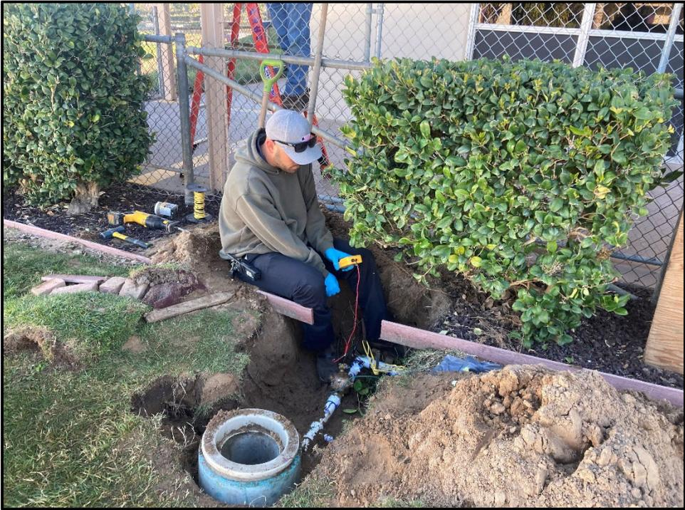
**ERHS – Jordan Markstone Repairing a Damaged Irrigation Wire**
