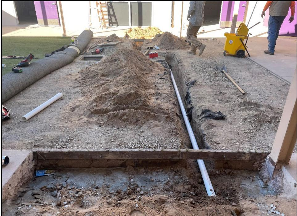
**ERHS Modernization – New Plumbing Goes in Under the Artificial Turf at the 200 Building**
