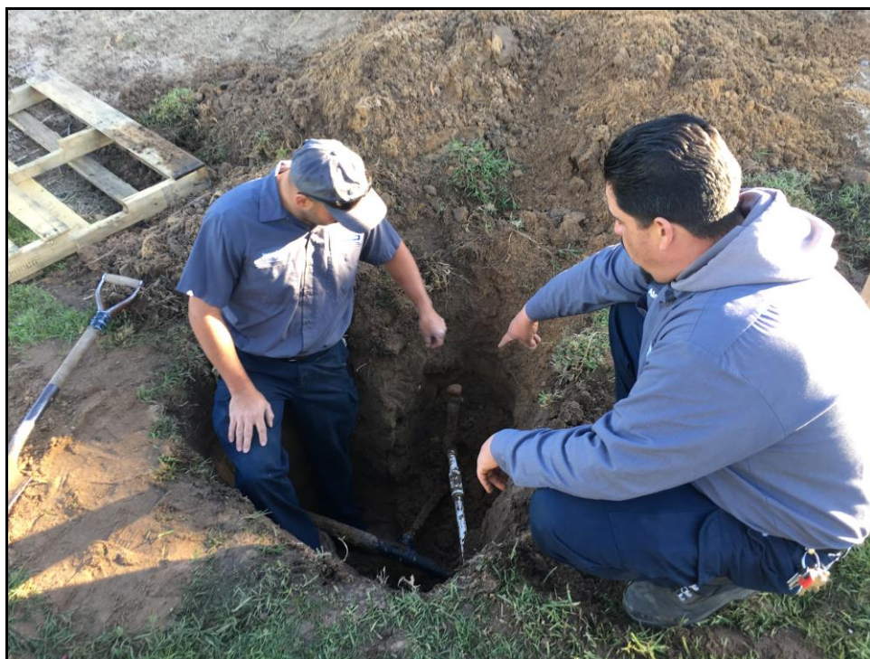
ERHS – Joseph Campos and Alan Rodriguez Repair Sprinkler Lines
