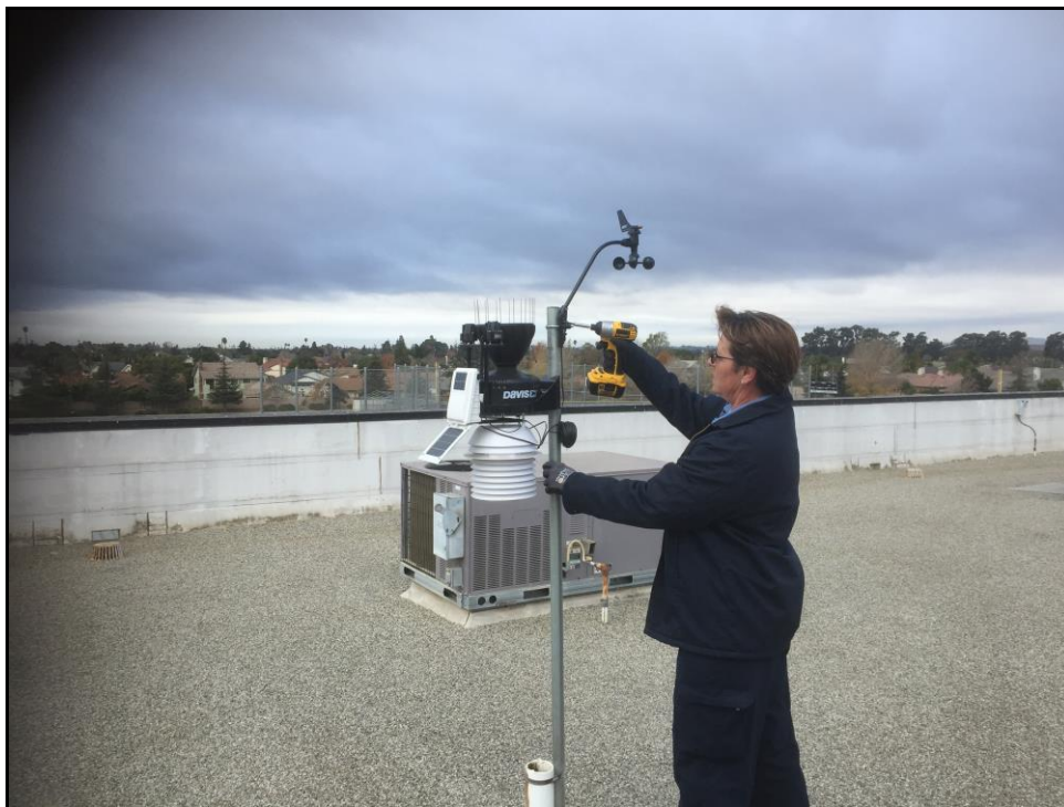
PVHS – Jennifer Abend Installs a New Weather Station for the Science Department
