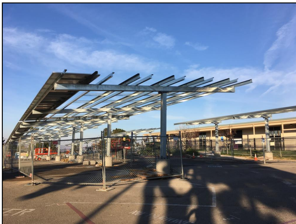
ERHS Solar Power – Steel Supports Installed in the Staff Parking Lot
