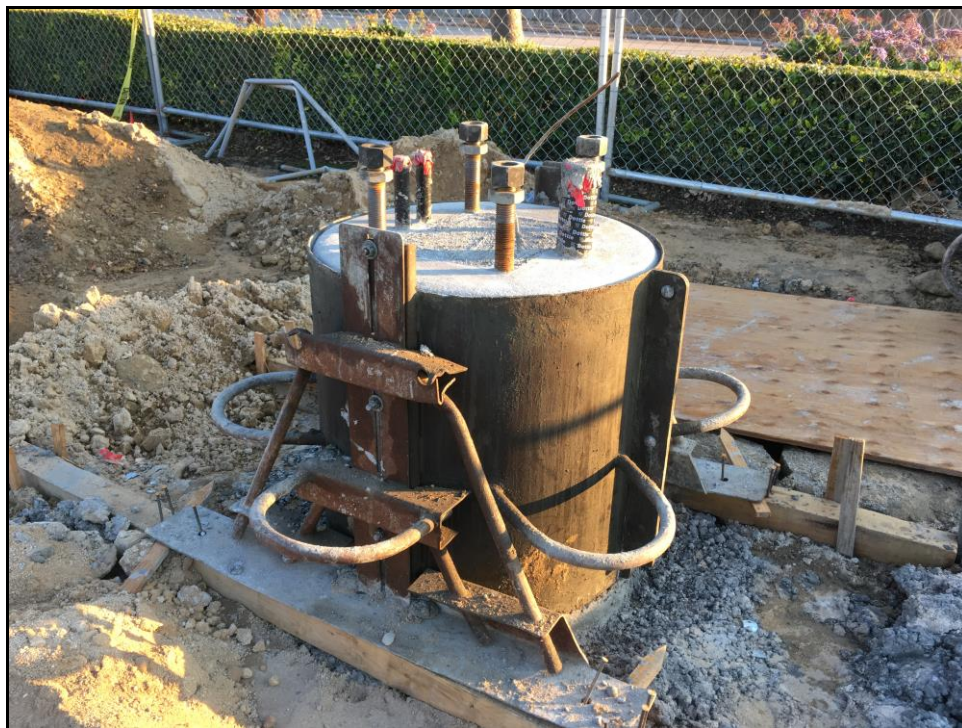
ERHS Solar Power – Final Concrete Piers in Place
