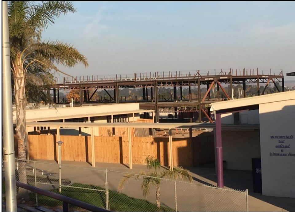
ERHS 38 Classroom Building – View of Third Floor from the Campus Quad
