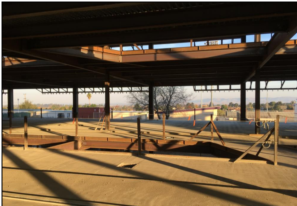
ERHS 38 Classroom Building – Second Floor Concrete Overlooking the Weight Room Roof
