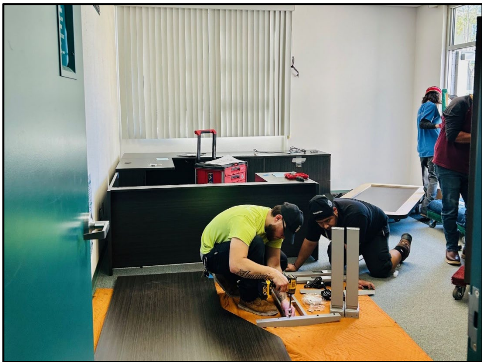
PVHS – New Office Furniture Installed in the Principal's Office
