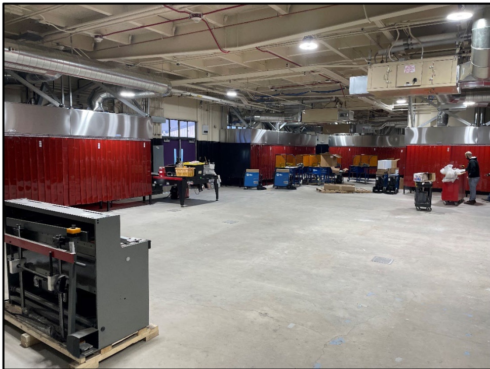
ERHS CTE Modernization – Welding Shop Plumbing Nears Completion
