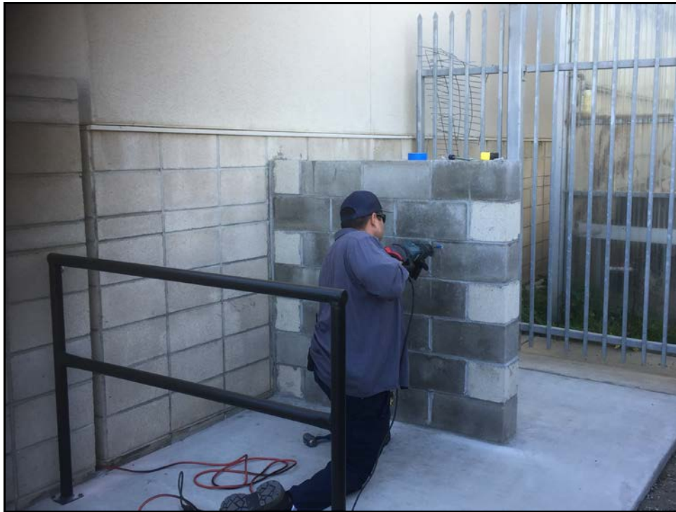
PVHS - Elias Camacho Prepares the Welding Gas Storage for Spare Tanks
