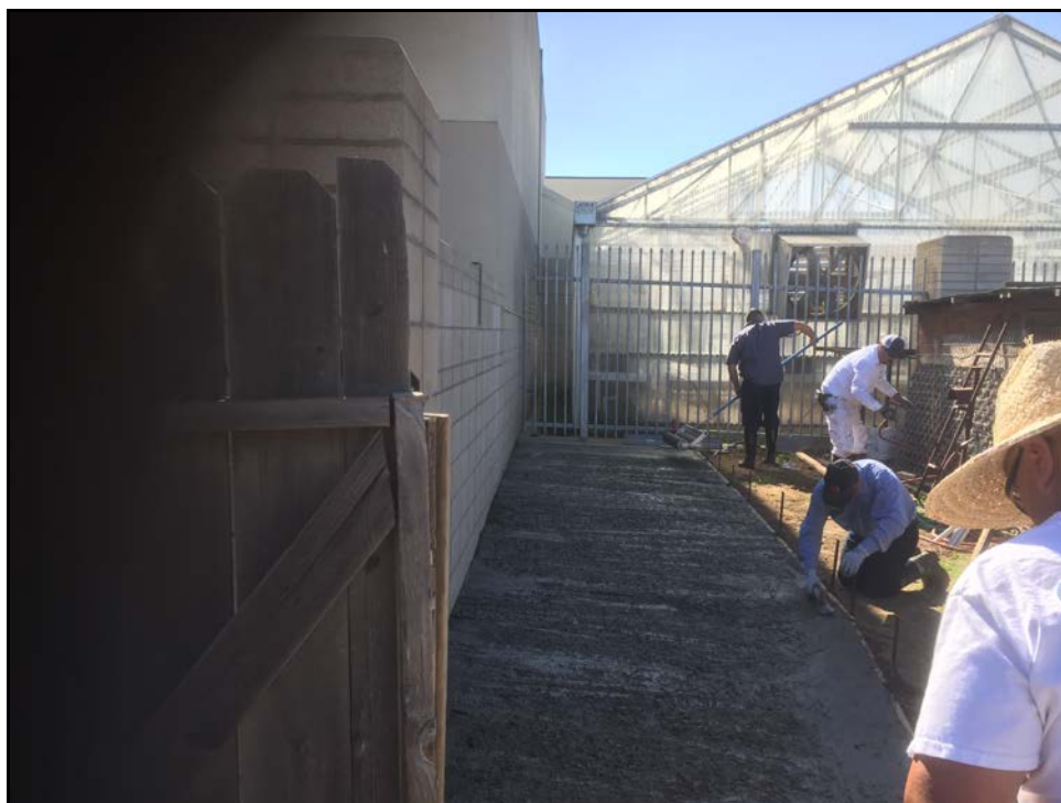
PVHS - Many Hands Pour Concrete for Welding Gas Storage
