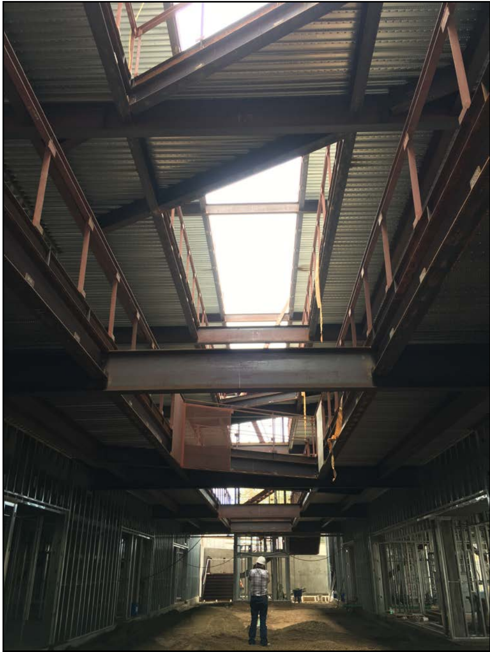
ERHS 38-Classroom Building – View from Ground Floor Shows Three Classroom Levels
