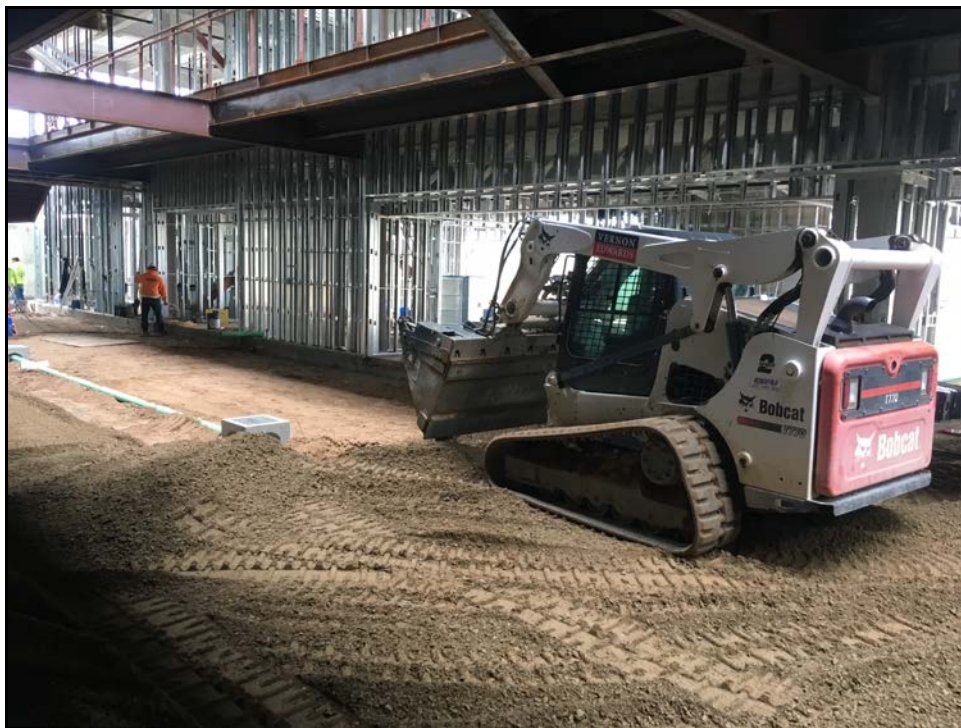
ERHS 38-Classroom Building – Preparing the First Floor for Concrete Walkway
