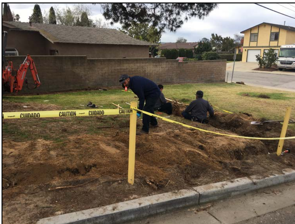
ERHS – The Grounds Crew Attacks an Irrigation Leak at the Berrywood Gate
