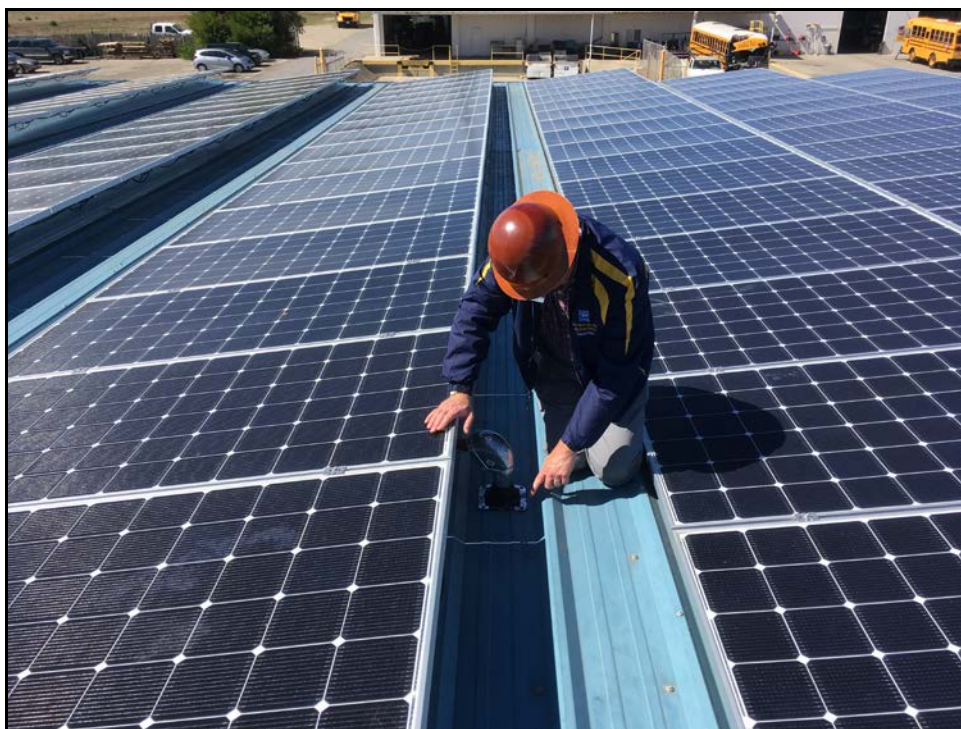
SSC Solar Power – District Inspector Reviews Bus Barn Roof Installation
