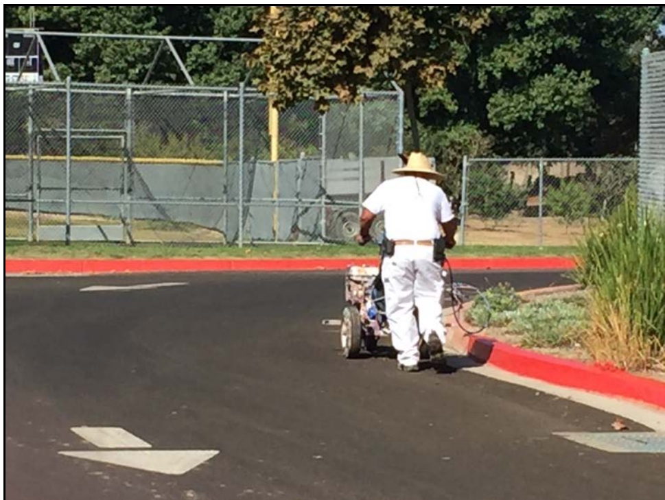
PVHS – Ray Segovia Repaints Campus Access Road Curbs
