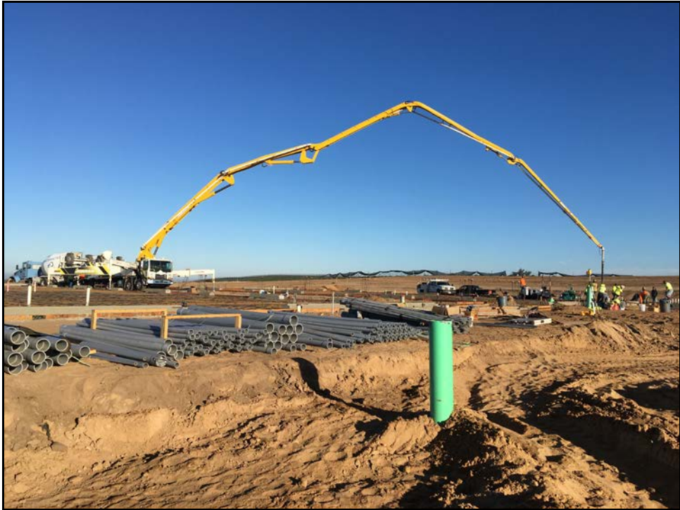
CTE Ag Center – Concrete Pouring Accomplished with a Pumping Unit
