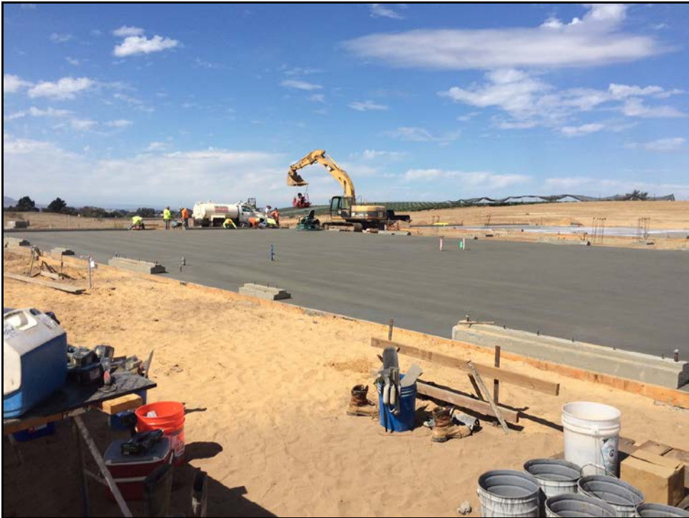
CTE Ag Center – Concrete Slabs are Finished for the Shop Buildings
