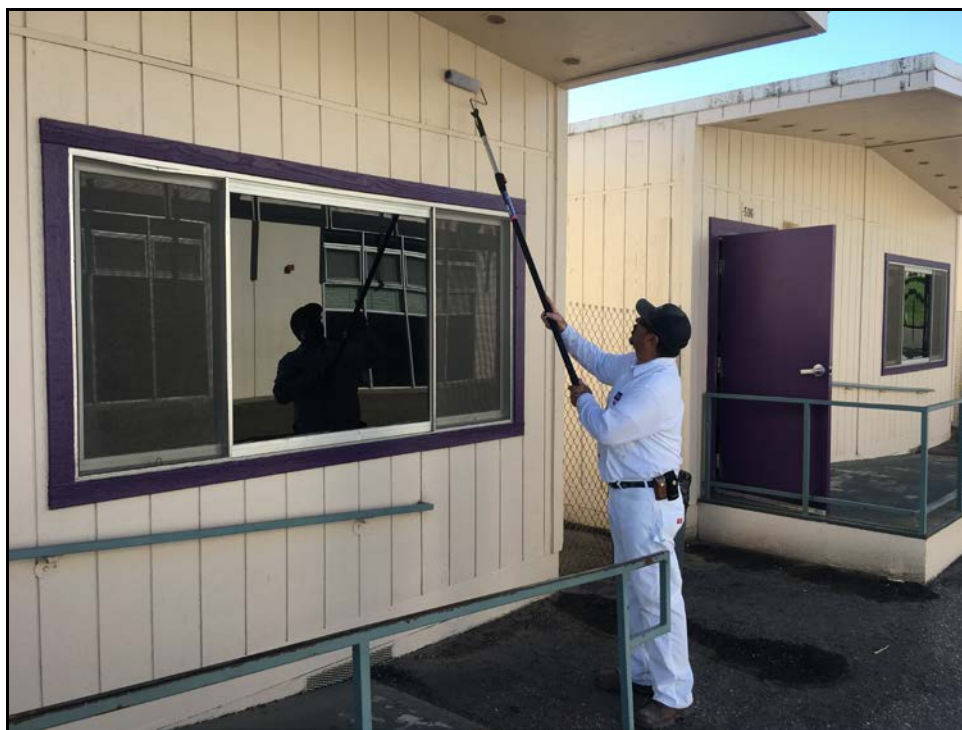
ERHS – Ernest Paz Paints Portable Classroom Exterior Walls
