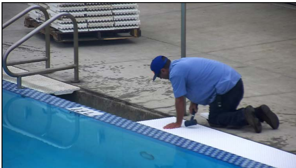
SMHS – Erik Fulton Installs Replacement Drainage Grates at the Pool
