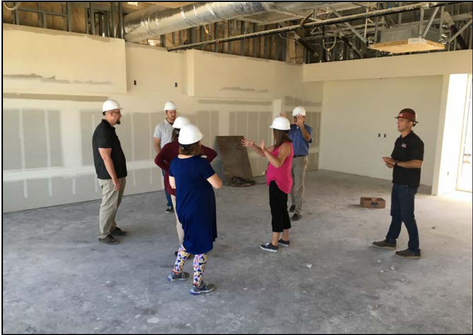
ERHS 38-Classroom Building – Teachers Tour the Classrooms Under Construction
