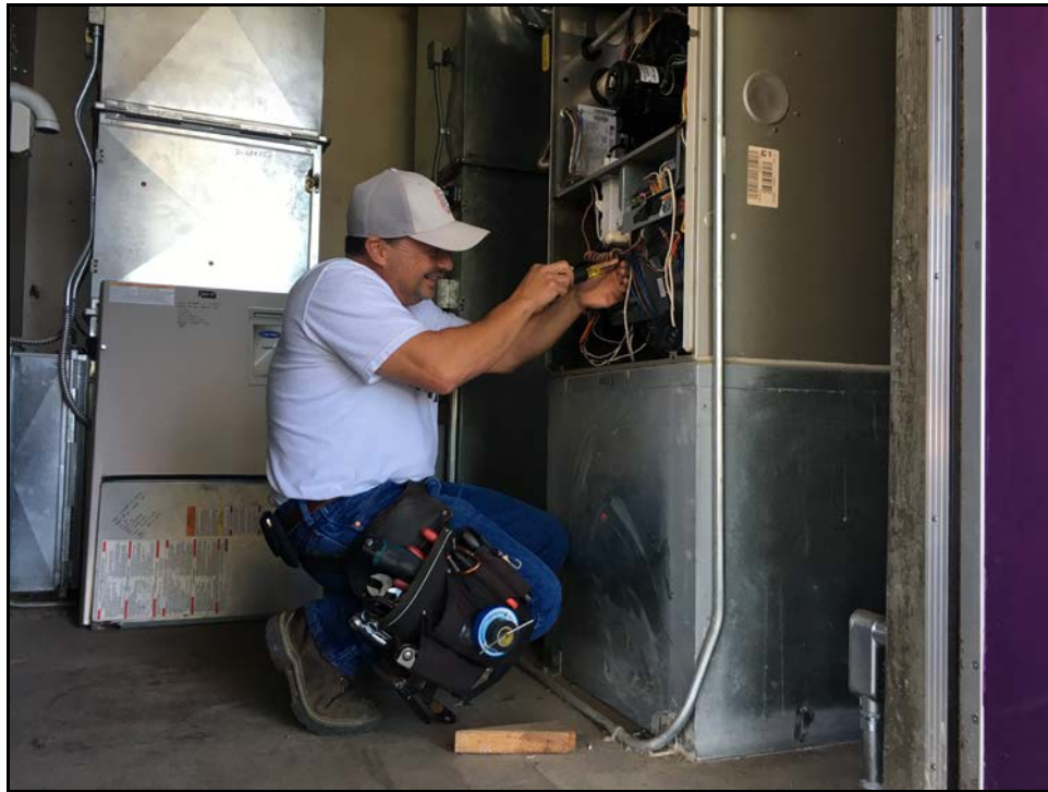
ERHS – Bernie Rayner Replaces the Fan Motor in the Administration Heater
