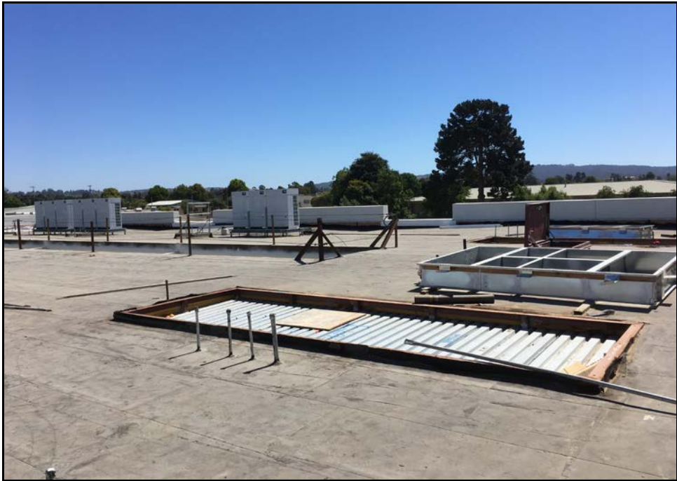
ERHS 38-Classroom Building – HVAC Units Are Placed on the Roof
