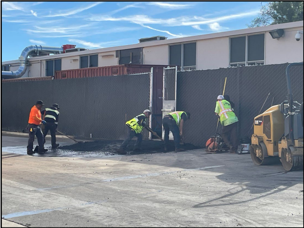
ERHS CTE Modernization – Installing an ADA Asphalt Path
