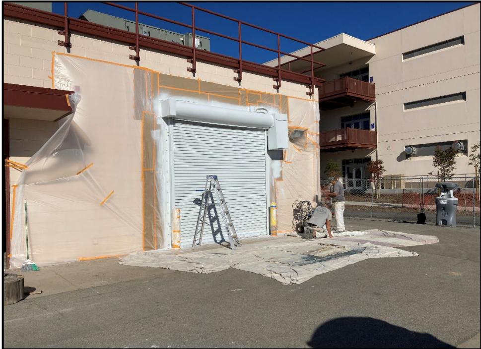
SMHS CTE Modernization – Painting Continues on all New Roll-up Doors
