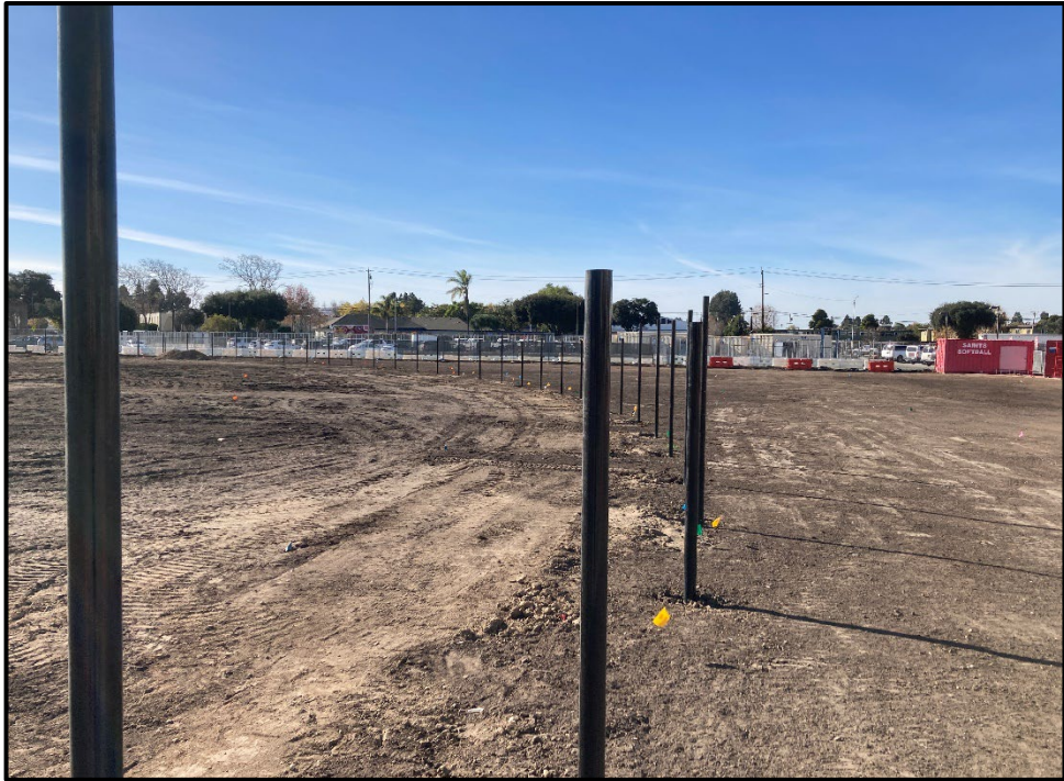
SMHS Reconstruction – Softball Outfield Fencing Posts are Being Installed
