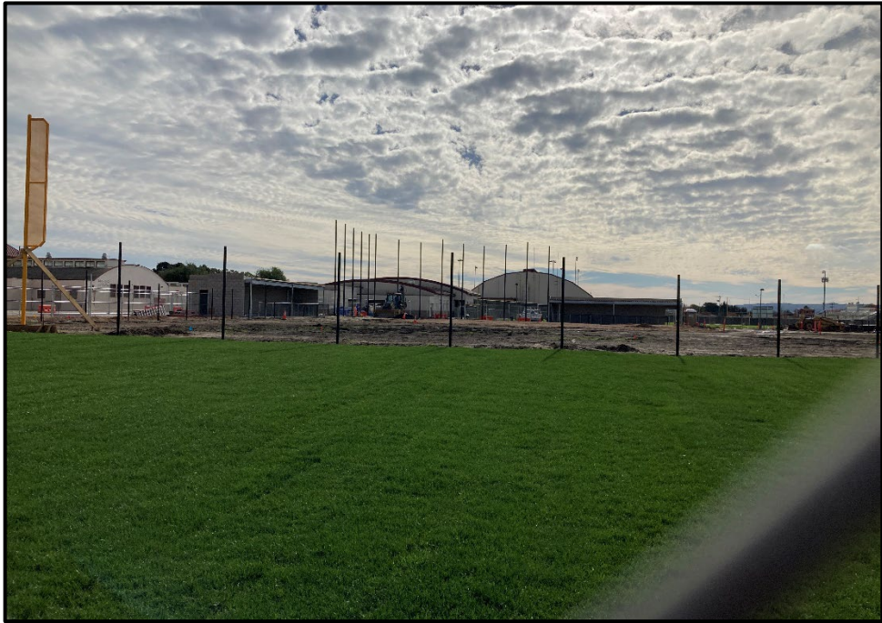
SMHS Reconstruction – Sod is Installed North of the Outfield Fencing
