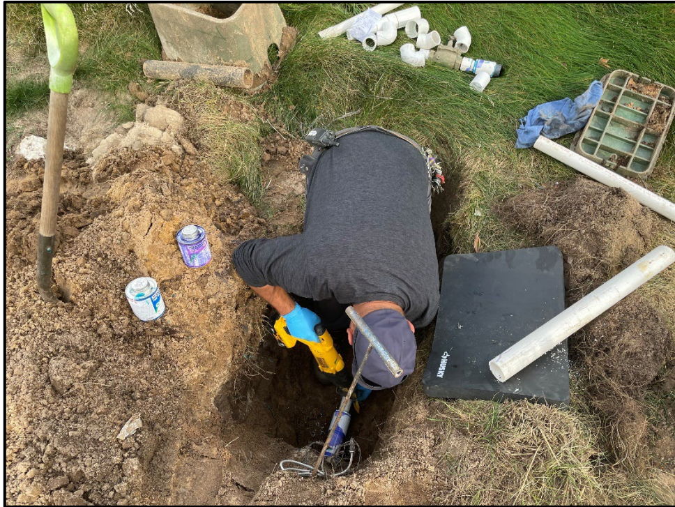
ERHS – Joseph Campos Repairing a Broken Water Line
