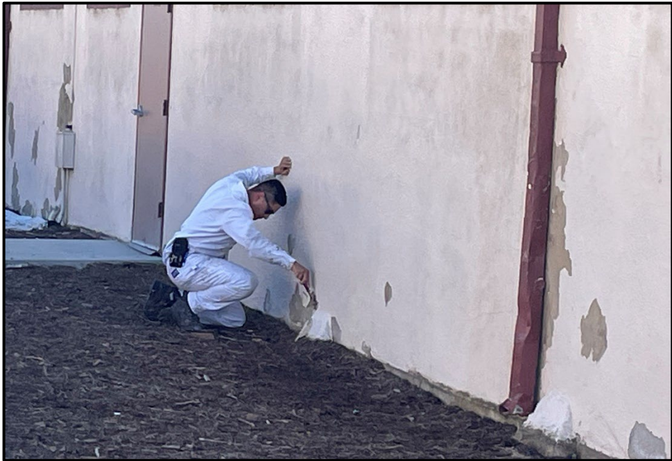
SMHS – Joel Amezcua Preparing to Paint the Exterior Wall of the 330 Agriculture Building
