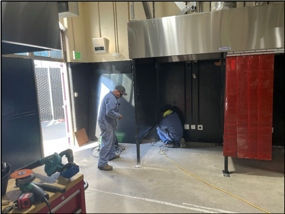
ERHS CTE Modernization – Welding Booth Installation is Underway
