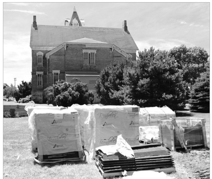
The shingles have arrived, and roofing work began July 1!
