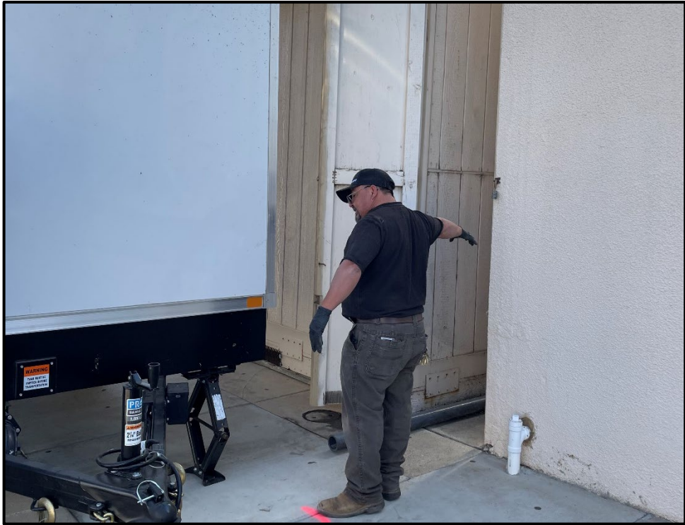
SMHS – Jesus Reyes Connecting the Plumbing for the New Portable Restroom Trailer
