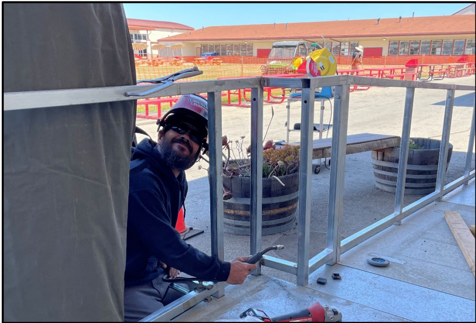
SMHS – Thomas Harbold Repairing a Portable Classroom Ramp Handrail
