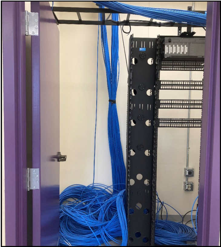
ERHS Modernization – Installed Upgraded Computer Cable
