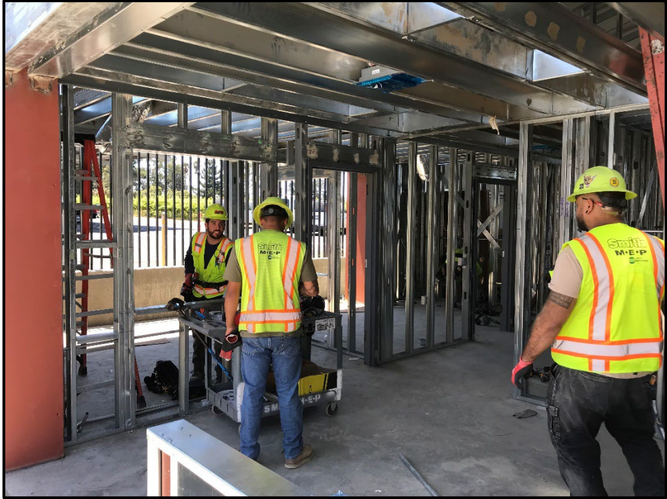
ERHS M&O Building – Interior Walls are Framed and Electrical Installation Begins
