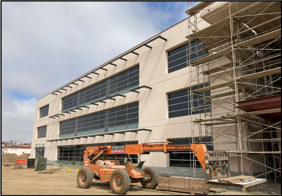
SMHS 50-Classroom Building – Campus Side Exterior Awaits Window Sun Screen
