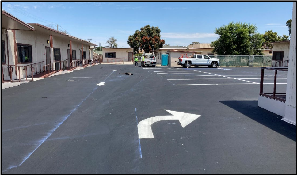
SMHS Lincoln Center – Paving, Striping, and Signage Work Has Been Completed
