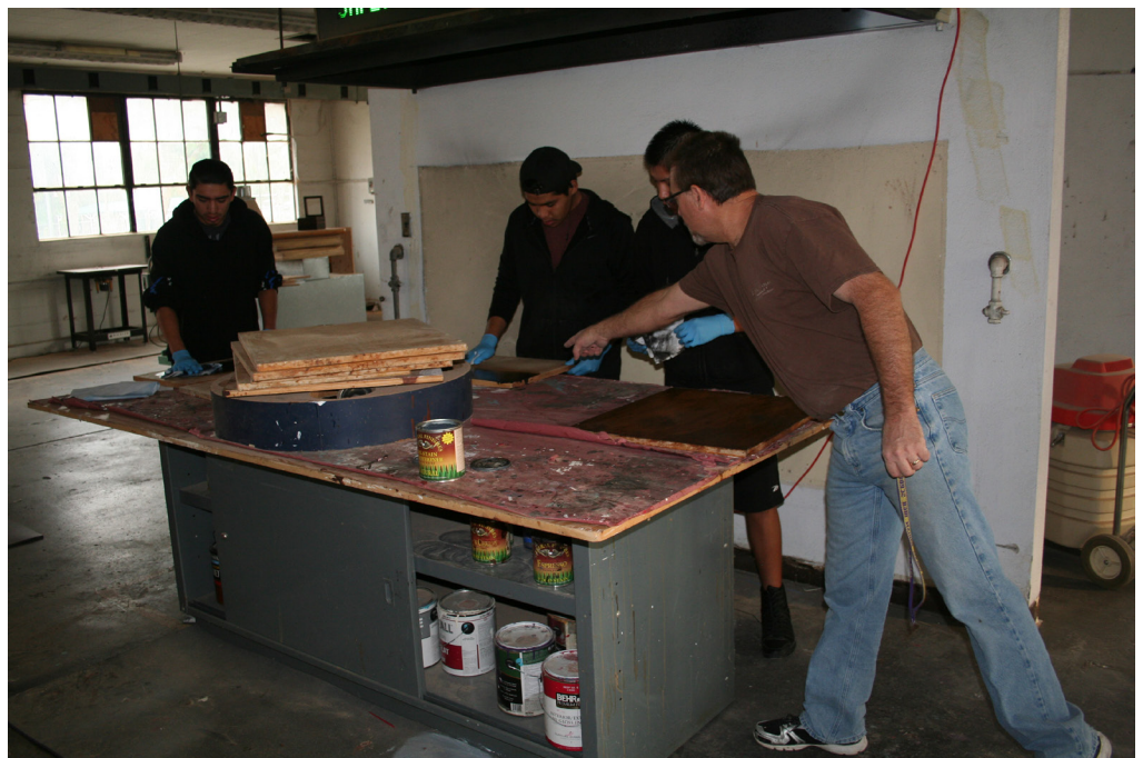
Figure 4. Students of Brian Hayden's (far right) construction 2 class staining cabinet doors.
