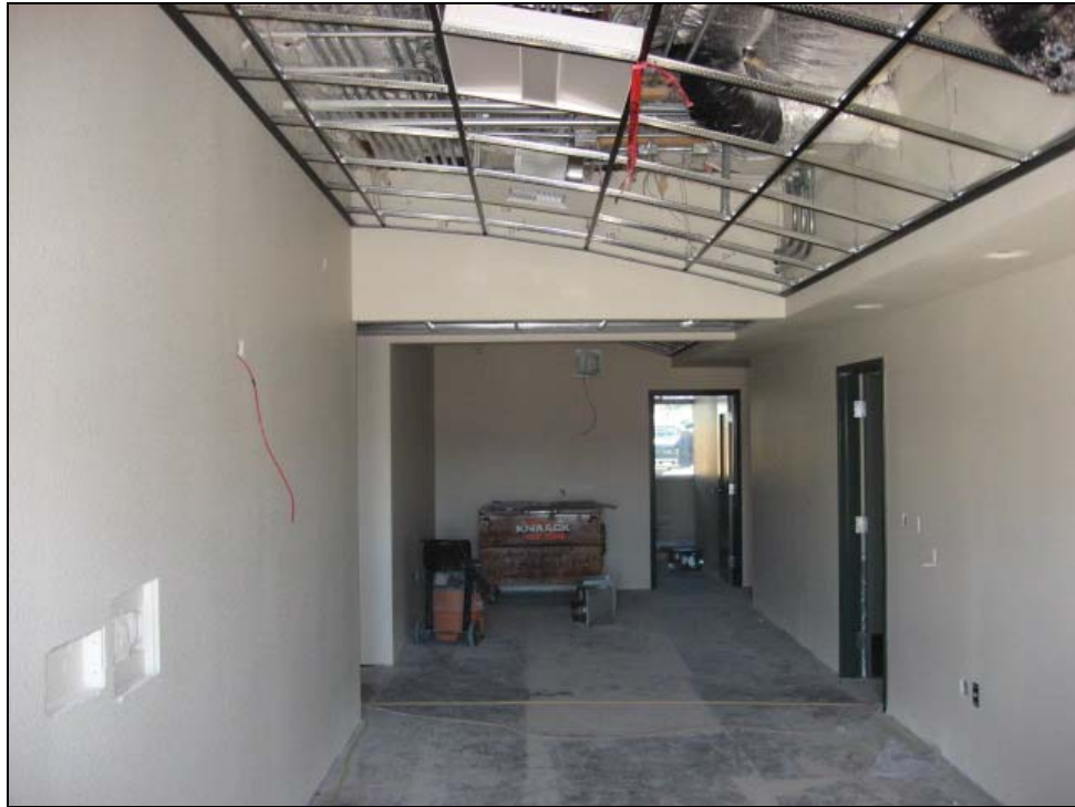
Righetti High Administration Architectural Arch Takes Shape
