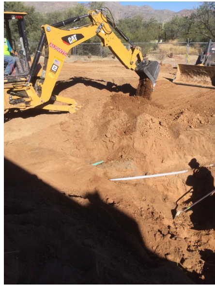
Agua Caliente Elementary School - Kindergarten Building site preparation continues.
