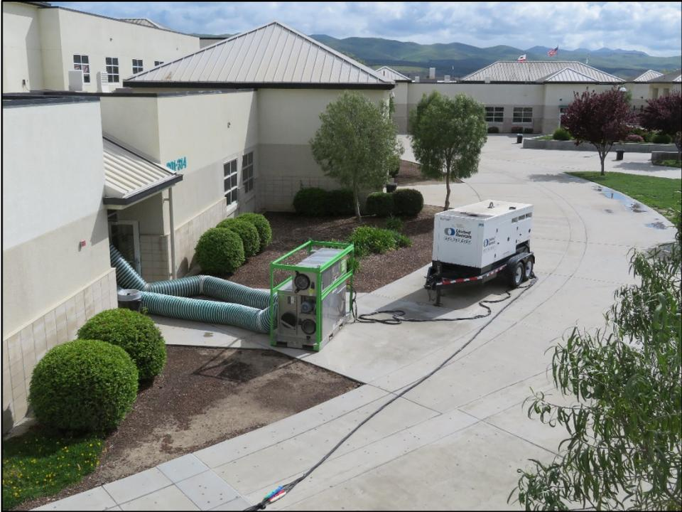
PVHS - Diesel Powered Desiccant Dryers Remove Moisture From the 300 Building
