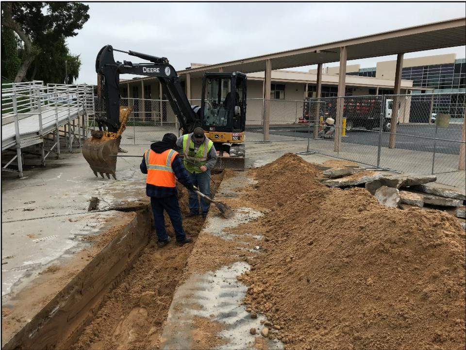
ERHS - Storm Drain Near the Greek Theater is Excavated to Clear a Blockage
