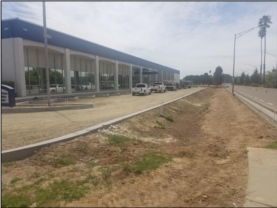
SSC West Parking - Curbs and Gutters in Place and Ready for Paving
