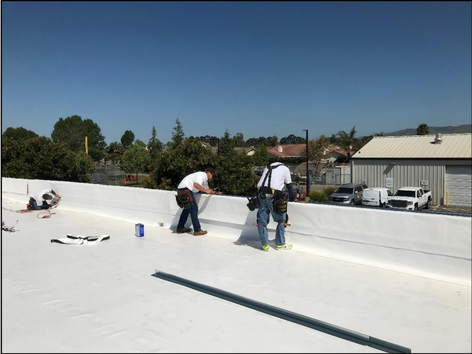
PVHS - Roofers Seal the Parapet Wall on a Modular Classroom Roof
