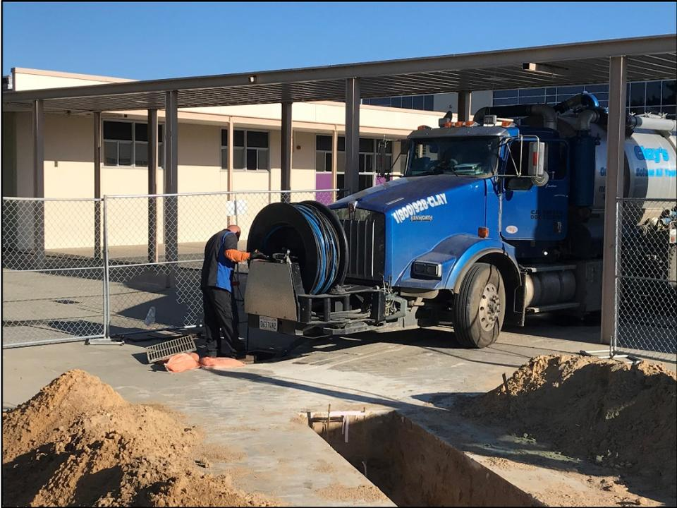
ERHS - Drain Hydro-Jet Used to Clear the Storm Drain
