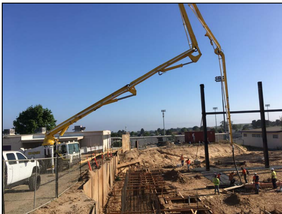
ERHS 38 Classroom Building – Concrete Footing Pour is Underway
