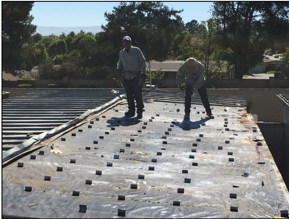
ERHS - Metal Roof Deck Comes off a Portable Roof
