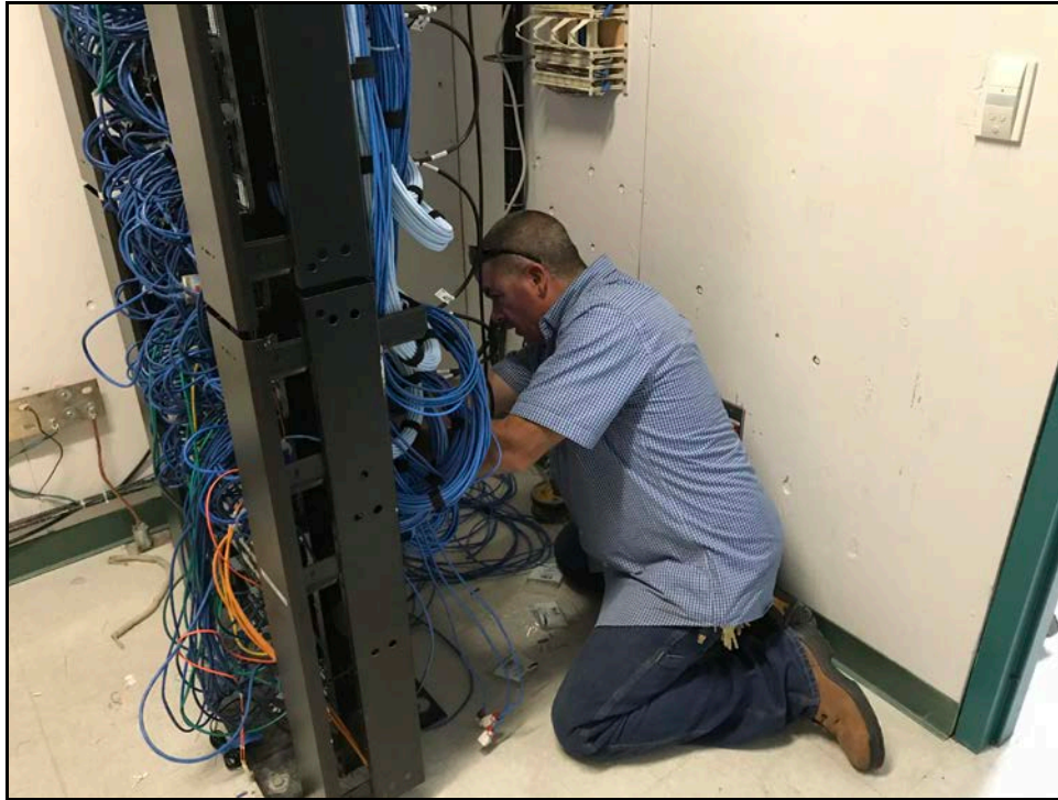
PVHS - New Electrician Andy Freitas Lands New Wire for VOIP Telephones
