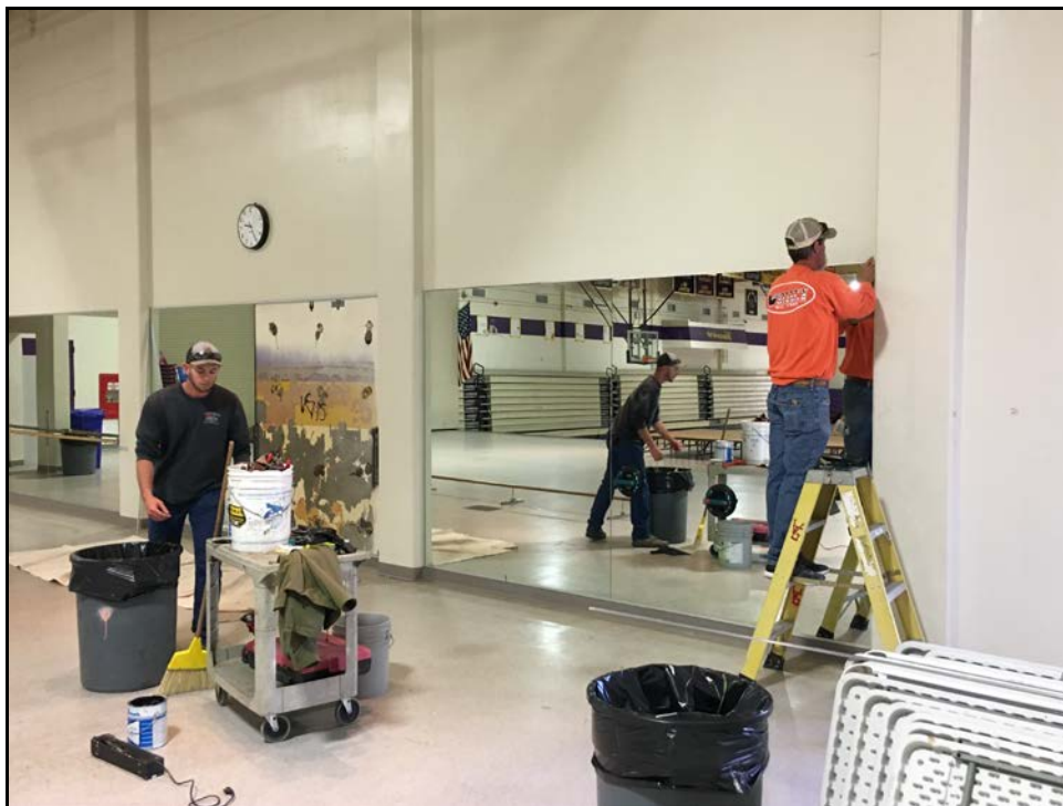
ERHS - New Mirrors Installed on the Gymnasium Stage
