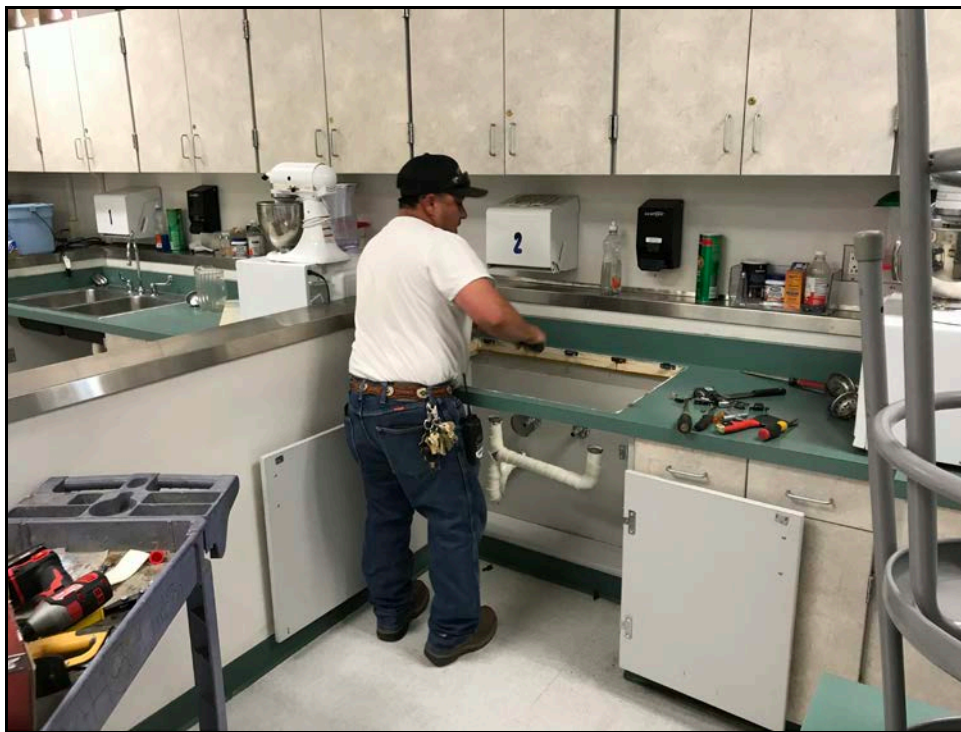
PVHS - New Plumber Jesus Reyes Installs Upgraded Sinks and Faucets in the Foods Lab
