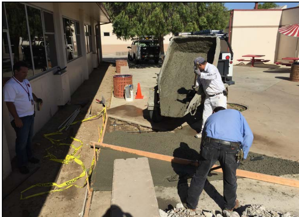
SMHS – José Placencia and Ernest Paz Repair Concrete After Math Building Water Leak
