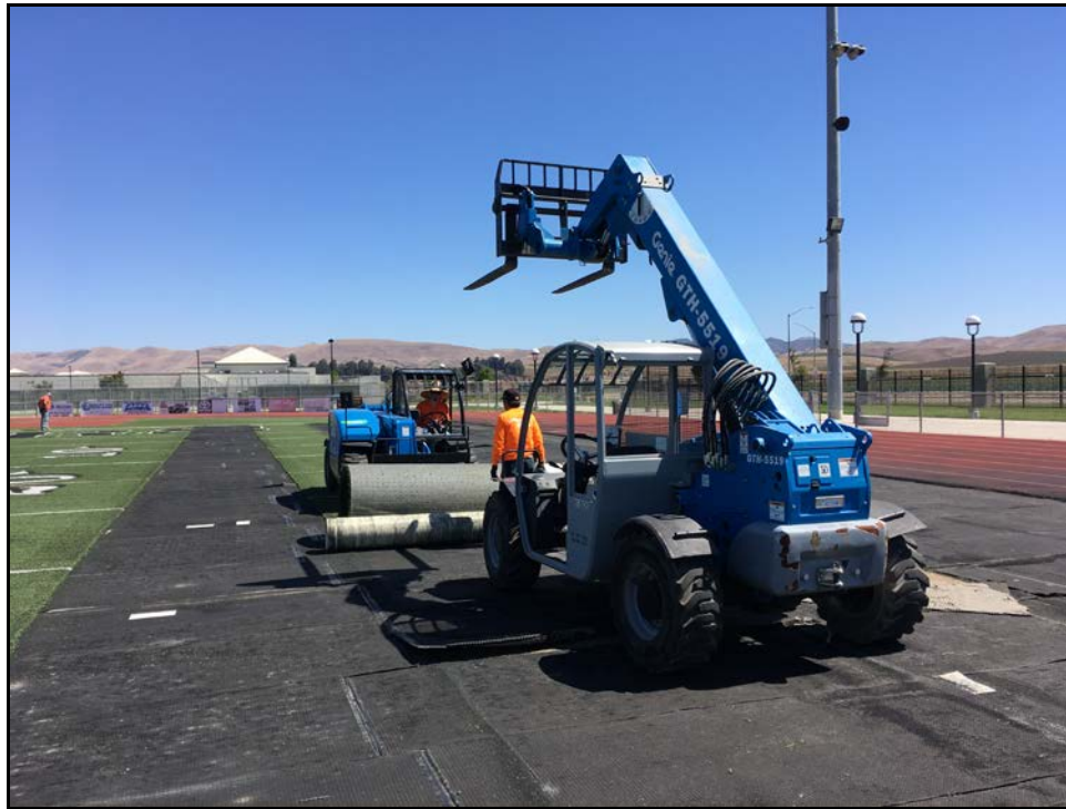
PVHS – The Original Turf is Cut and Removed in Large Rolls
