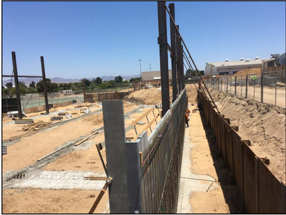
ERHS 38 Classroom Building – First Floor Concrete Wall is Poured
