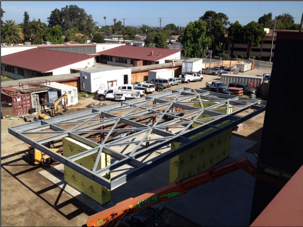
SMHS – Broadway Classroom Building Band Shelter Roof Framing
