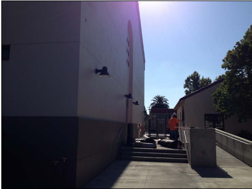
SMHS – Broadway Classroom Walkways and Ramps Taking Shape
