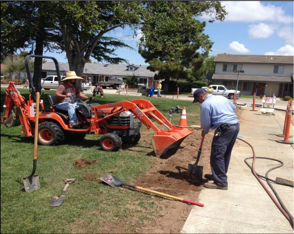
DHS – Juan Rodriguez and Ricardo Eliserio Grade after the County installed a New Sidewalk
