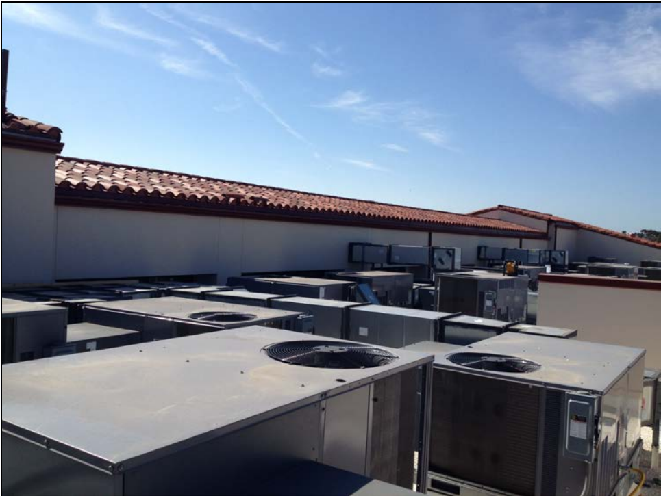
SMHS – Broadway Classroom Building Tile Roofs and HVAC Units
