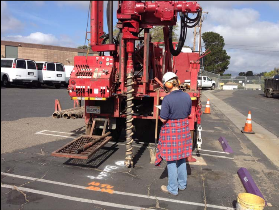
ERHS – Core Drilling in Preparation for the New 38-Classroom Building
