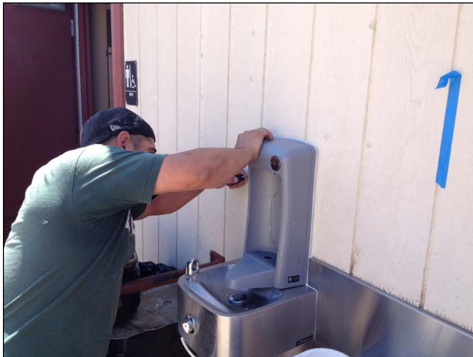
SMHS – Flavio Rodriguez Installs a Hydration Station near Softball and Portable Classrooms
