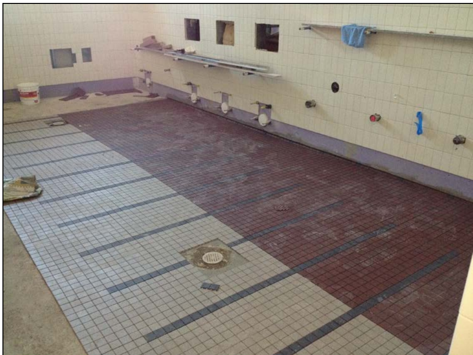
SMHS – Broadway Classroom Building Restroom Tile Installation in Progress
