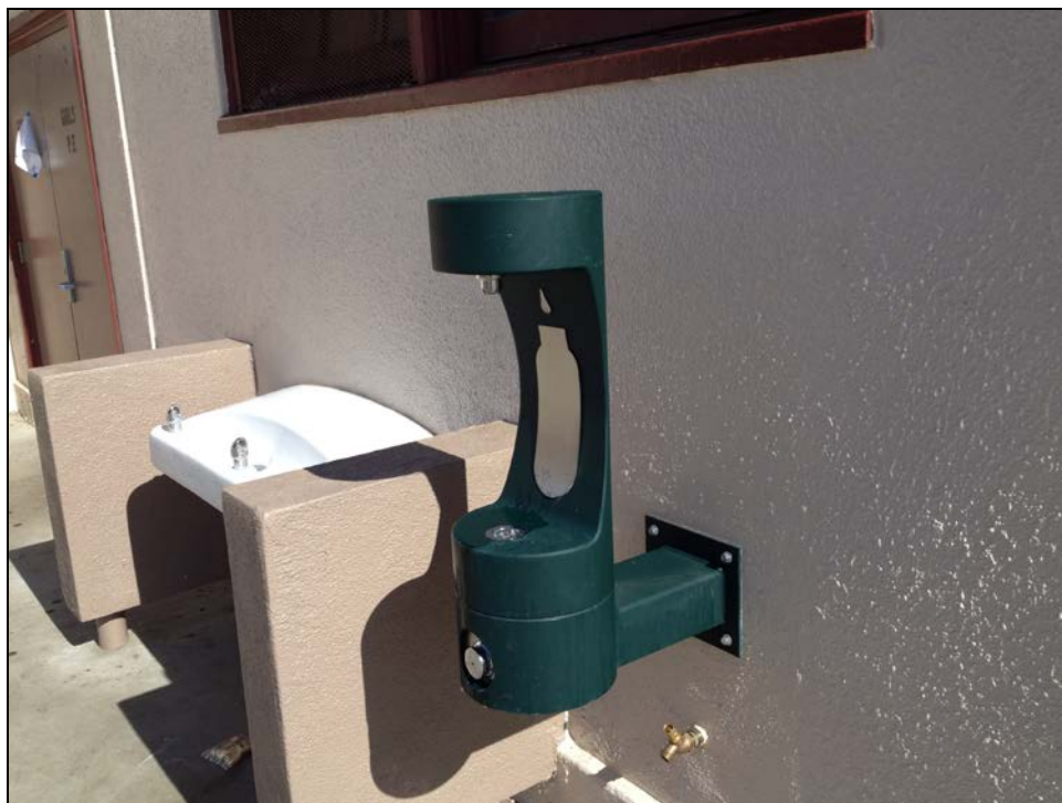
SMHS – The Small Gymnasium Hydration Station with Finished Stucco and Paint
