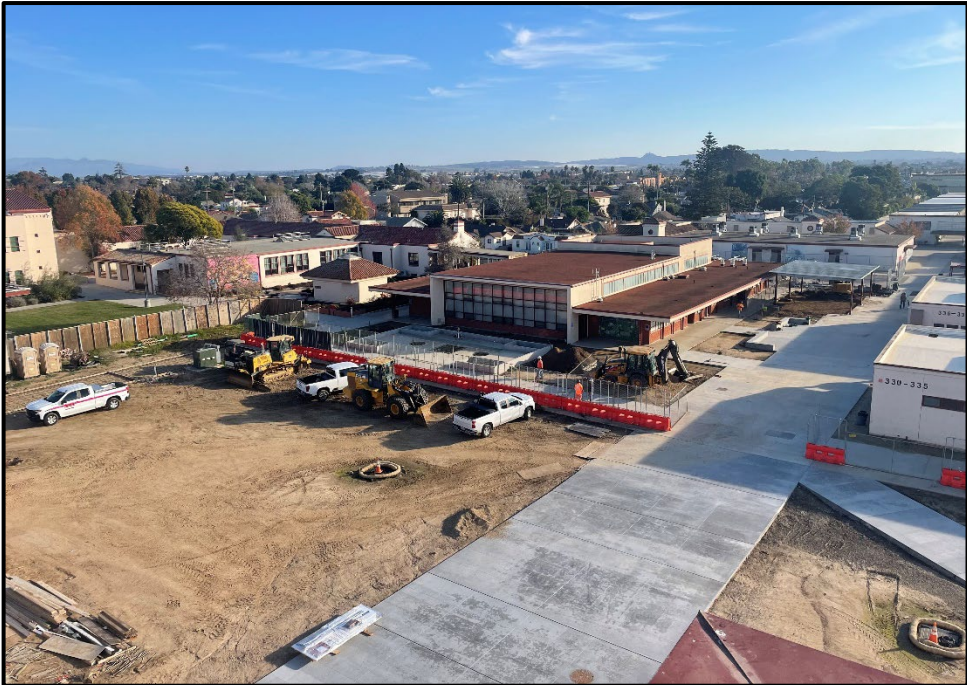
SMHS 50-Classroom Building – Installing Concrete Walkways Connecting the Campus
