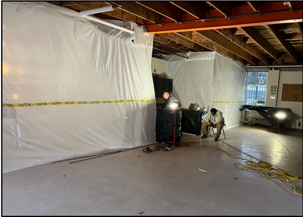
ERHS Modernization – Asbestos Abatement and Containment Continues Through Modernization Phases
