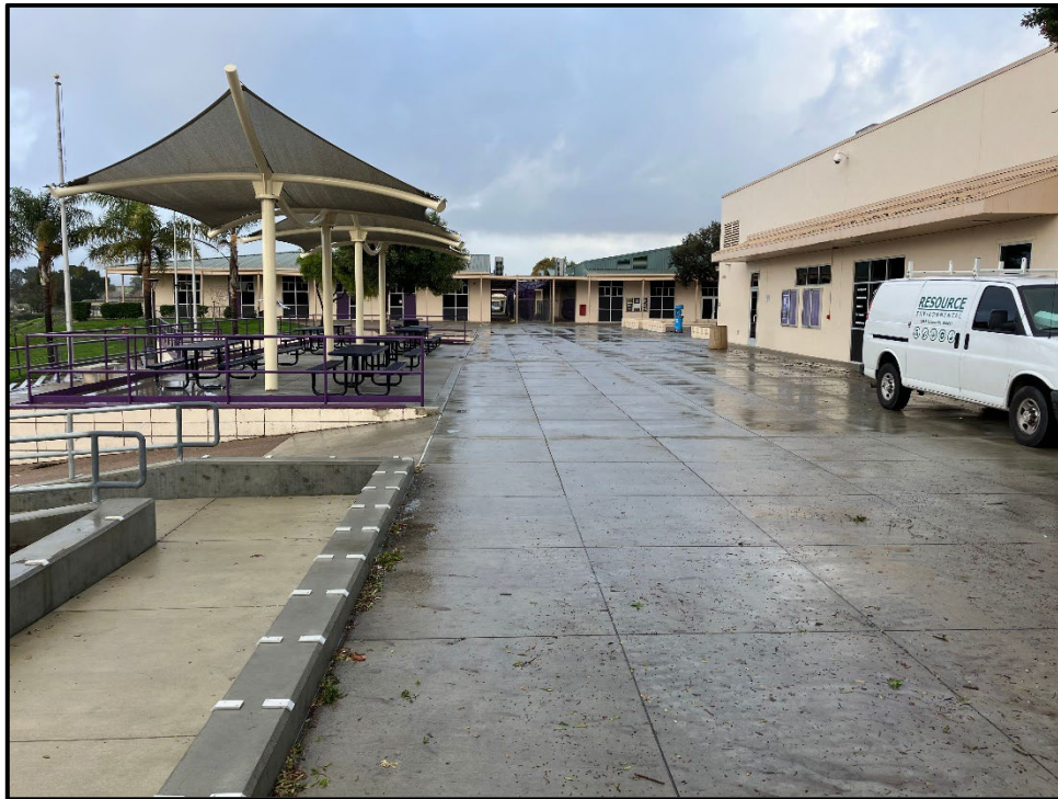
ERHS Shade Canopy - Lunch Tables Installed Under the New Quad Area Shade Canopy
