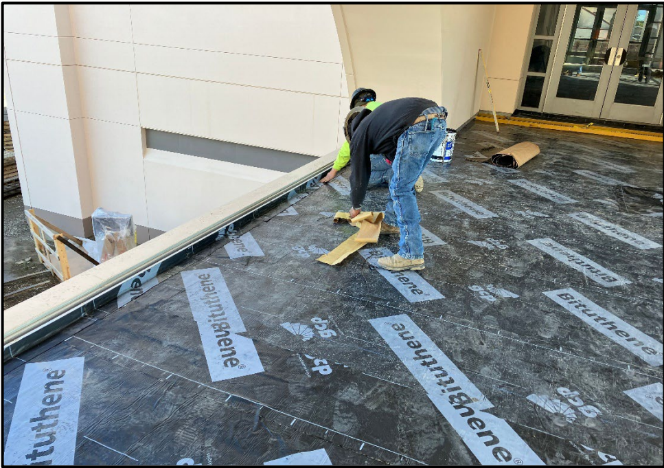
SMHS 50-Classroom Building – Waterproofing is Applied to the Second Story Walkway
