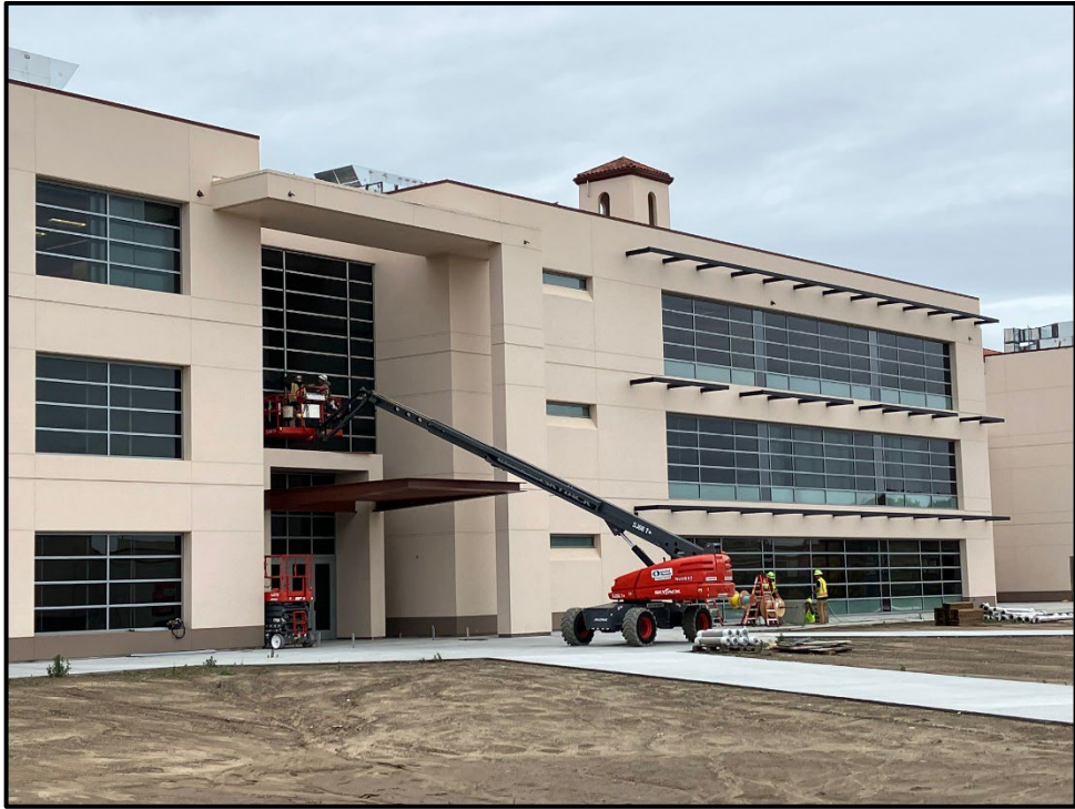
SMHS 50-Classroom Building – Finishing the Installation of Exterior Hallway Windows
