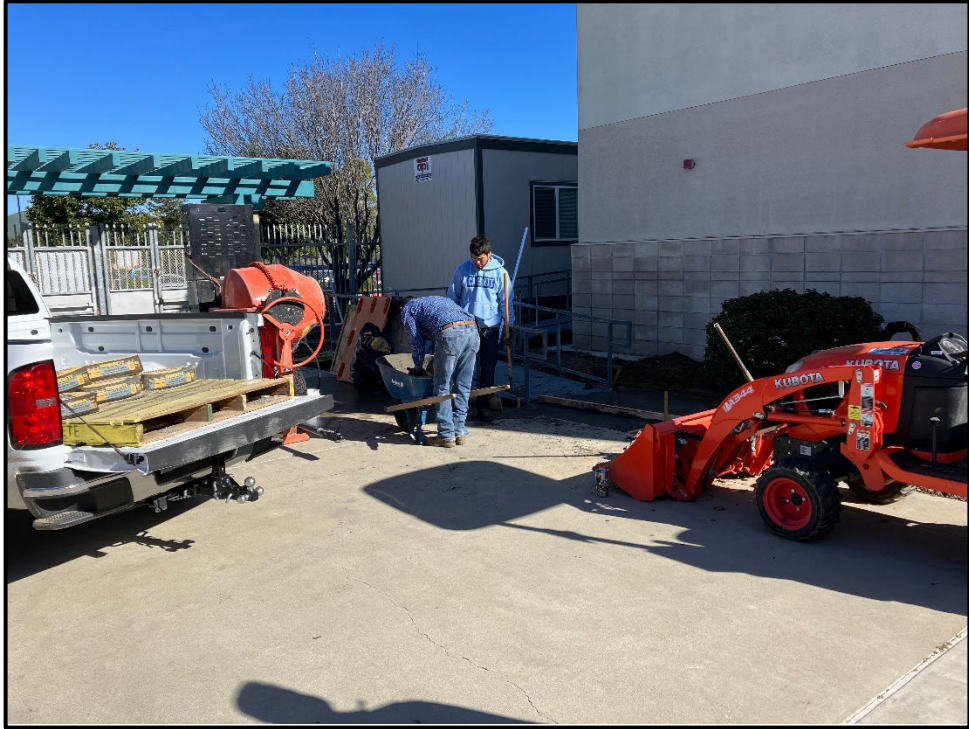
PVHS – Jose Gamino and Chase Richardson Pouring Concrete for the IT Trailer
