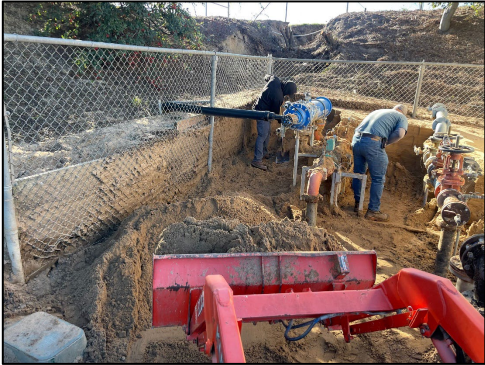
ERHS – Erik Escobar and Joseph Campos Repairing Damage Caused by Storm Erosion
