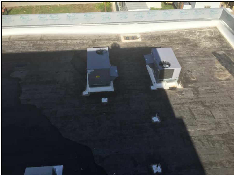
PVHS Performing Arts Center – Built-up Roof and HVAC Installation In-progress
