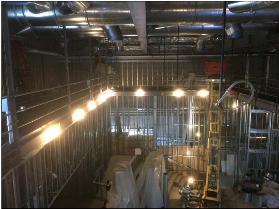
PVHS Performing Arts Center – Interior Finishes Installation Underway
