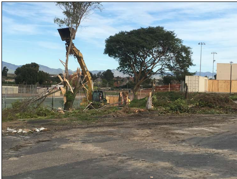
ERHS 38 Classroom Building – Construction Begins over Winter Break
