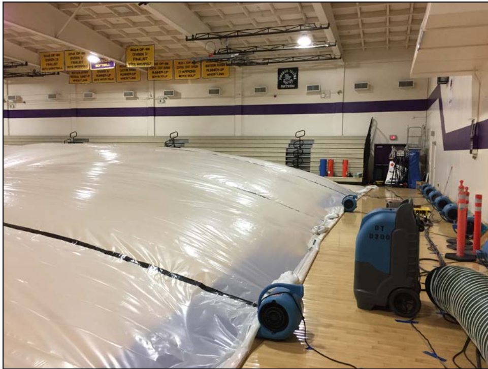
ERHS - Gymnasium Water Restoration in Full Swing
