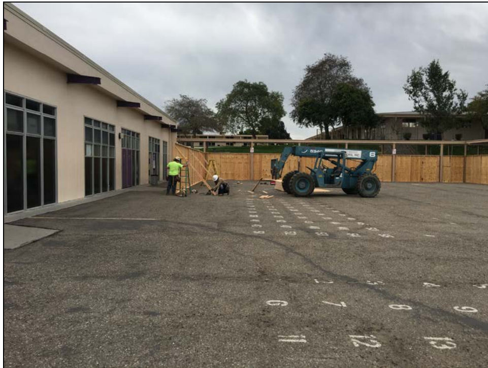
ERHS 38 Classroom Building – Barriers Installed to Separate Construction & School
