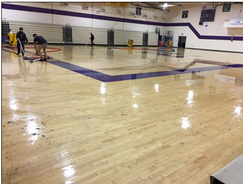
ERHS – Gymnasium Fire Sprinkler Water Leak; M&O Team Begins the Clean-up
