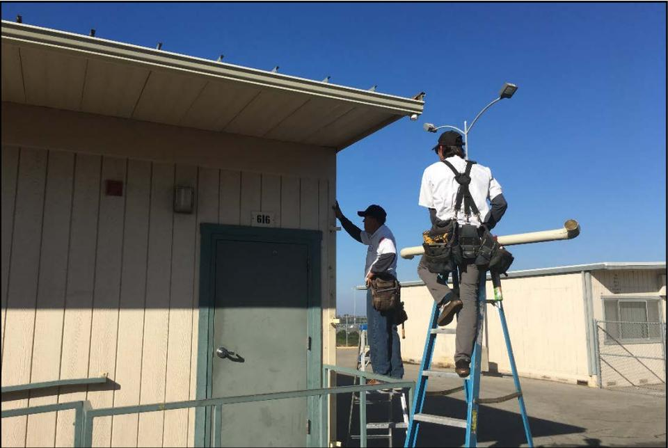
ERHS - Rain Gutter and Downspout Installation Underway
