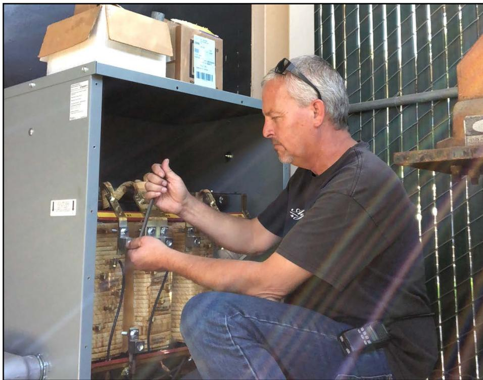
ERHS – Del Ward Prepares Power and a New Transformer for the Ceramic Kilns
