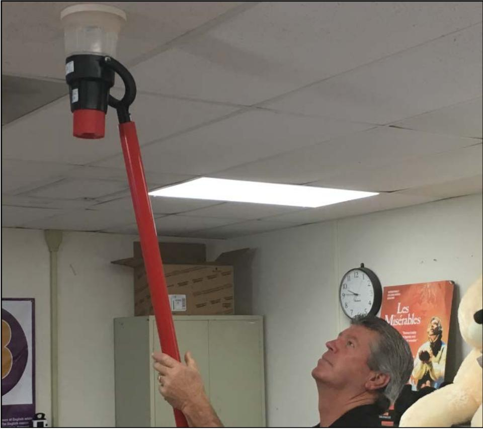
ERHS - Testing Fire Alarm Devices per NFPA 72
