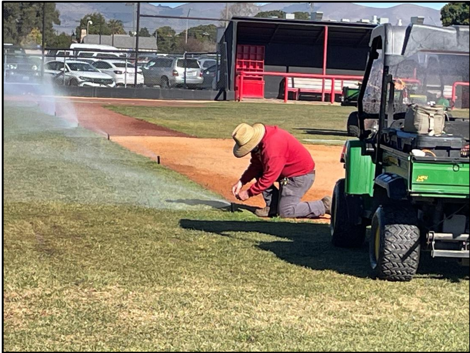
SMHS – Jordan Markstone Repairing Sprinkler Heads
