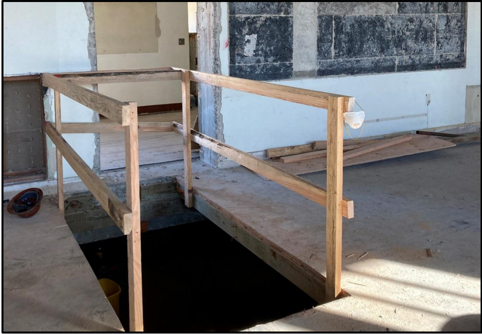
SMHS Admin to Classroom – Subfloor Access for Plumbing and Electrical Installation
