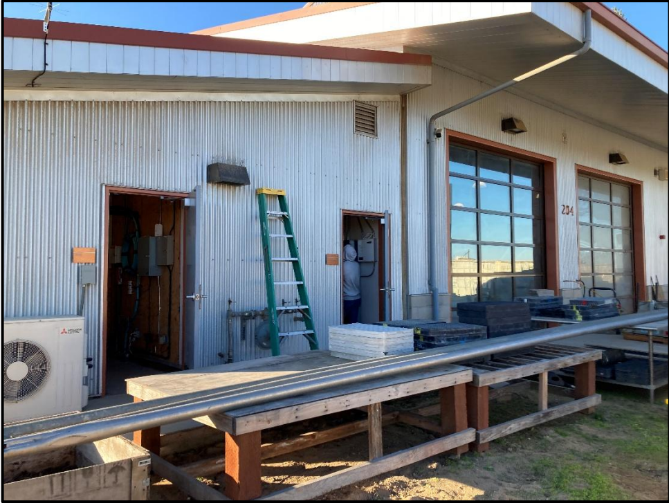
MRCTECAF M&O Building – Locating Utilities for New Building
