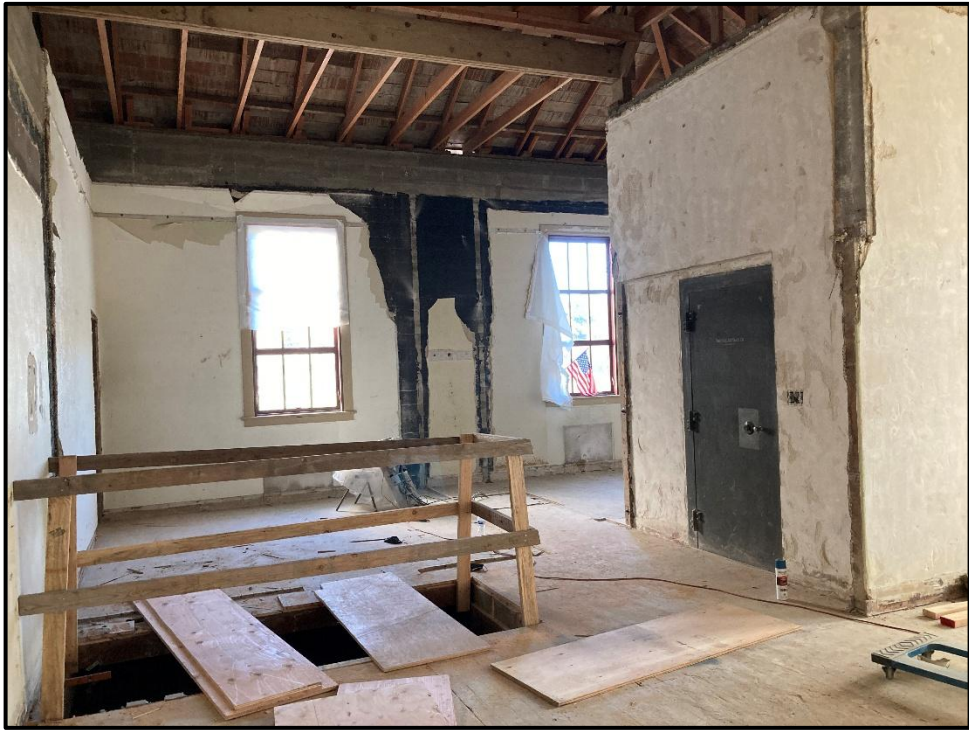
SMHS Admin to Classroom – Exposed Ceiling for HVAC Installation
