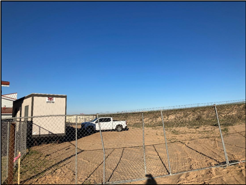
MRCTECAF M&O Building – Grading, Fencing, and Construction Office Being Installed
