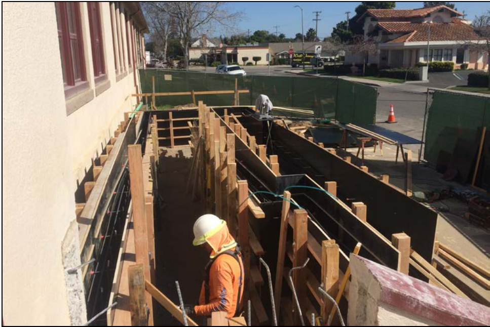
SMHS – The New Parking Lot Requires a New Ramp for the Front Entrance
