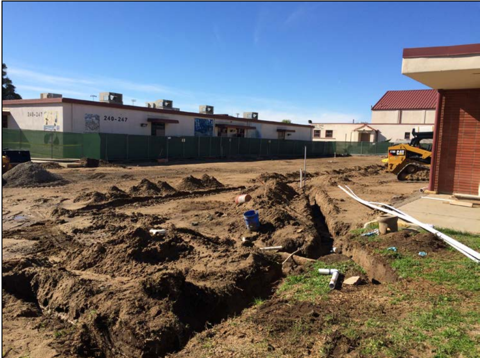
SMHS – New Visitor Parking Lot Underground Utilities Relocation Underway
