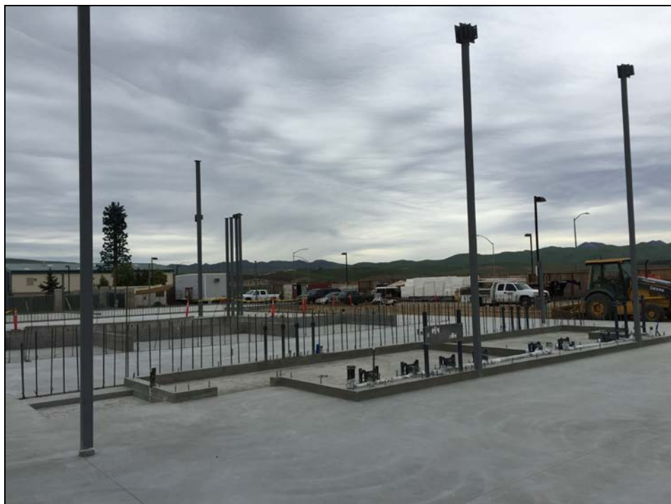
PVHS – Performing Arts Center Foundation Awaits Structural Steel. Dramatic Background adds to the Excitement and Anticipation
