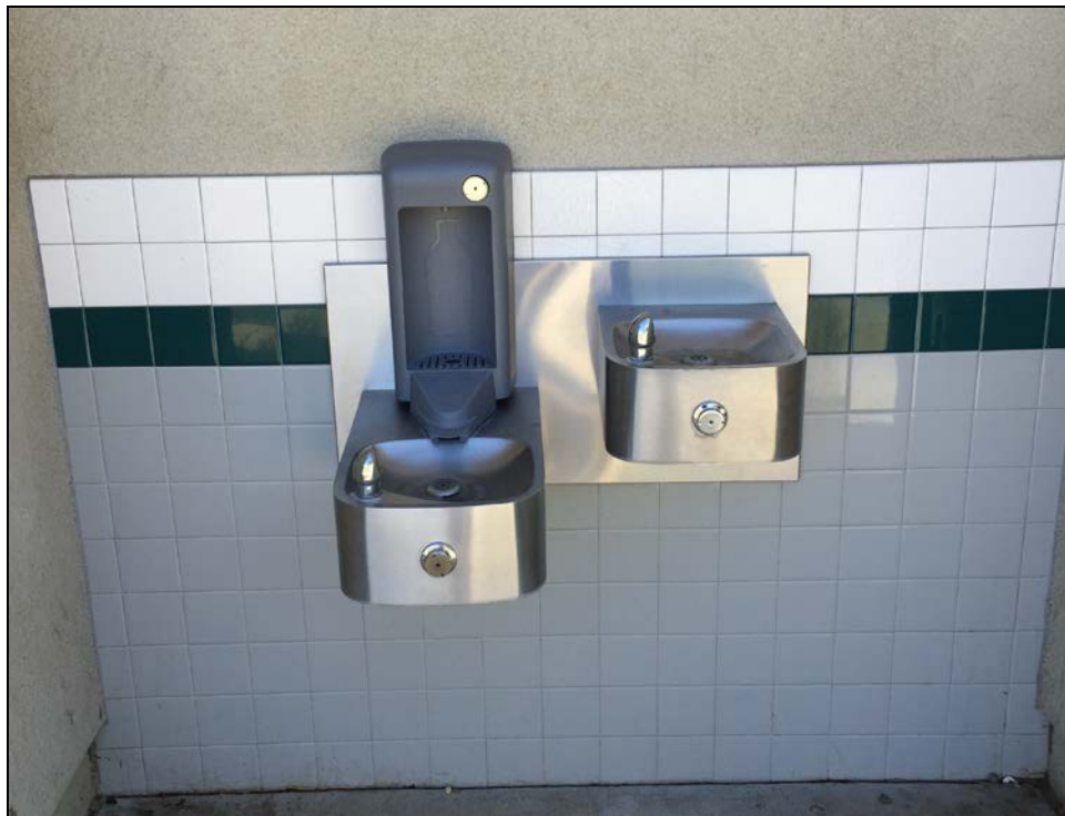
PVHS - Two Hydration Stations Installed on the 300 and 400 classroom Building Exteriors
