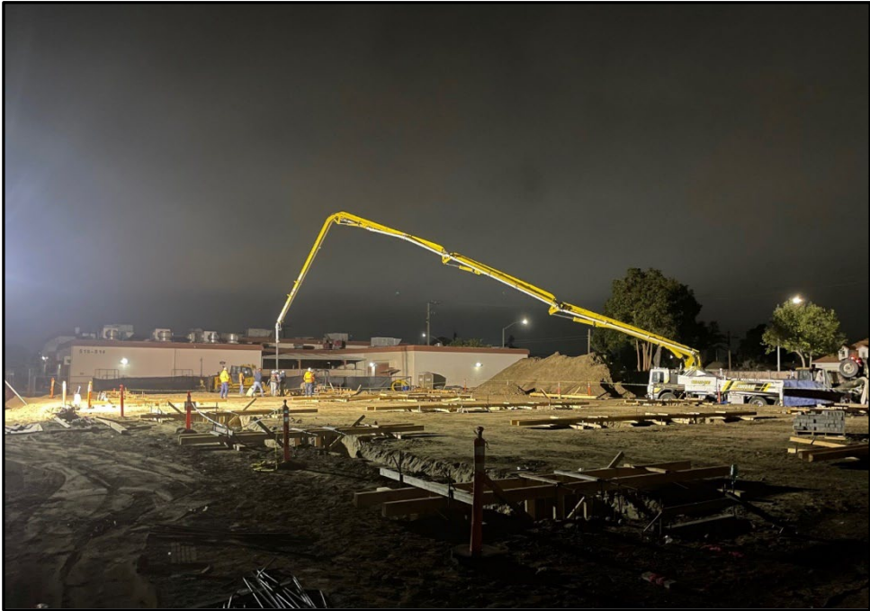
SMHS 50-Classroom Building – Early Morning Concrete Pouring for Footings
