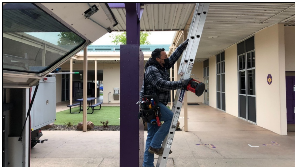
ERHS – Bernie Rayner Heads onto the Roof to Repair a Heating Unit
