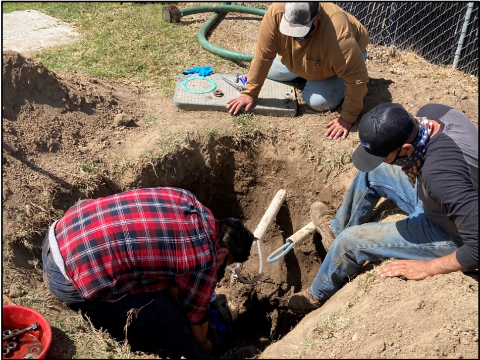
PVHS – Grounds Crew Repairs the Gopher Control Chemical Dispenser at the Irrigation Well
