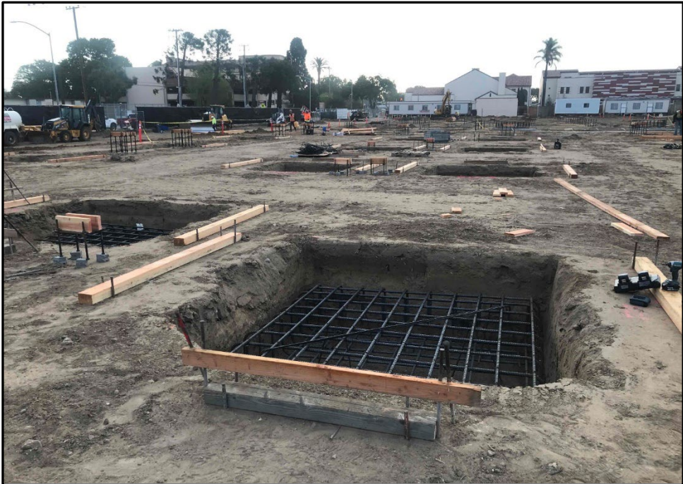
SMHS 50-Classroom Building – Footings and Rebar in Place
