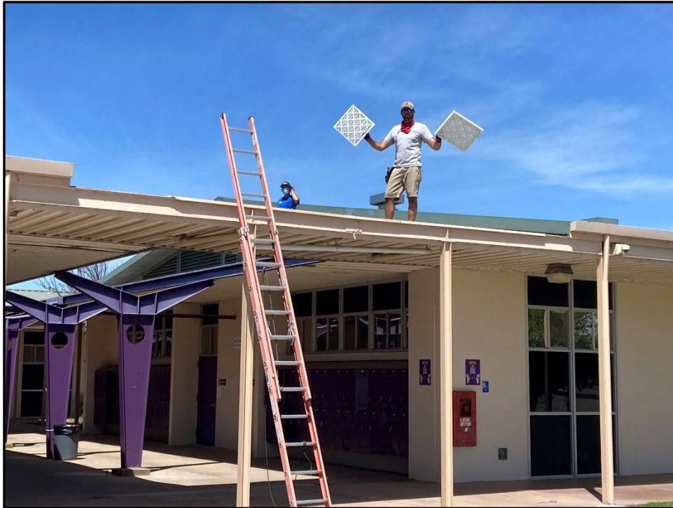
ERHS – MERV 13 Air Filters are Installed throughout the District
