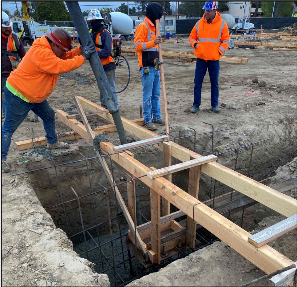
SMHS 50-Classroom Building – Three Story Footings are HUGE!!!
