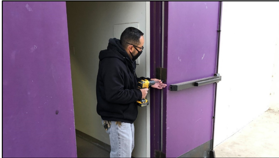
ERHS – Jimmy Salutan Inspects and Repairs Campus Doors
