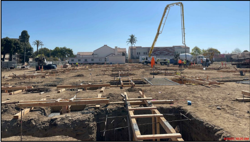
SMHS 50-Classroom Building – Pouring of Footings Continues
