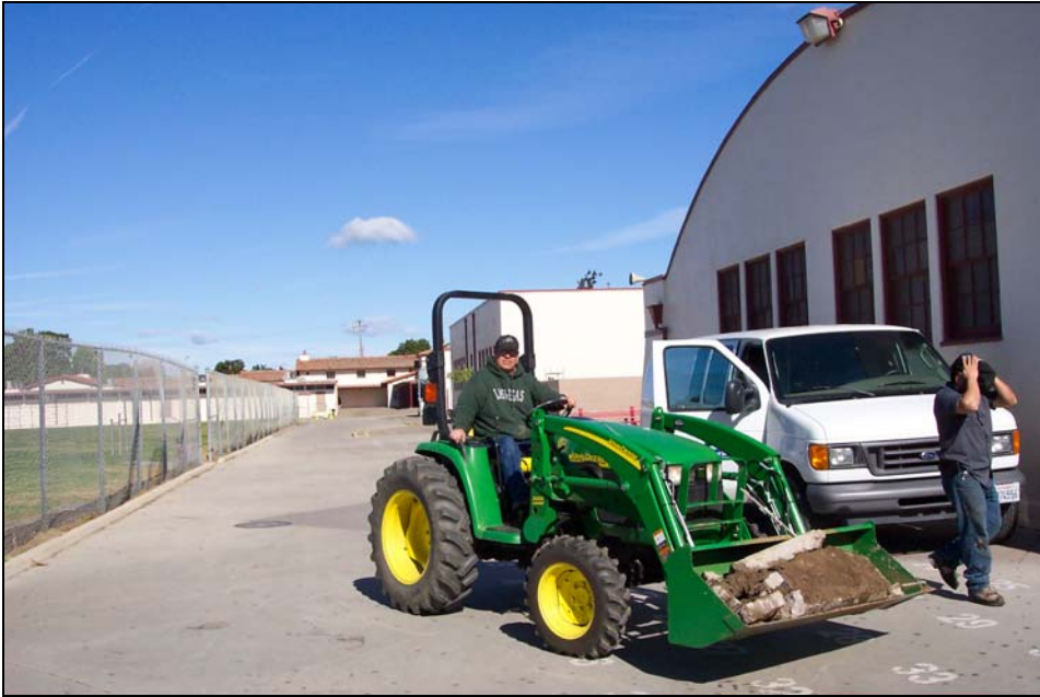
SMHS - Repairing a Collapsed Irrigation Conduit Near the Small Gymnasium
