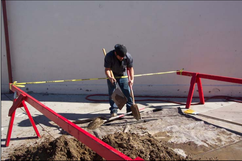
SMHS – Repairs Can Get Messy
