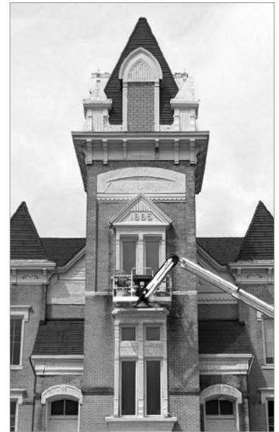
Joshua Davis works on wrapping the new Ad Building windows. Over the summer, the new roof and windows were installed, and metal work was completed.
