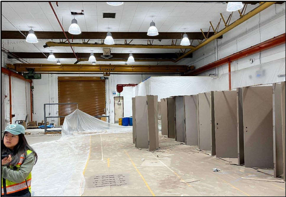
SMHS CTE Modernization – New Interior and Exterior Doors are Being Painted
