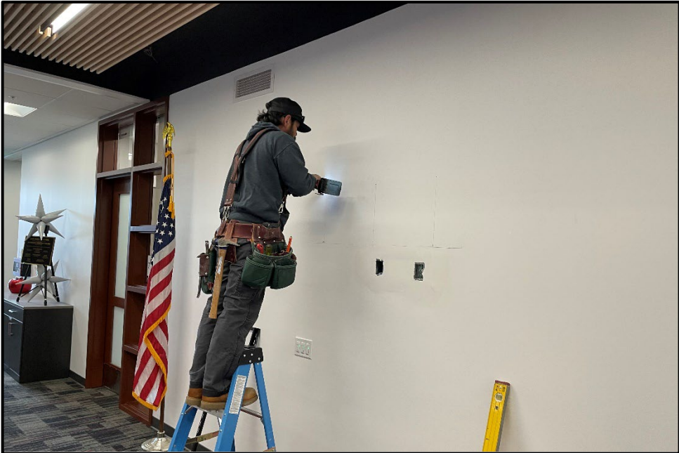
SMHS – Tom Harbold Installs New Monitor Brackets in the Administration Building
