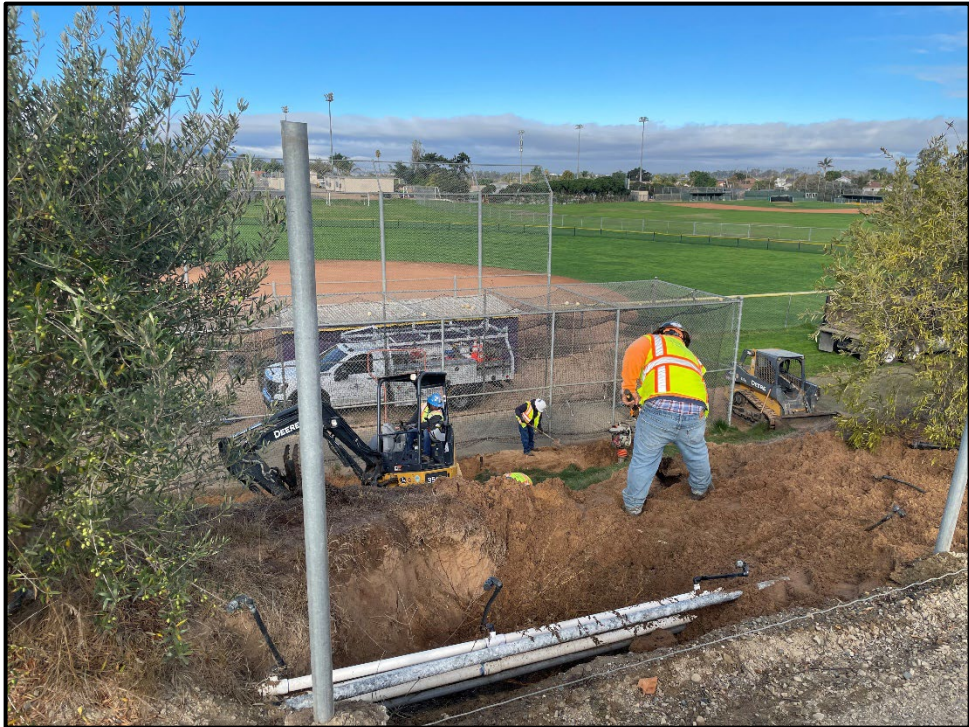
ERHS Slope Stabilization – Repairing the Slope East near the Softball Field
