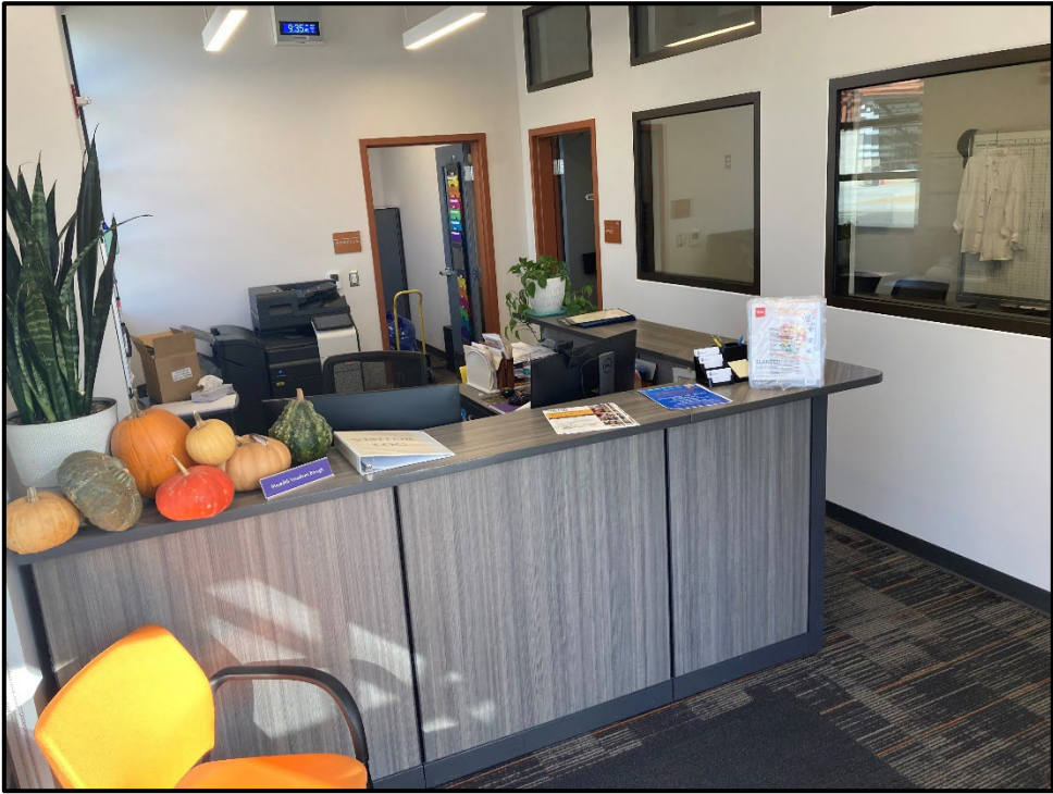
MRCTECAF Front Office Space Design – Nearing Completion
