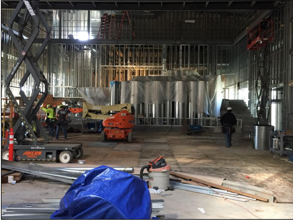
PVHS – The Sloping Theater is Filled and Covered to Avoid Scaffolding
