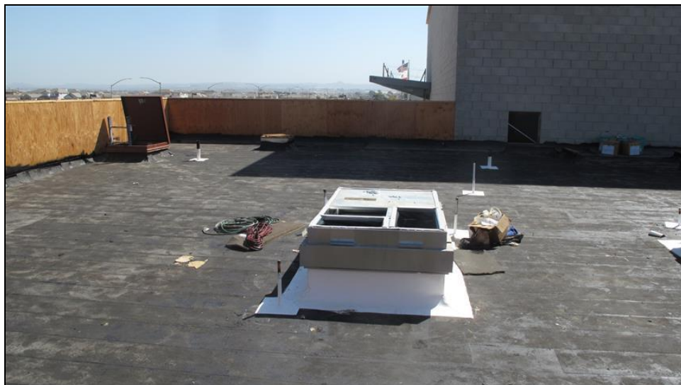
PVHS – Performing Arts Center Roofing Base Sheets Applied
