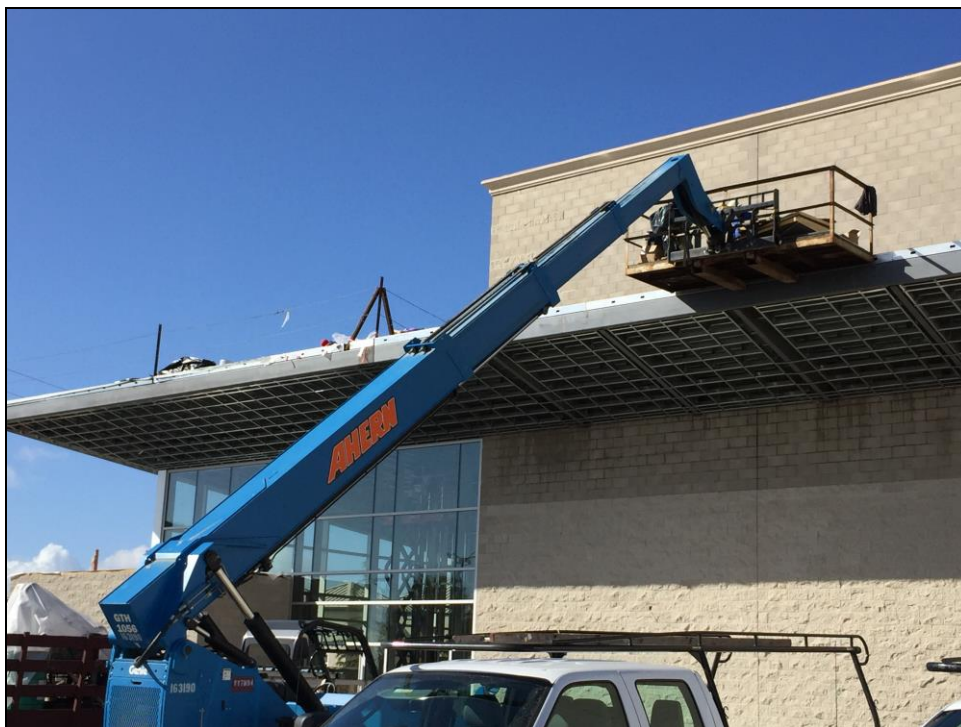
PVHS – Installing Insulation on the Performing Arts Center Roof
