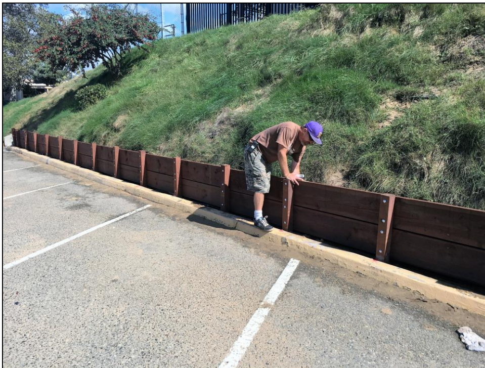
ERHS – Denton Tilley Assembling a New Retaining Wall at the Student Parking Lot
