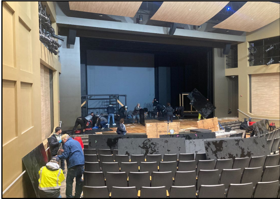
PVHS – Students and Staff Removing the Performing Arts Center Stage Flooring
