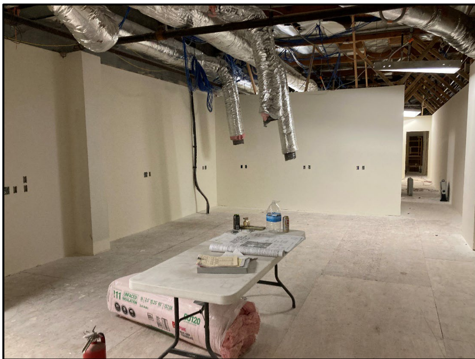
SSC Second Story Reconfiguration – Wall Finishes Near Completion and HVAC In-Progress
