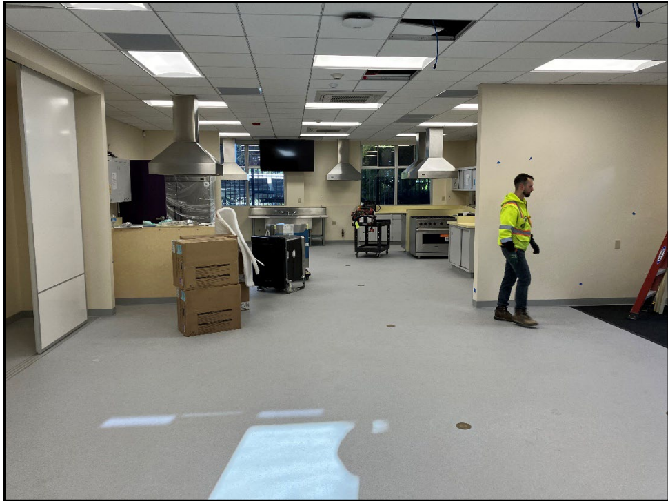
ERHS Modernization – Foods Lab New Exhaust Hoods in Place
