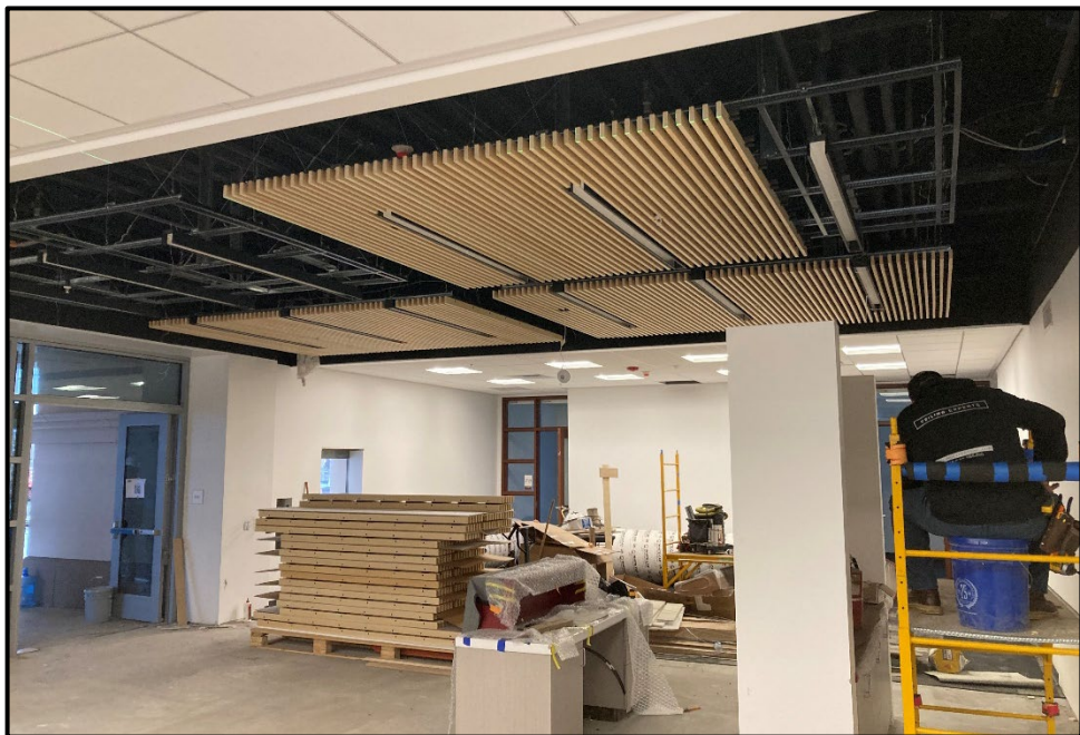
SMHS 50-Classroom Building – Main Hallway Finished Ceiling Installation Underway
