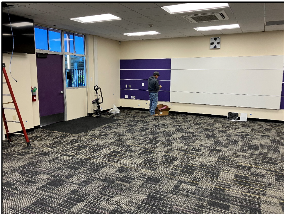
ERHS Modernization – Interior Finishes are Finalized in the West 100 Building Classrooms
