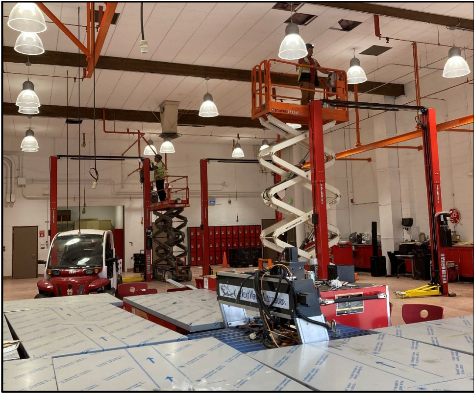
SMHS CTE Modernization – Installing Power to the Newly Installed Vehicle Lifts
