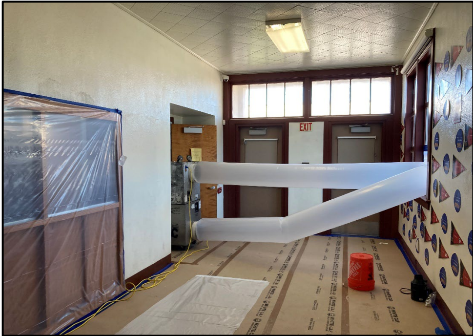
SMHS Admin to Classroom – Asbestos Abatement Ongoing
