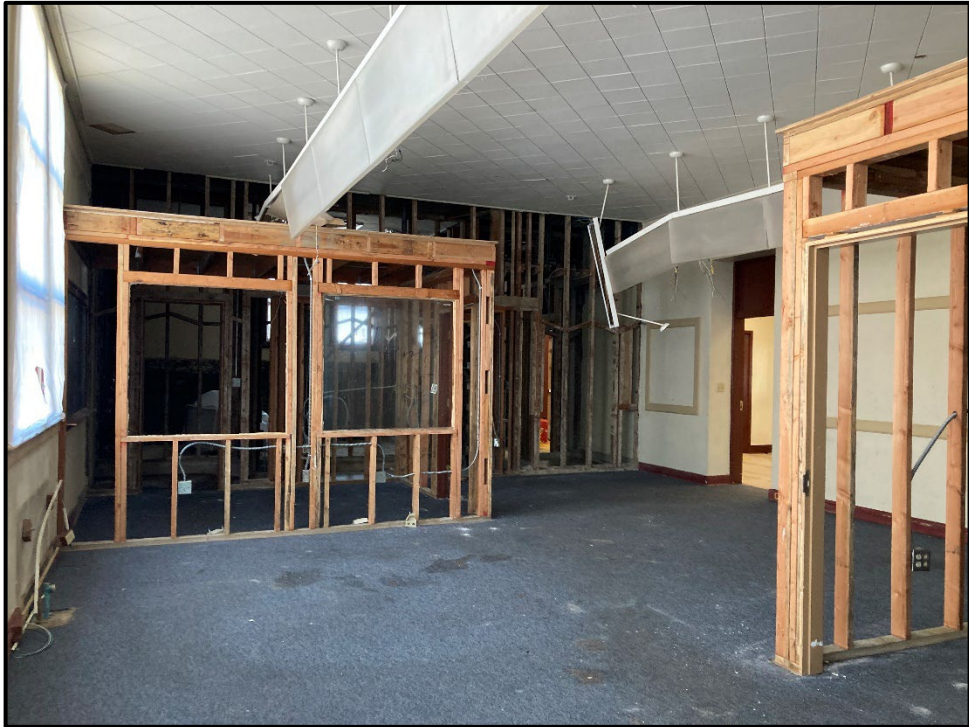
SMHS Admin to Classroom – Demolition of all Interior Walls is Ongoing
