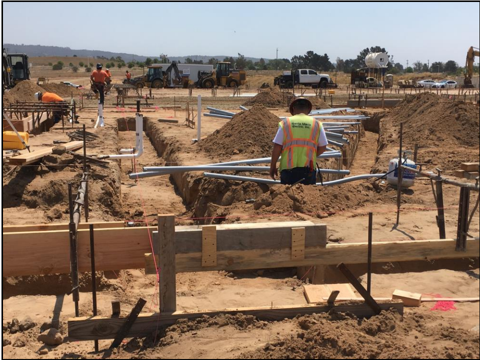
CTE Ag Center – Underground Utilities Go into Place for the Shop Buildings
