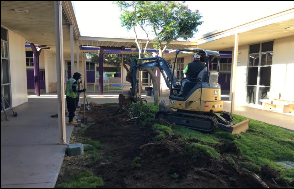
ERHS – Demolition Begins for a Native Garden in the Science Building Courtyard
