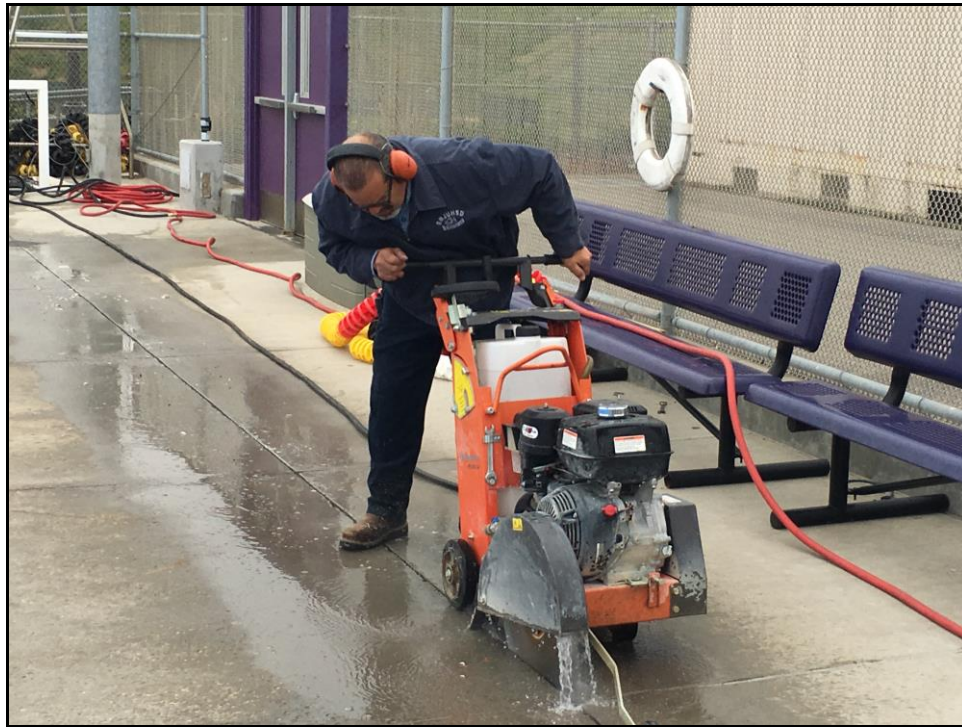
ERHS – José Placencia Cuts Drain Slots on the Pool Deck
