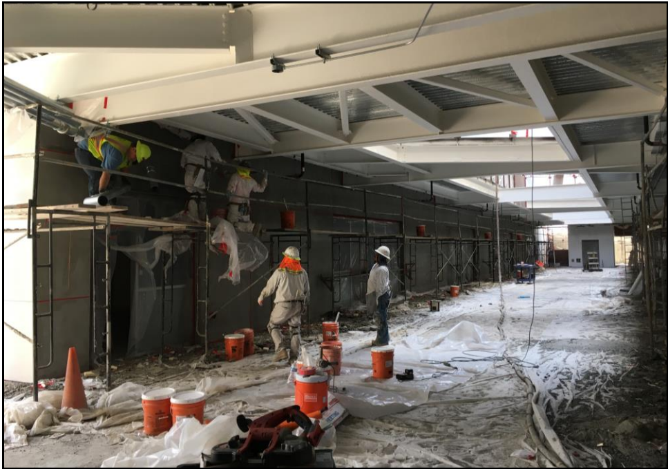
ERHS 38-Classroom Building – Exterior Stuccoing is Underway Throughout the Building
