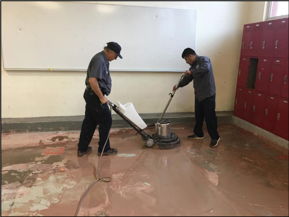
SMHS – James Harvey and Miguel Sanchez Polish the Concrete in the Boys’ Locker Room
