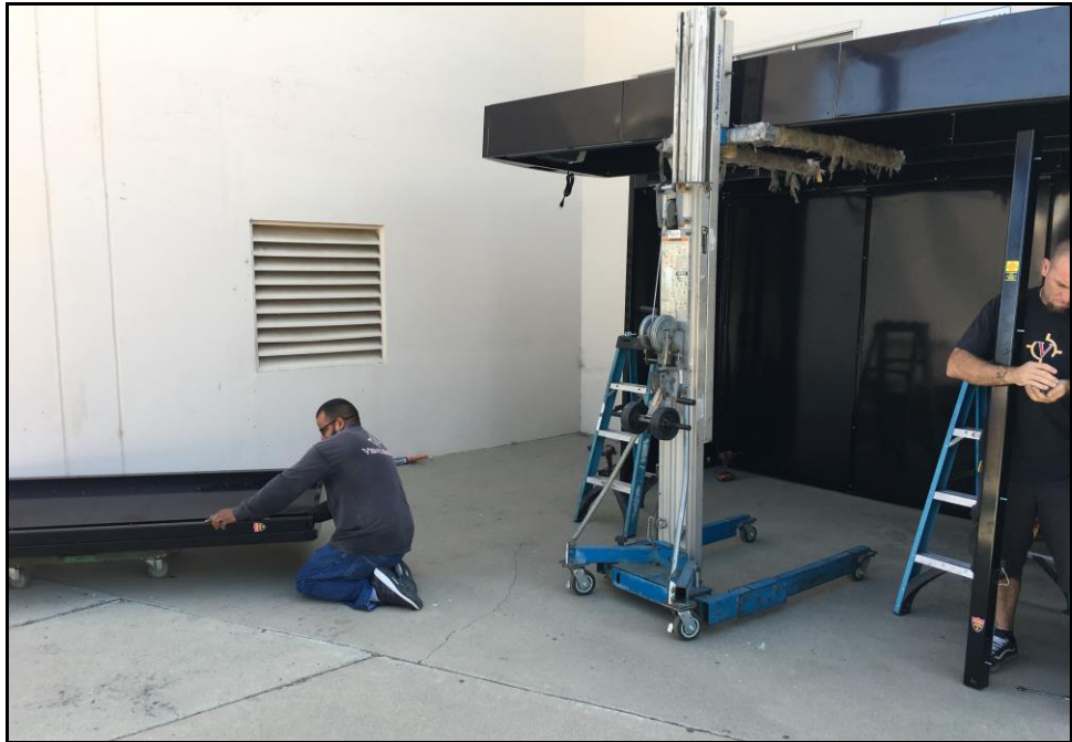
ERHS – New Satellite Food Service Station Assembled Near the Gymnasium
