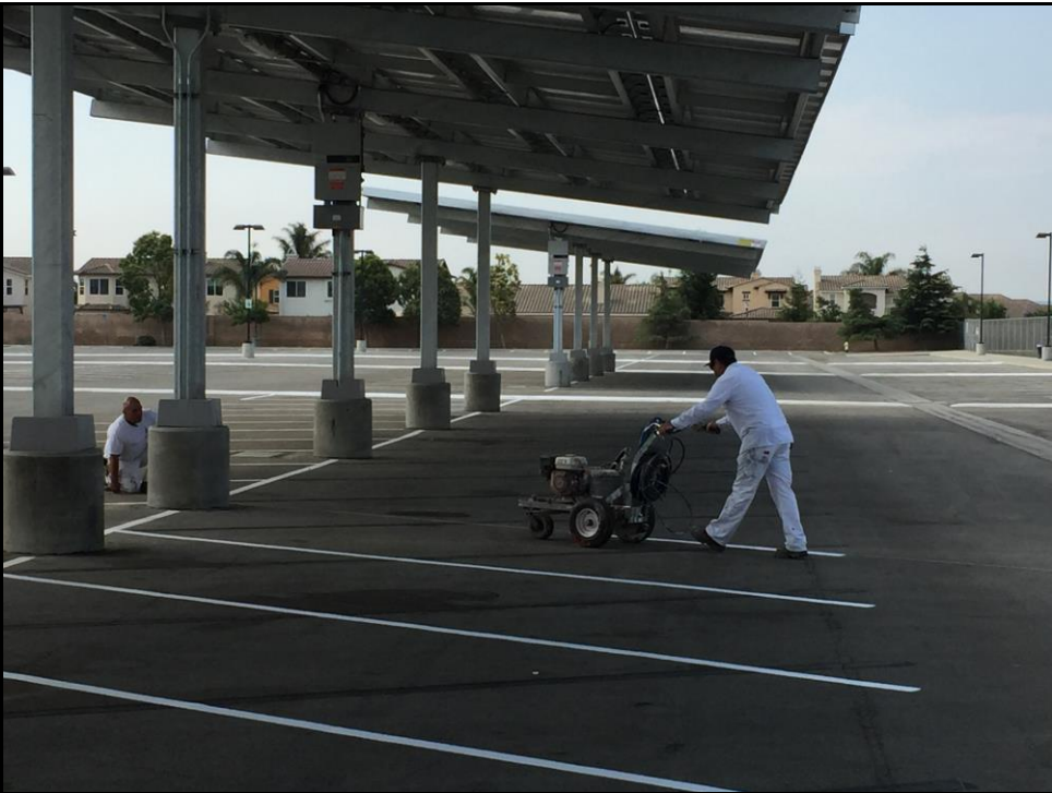
PVHS – Ernest Paz and Ray Segovia Restripe the Student Parking Lot
