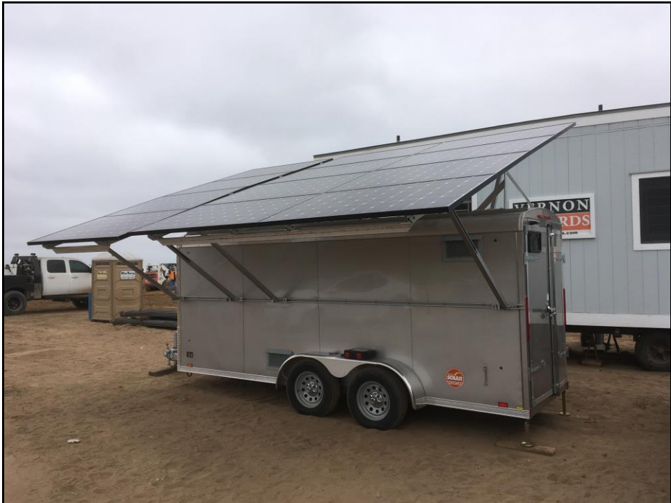
CTE Ag Center – Temporary Power for Construction is Provided by a Mobile Solar Plant
