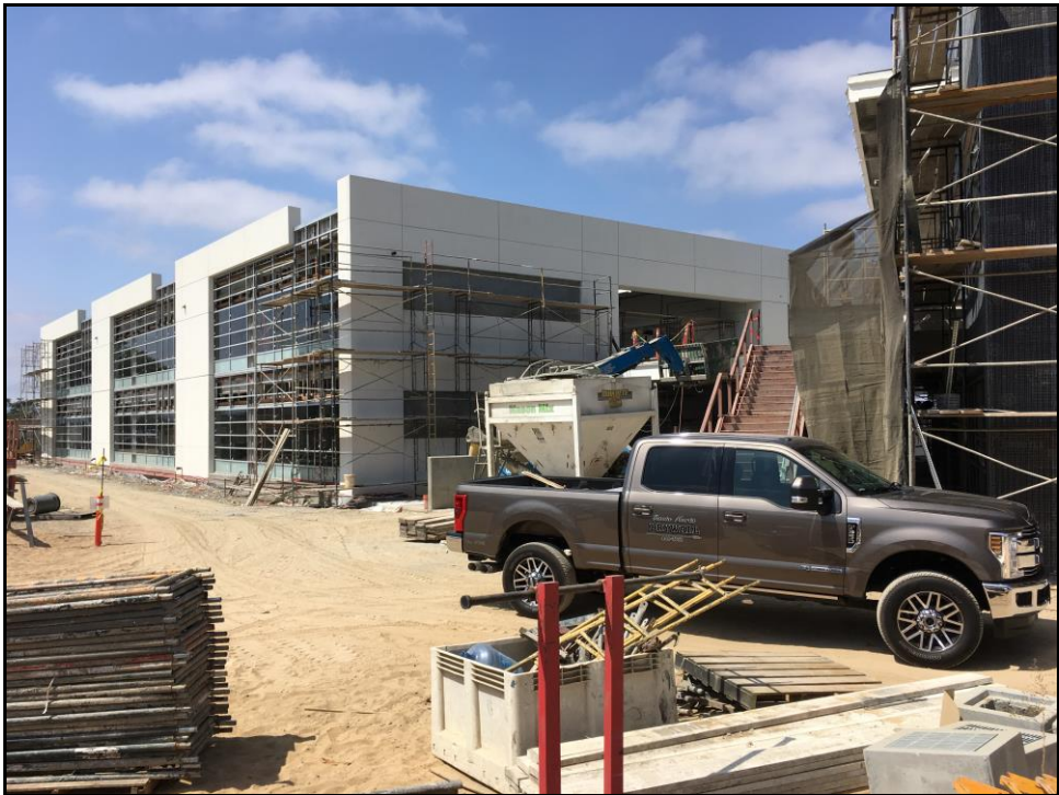
ERHS 38-Classroom Building – Stucco Batch Plant in Place to Mix Mortar on Site
