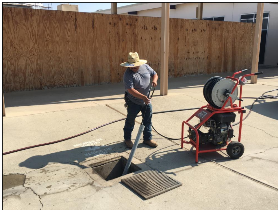
ERHS – Jesus Reyes Clears the Storm Drain Near the Gymnasium
