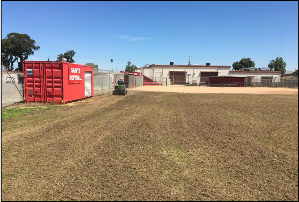
SMHS – Alan Rodriguez Works on the Softball Field Outfield Renovation
