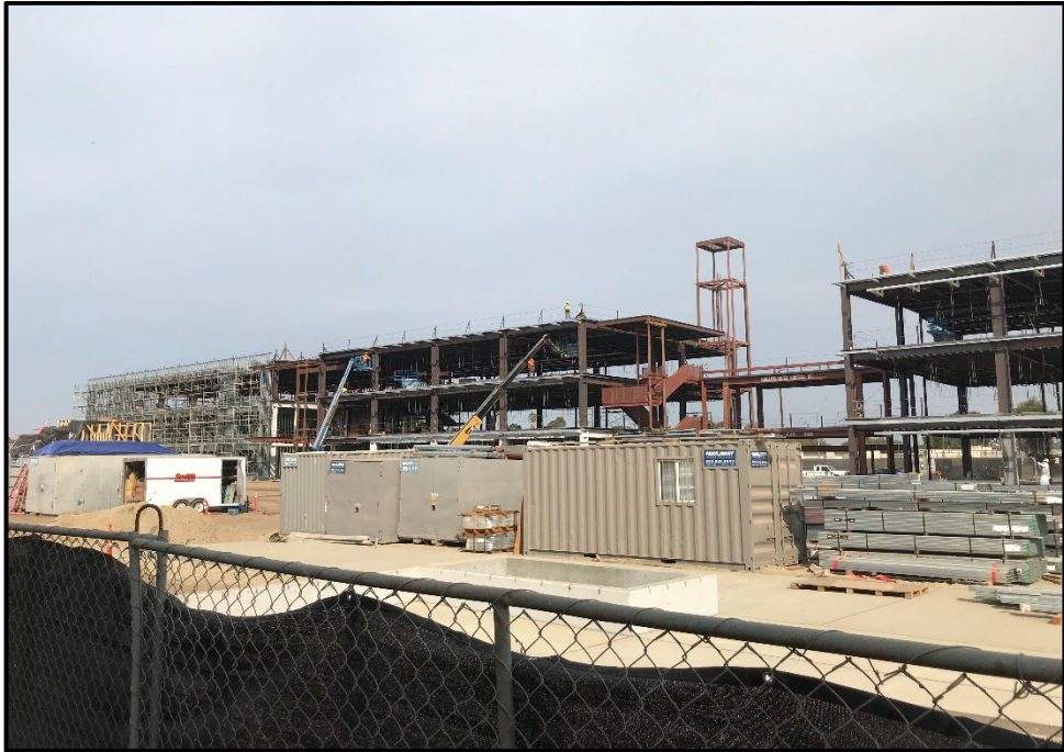
SMHS 50-Classroom Building – Overall View from the School Campus Shows the Students’ View of Construction
