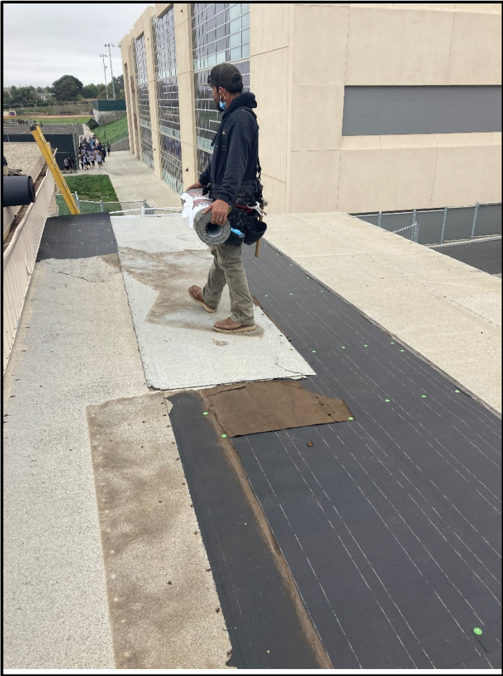
ERHS – Tom Harbold Reroofs the Ag Science Building Storage Area
