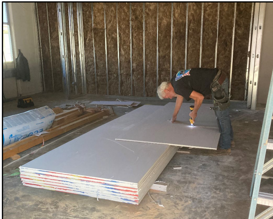
ERHS Modernization – Drywall Installation Begins in Earnest
