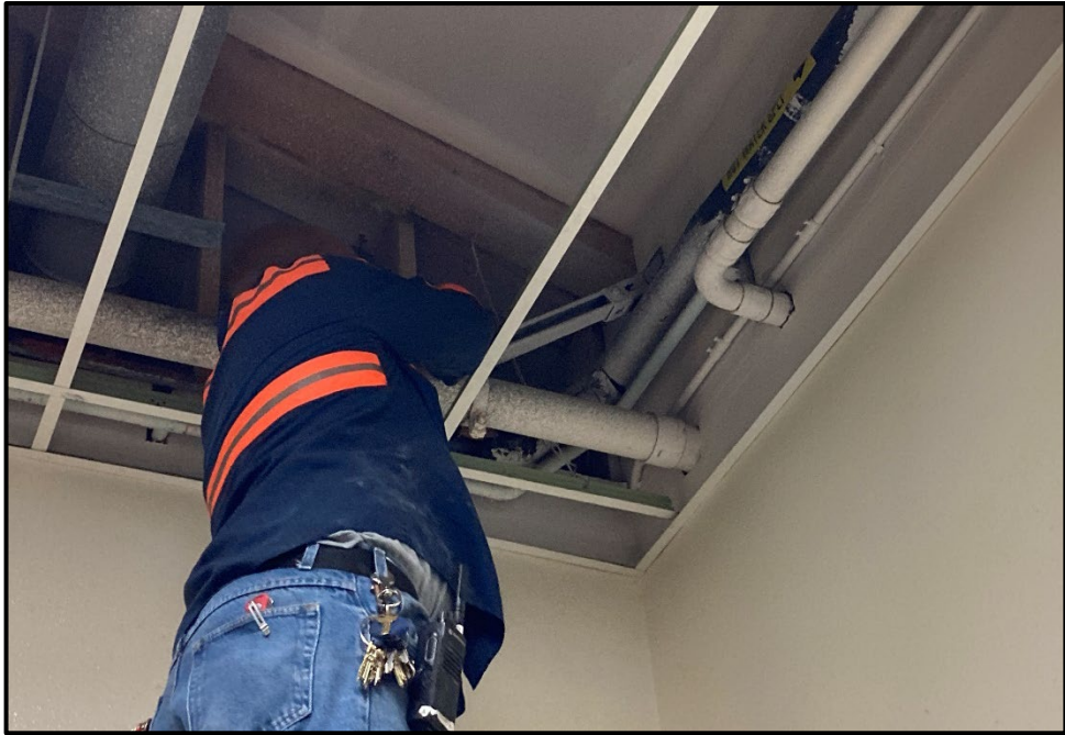
SMHS – Alex Anguiano Alcaraz Investigates a Water Leak in the Cafeteria Kitchen Attic
