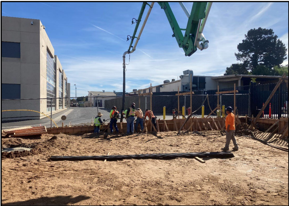
ERHS Maintenance and Operations Building – Retaining Wall Concrete Pour in Progress
