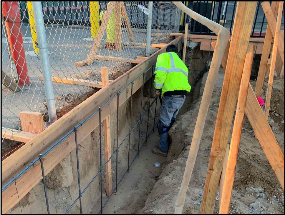
ERHS Maintenance and Operations Building – Forming for Retaining Wall is Underway
