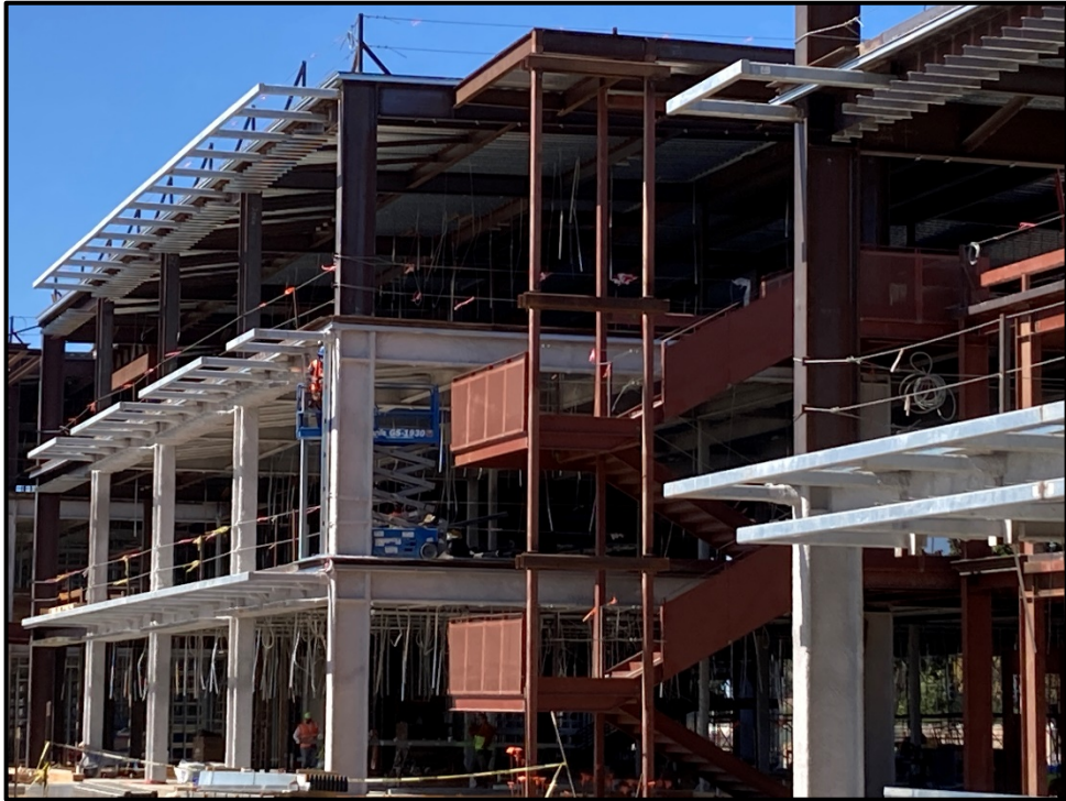
SMHS 50-Classroom Building – Light-colored Tubular Stand-offs will Support Architectural Panels
