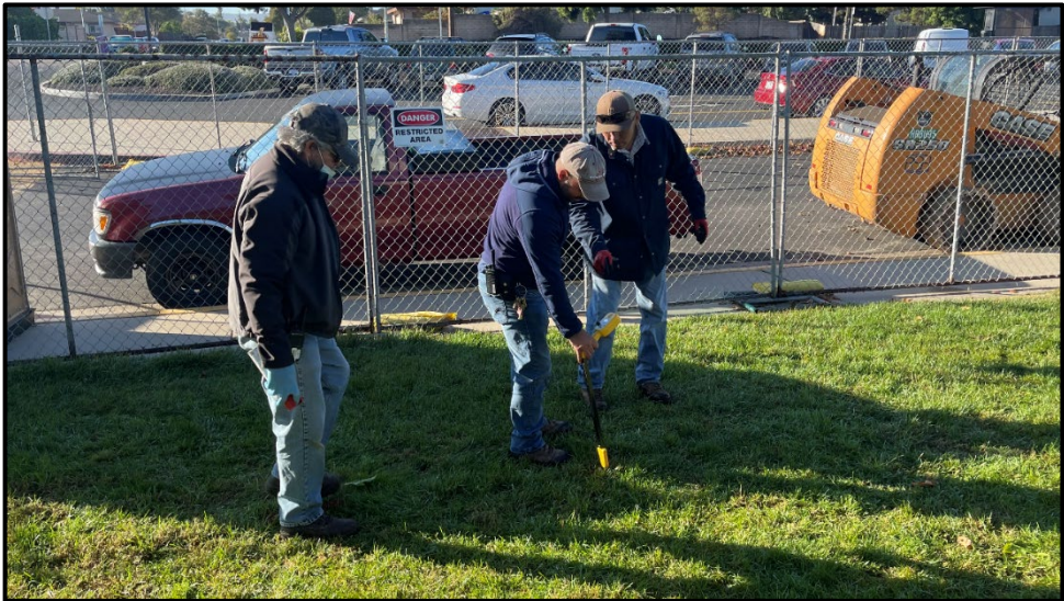
ERHS – The Grounds Crew Uses a Locating Device to Find a Broken Irrigation Wire
