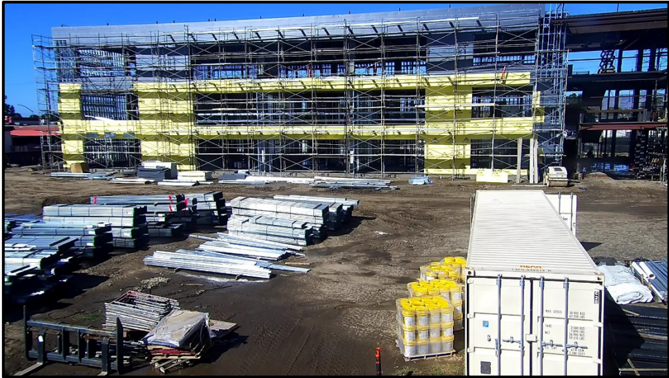
SMHS 50-Classroom Building – Exterior Insulation Begins to Enclose the Building
