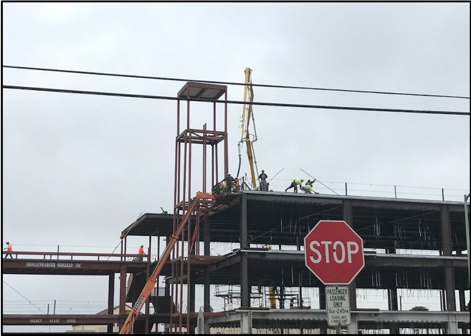
SMHS 50-Classroom Building – Pumping Concrete for the Roof
