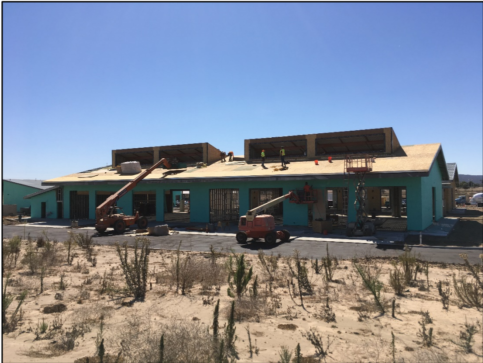
CTE Ag Center – Roofing Begins on the Shop Buildings
