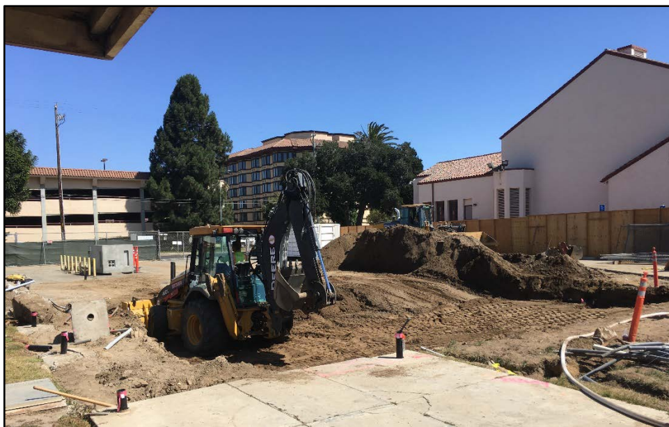
SMHS Reconstruction – Excavation Begins for the New Power House Foundation
