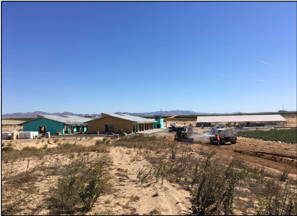
CTE Ag Center – Forging a New Access Road
