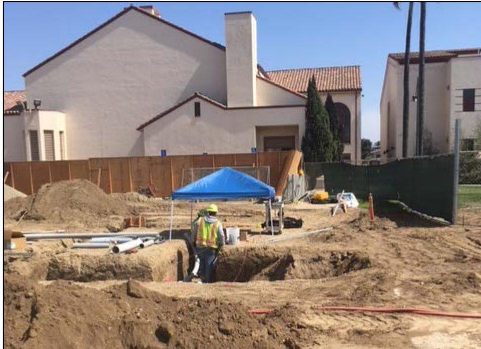
SMHS Reconstruction – Electricians Prepare Conduit and Vaults for Power Distribution Lines
