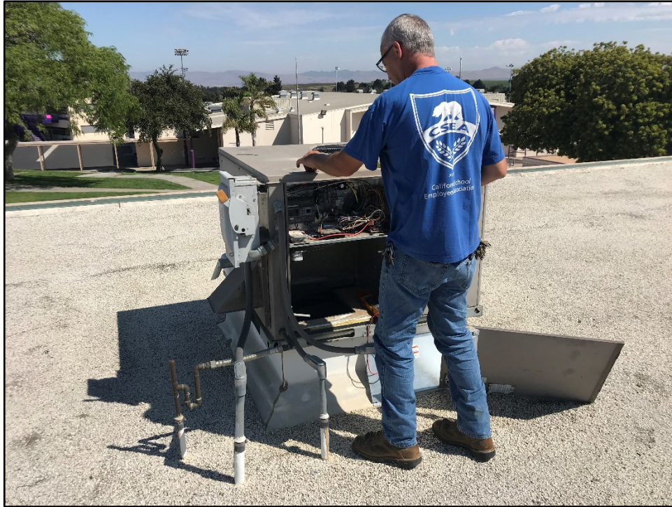
ERHS - Del Ward Investigates HVAC Issues at the Administration Building
