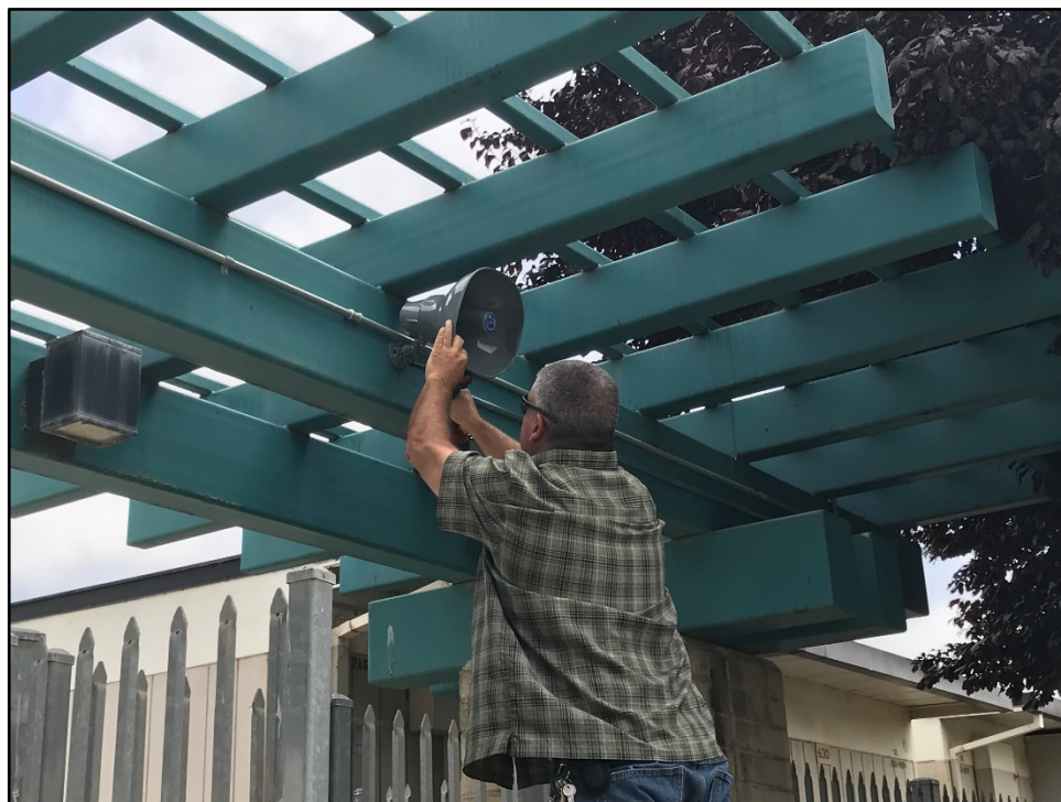
PVHS – Andy Freitas Installs a Public Address Speaker to Cover the Softball Fields
