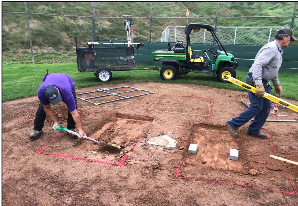
ERHS – Grounds Crew Installs New Clay Brick in the Junior Varsity Batter's Box
