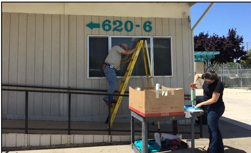
PVHS – New Building Signs Improve Identification for Daily Use and Emergency Events
