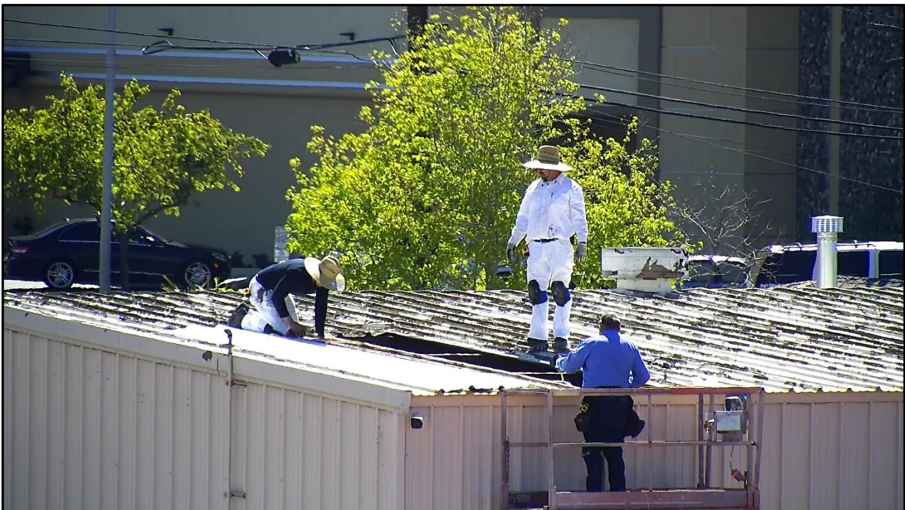
SMHS - District Maintenance Crew Replaces a Skylight with Metal Roofing
