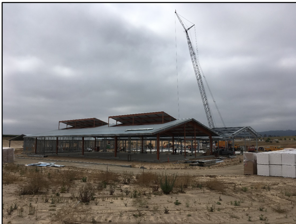
CTE Ag Center – Shop Building B Roof Decking Installed
