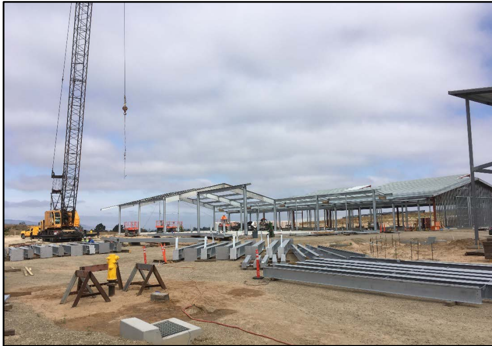
CTE Ag Center – Structural Steel Arranged to Set in Place
