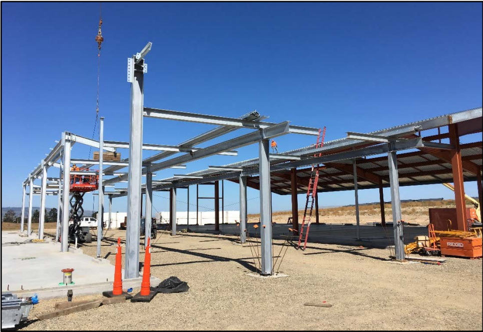
CTE Ag Center – Steel for the Trellis Between Shop Buildings is Underway
