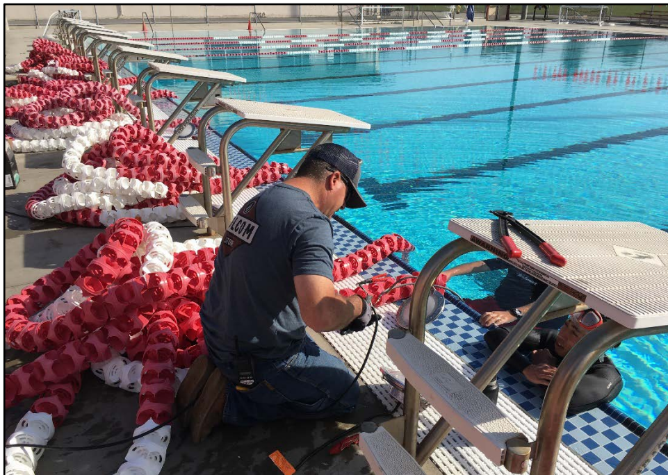
SMHS – Andy Freitas Works On-Deck While a Diver Replaces Pool Lights
