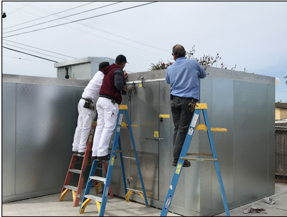
ERHS – District Maintenance Crew Assembles Agriculture Science Flower Cooler and Specimen Freezer
