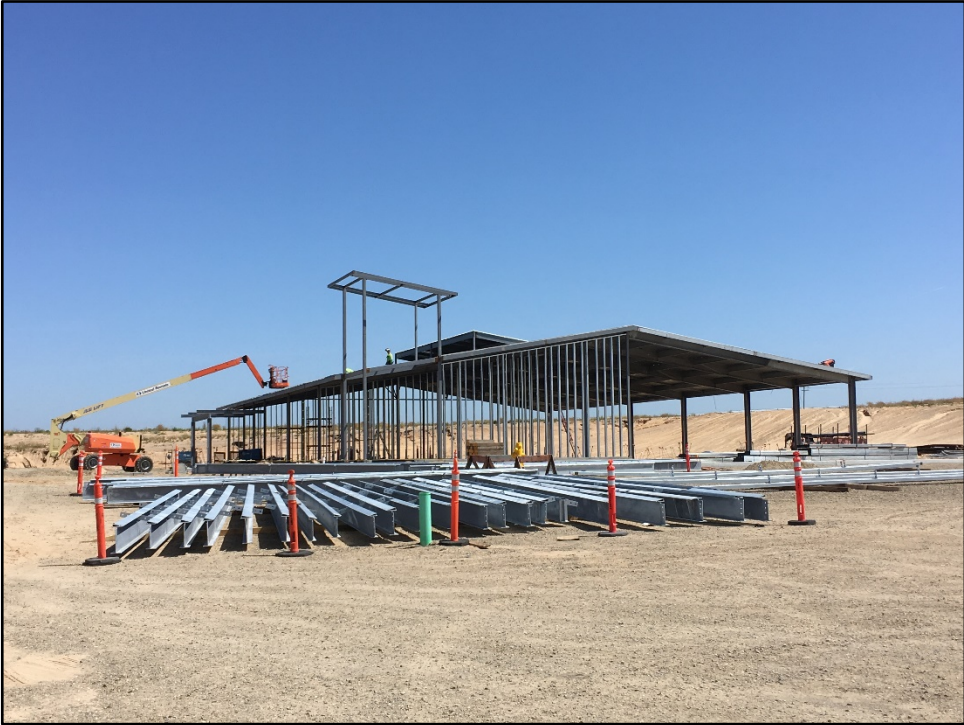
CTE Ag Center – Culinary Arts Building Tower Takes Shape
