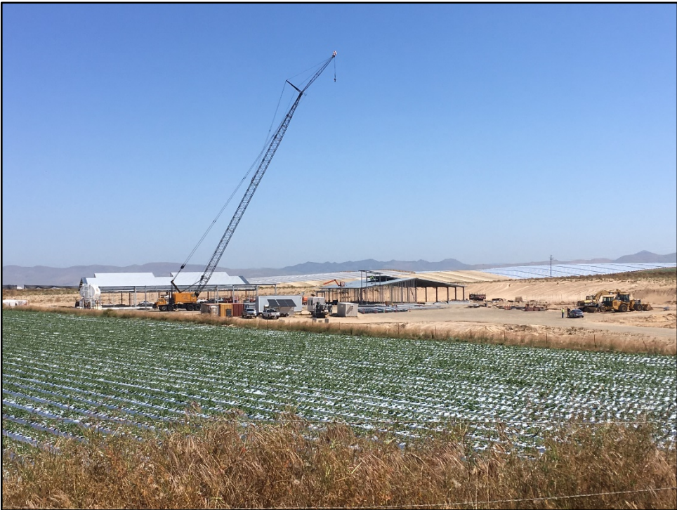
CTE Ag Center – Overall View of the Construction Site
