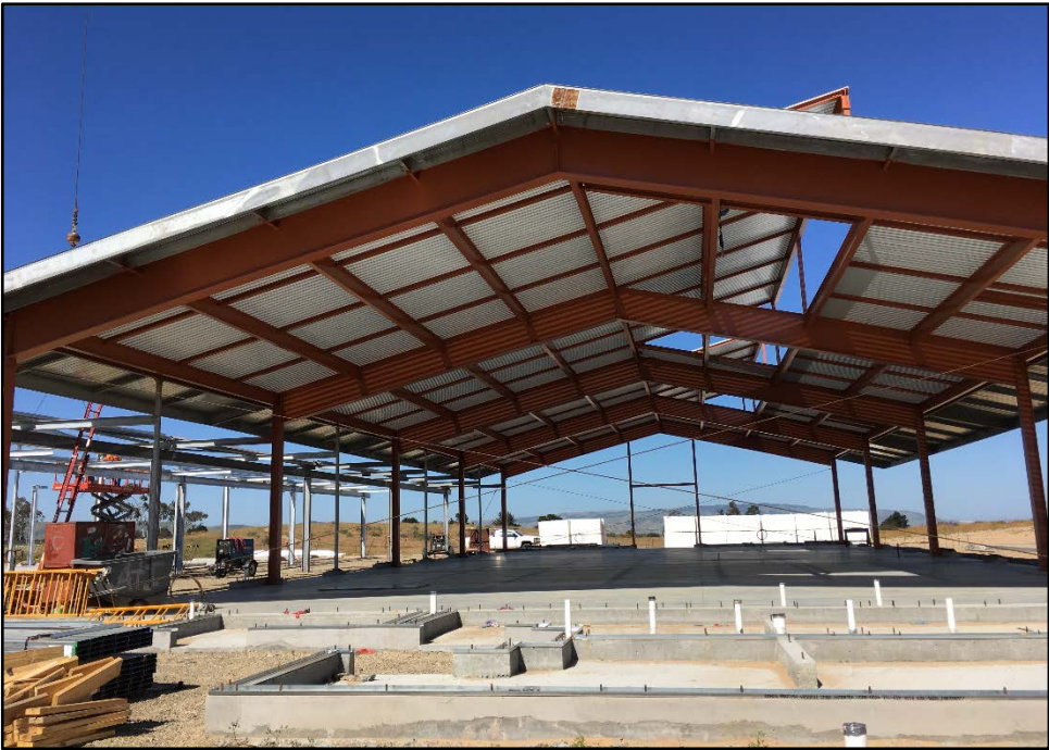
CTE Ag Center – Roof Decking for Shop Building B is Complete
