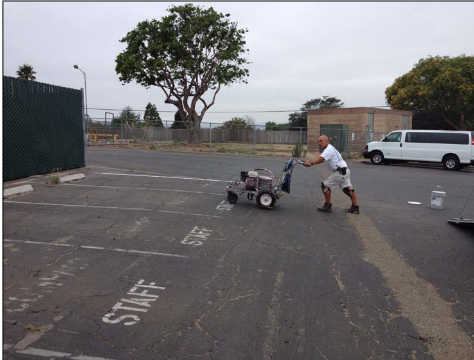
ERHS - Ray Segovia Restriping the Parking Lot
