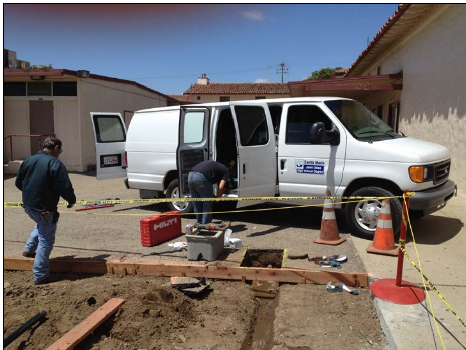
SMHS - José Placencia and Flavio Rodriguez Reroute a Water Line and Prepare to Replace Buckled Concrete at the Band Room
