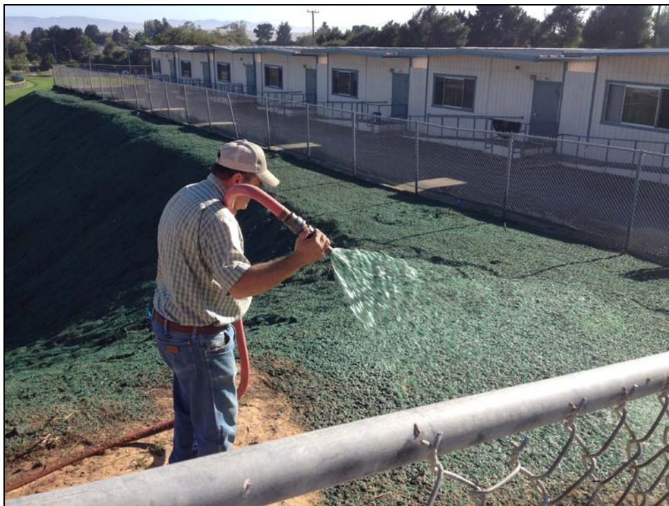
ERHS – 78,000 Square Feet of Hillside Receive Hydroseeding
