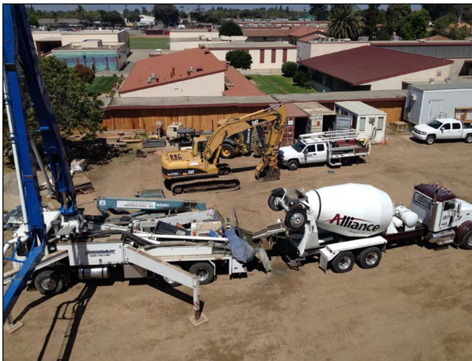
SMHS - 14 Classroom Building Concrete Pumping Station
