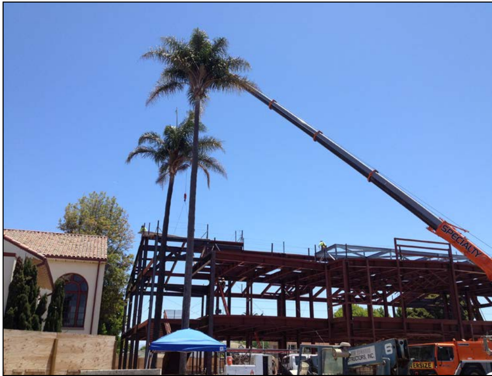
SMHS - 14 Classroom Building Metal Roof Decking Installation
