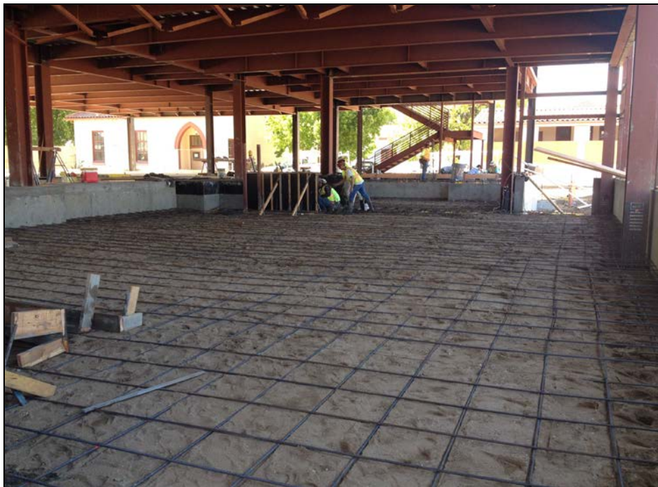
SMHS - 14 Classroom Building Ground Floor is Prepared for Concrete
