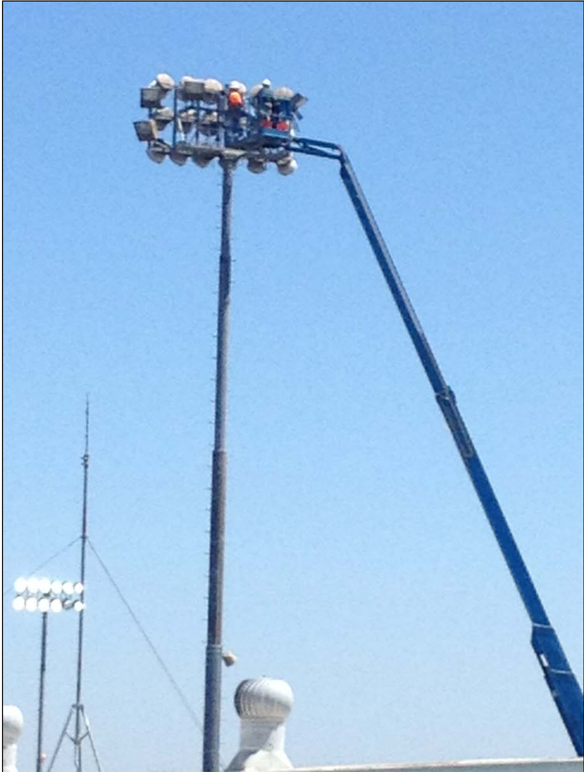
ERHS – Competition Lights Replaced High above the Football Stadium
