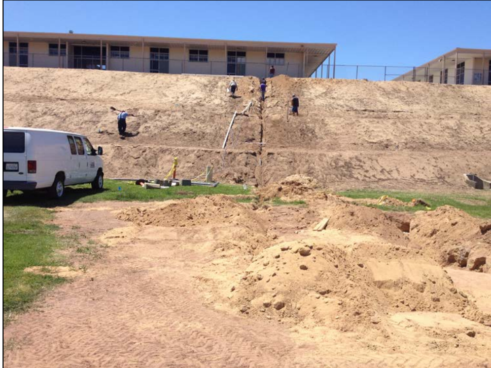
ERHS – Grounds Keepers from All School Sites Joined Forces to Install New Sprinklers
