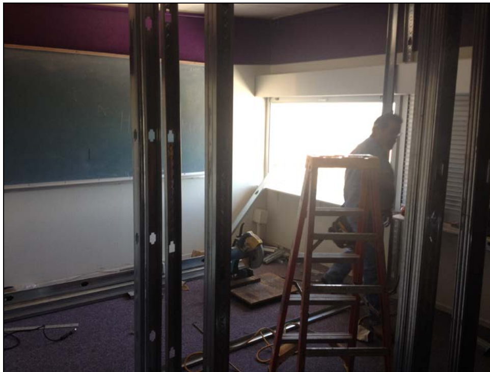
ERHS - Jose Placencia Performs Upgrades to the Press Box
