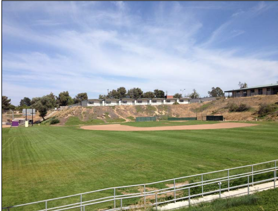
ERHS – Sports Field Hillside before Renovation
