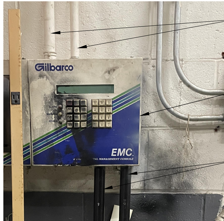
PHOTO 5 EXISTING TANK MONITORING SYSTEM
