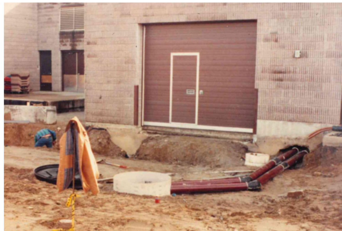
PHOTO 3 EXISTING TANK MANWAY SUMP AND UST SYSTEM PIPING
