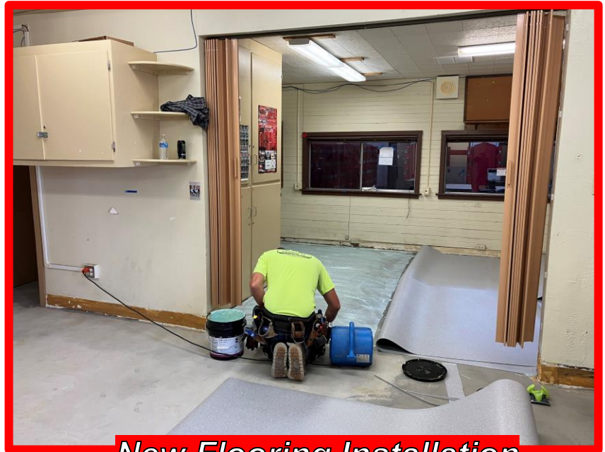
New Flooring Installation
