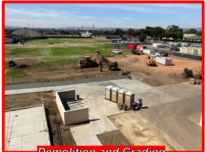
Demolition and Grading
