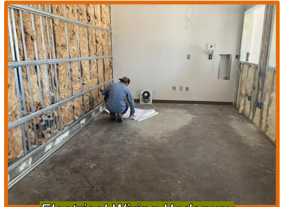
Electrical Wiring Underway
