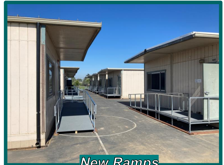
Assembling New Ramps
