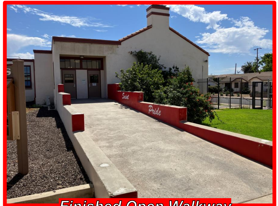
Finished Open Walkway
