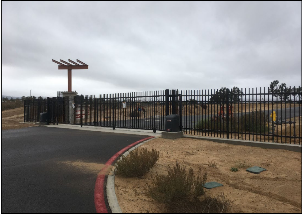
CTE / Ag Center – View of Entrance Gate from inside the Campus
