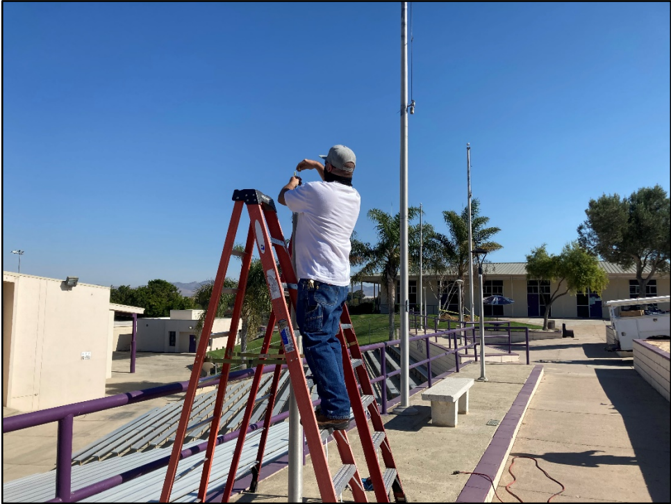
ERHS – Andy Freitas Installs New LED Lights in the Greek Theatre
