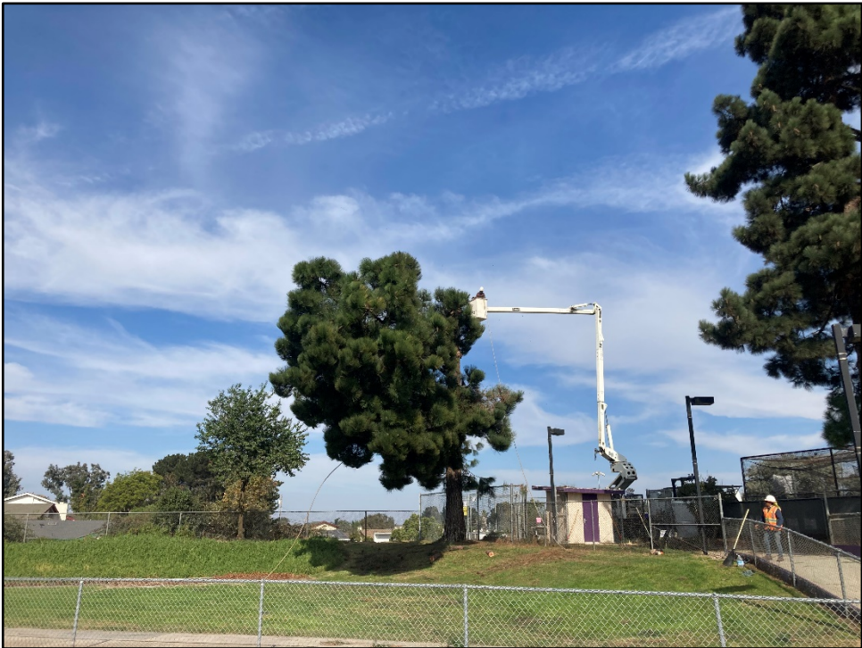
ERHS – Tree Removal In-progress near the Football Ticket Booth
