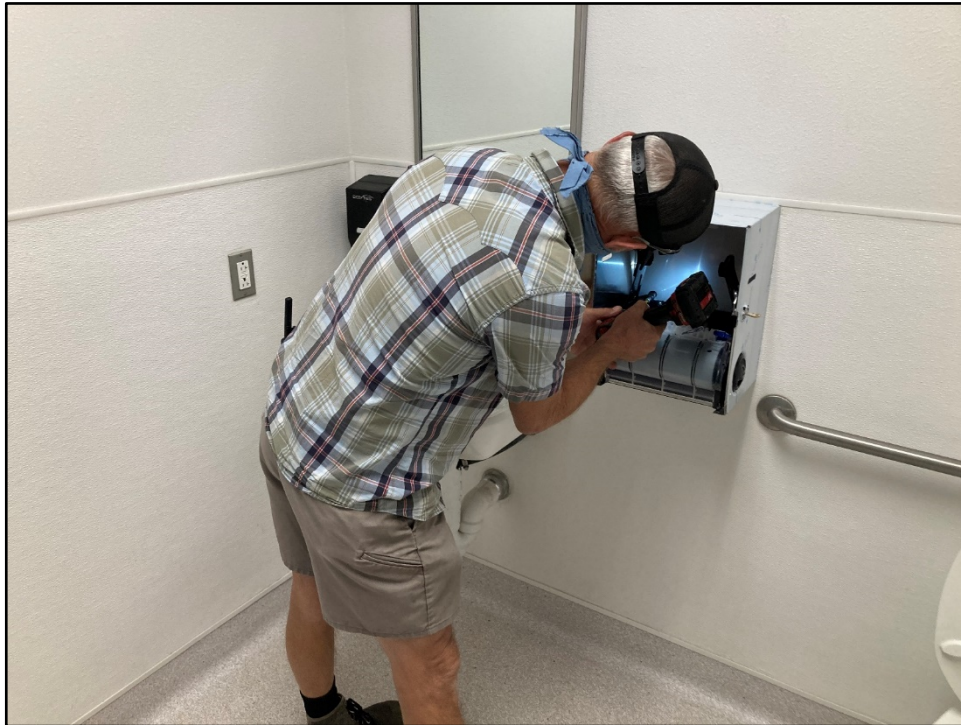
PVHS – Greg Parker Installs Paper Towel Dispensers to Comply with COVID-19 Guidance
