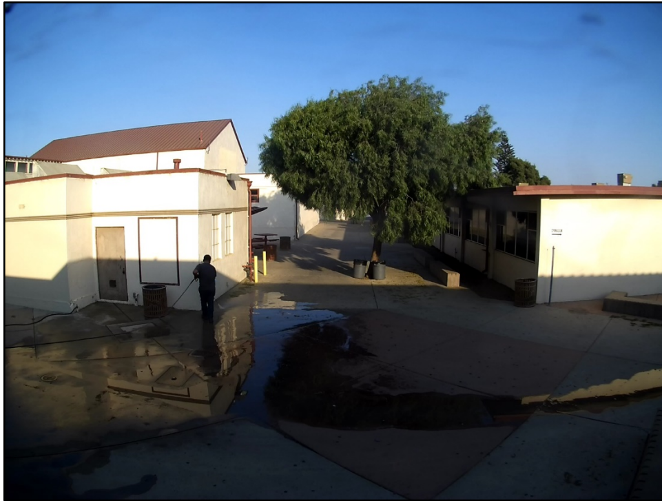
SMHS – Alex Banda Pressure Washes the Walkways at the Small Gymnasium
