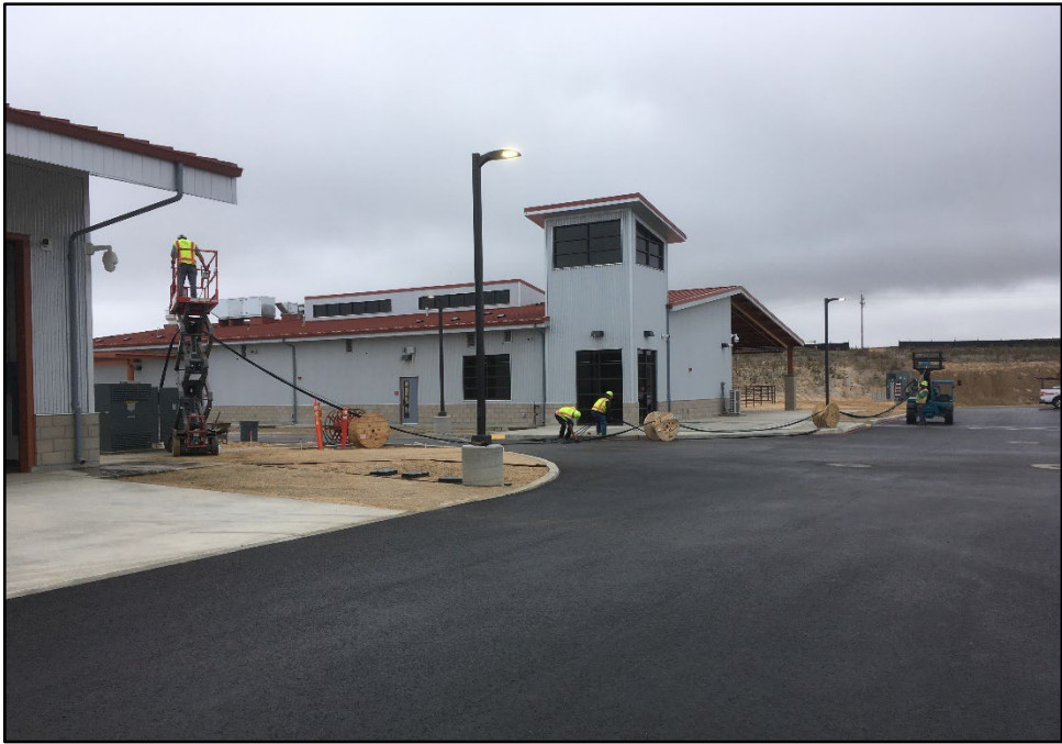
CTE / Ag Center – New Power Cable is Routed to the Transformer
