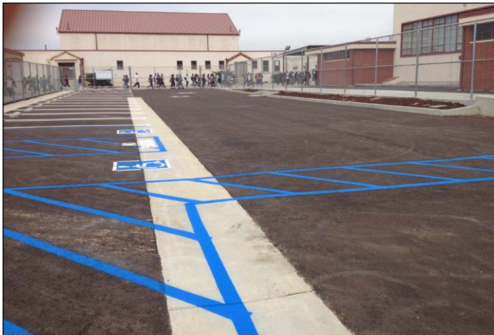
SMHS – Camino Colegio Parking Lot Paving Ready for Visitors
