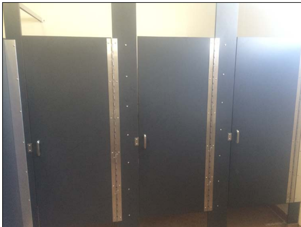
SMHS - New Restroom Partitions in the Girls' Locker Room
