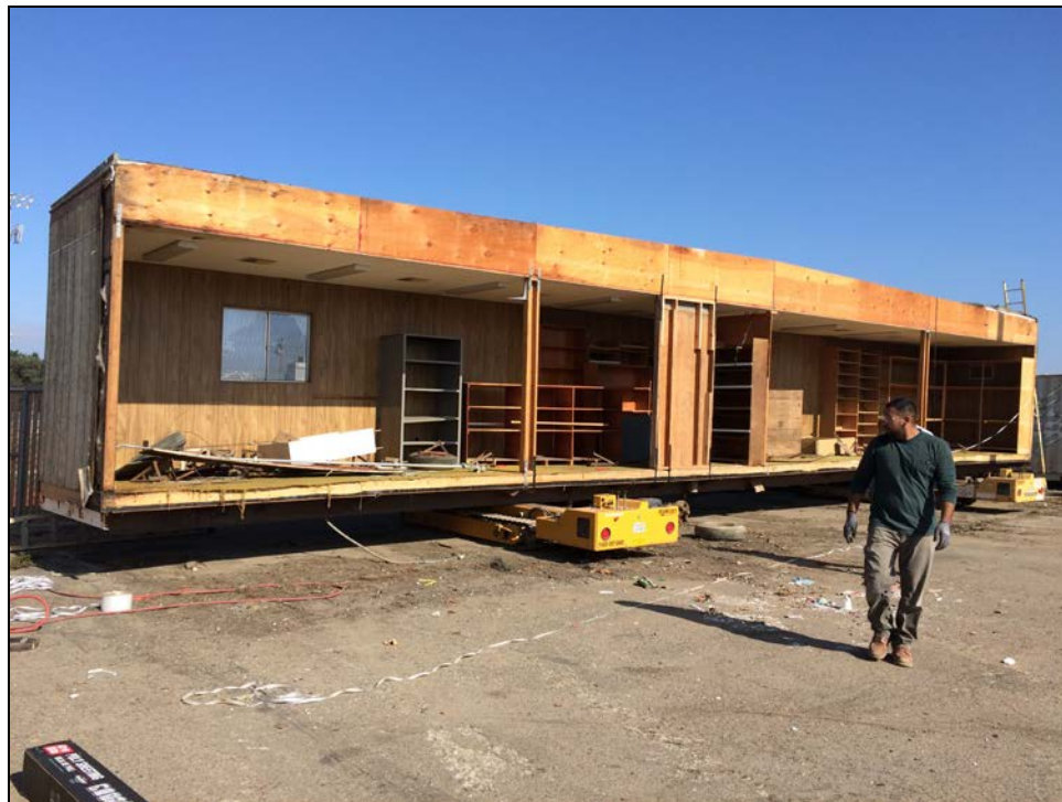
SMHS - Maintenance Equipment Storage Trailer is Prepared for Removal
