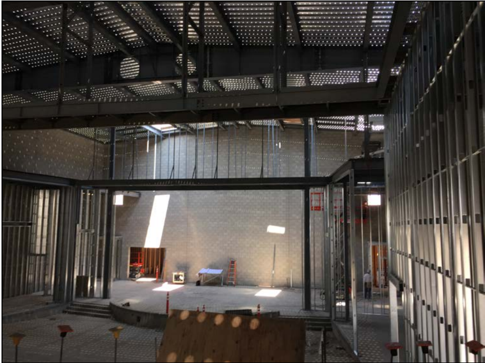
PVHS - Theater Catwalks in Progress and Roof Decking Complete
