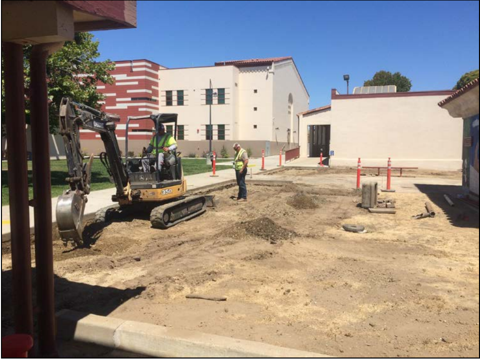
SMHS – New Walkway Under Construction near the Art Gallery
