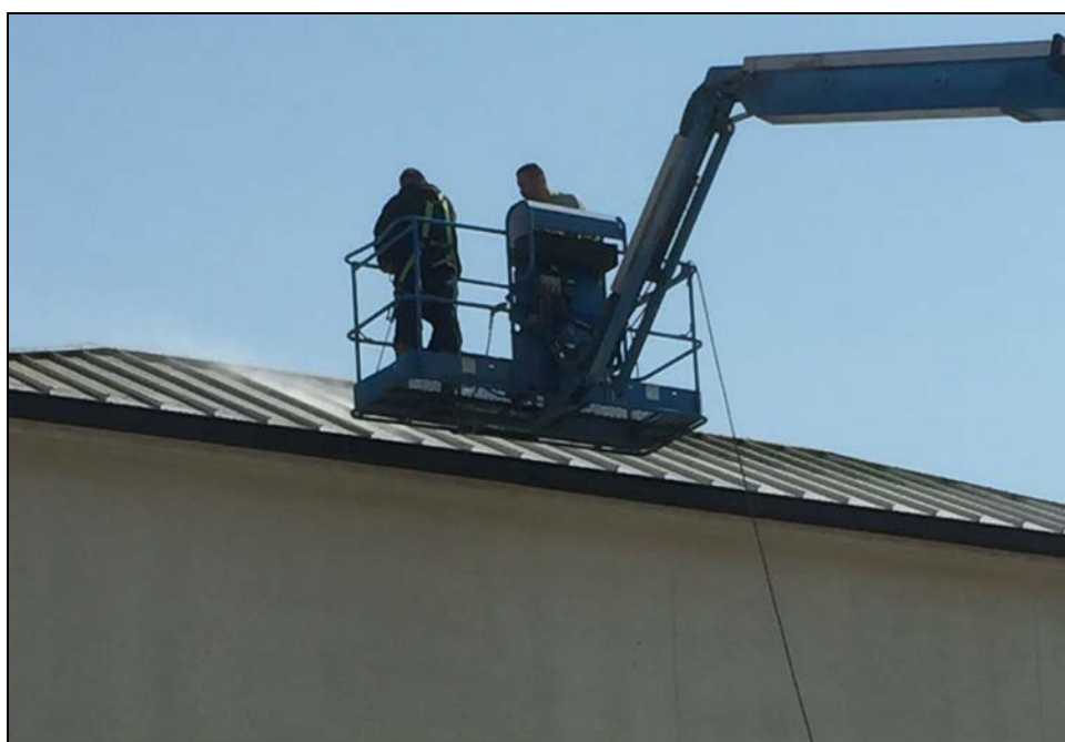
PVHS – Joe Mejia and Ruben Rodriguez Power Wash the Metal Roofs
