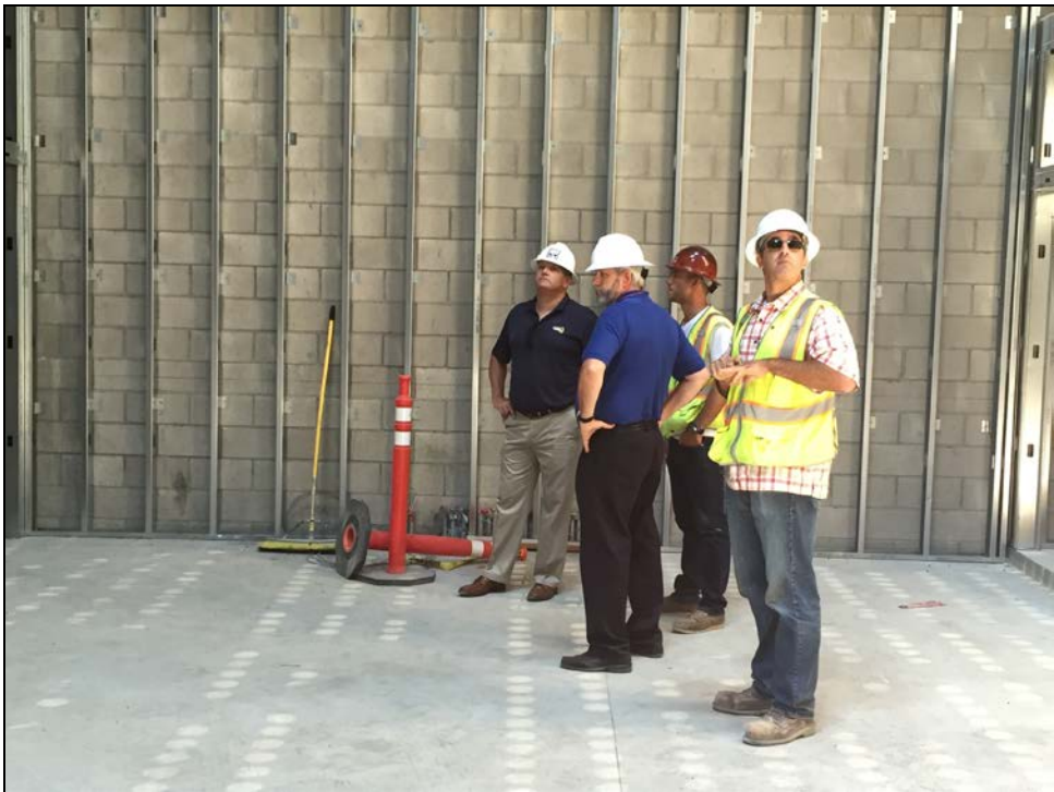
PVHS - Inspection Team Reviews Performing Arts Center Progress
