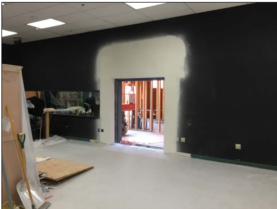
PVHS – Performing Arts Center Tie-in to Drama Classroom Nears Completion
