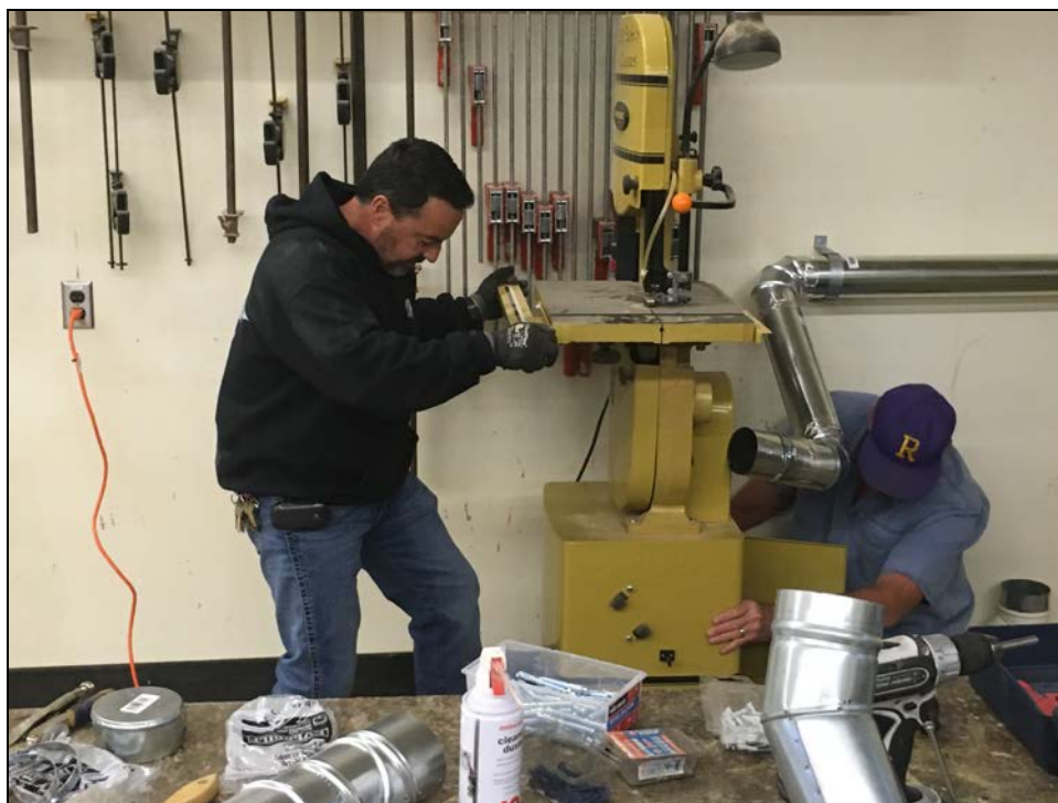
ERHS – Bernie Rayner and Gordon Greer Revise the Wood Shop Dust Collection System
