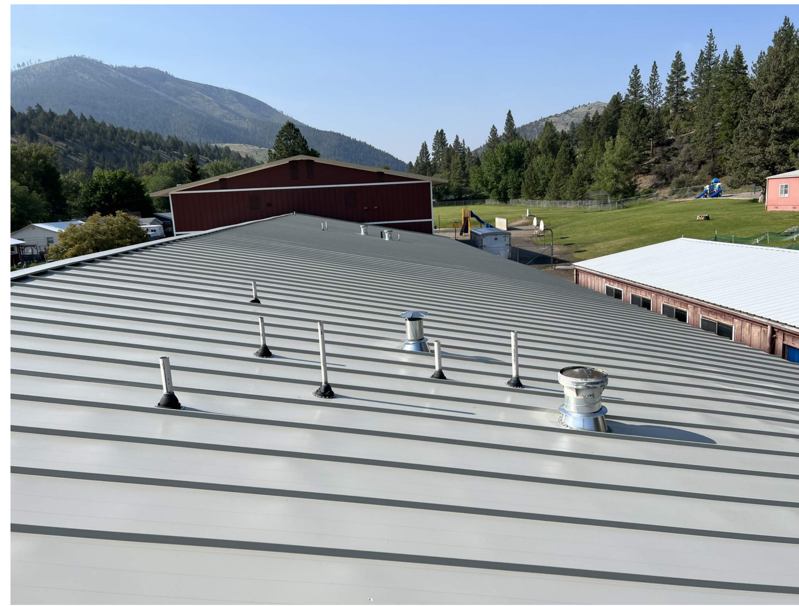
3 EXISTING PHOTO #2 A1.00
