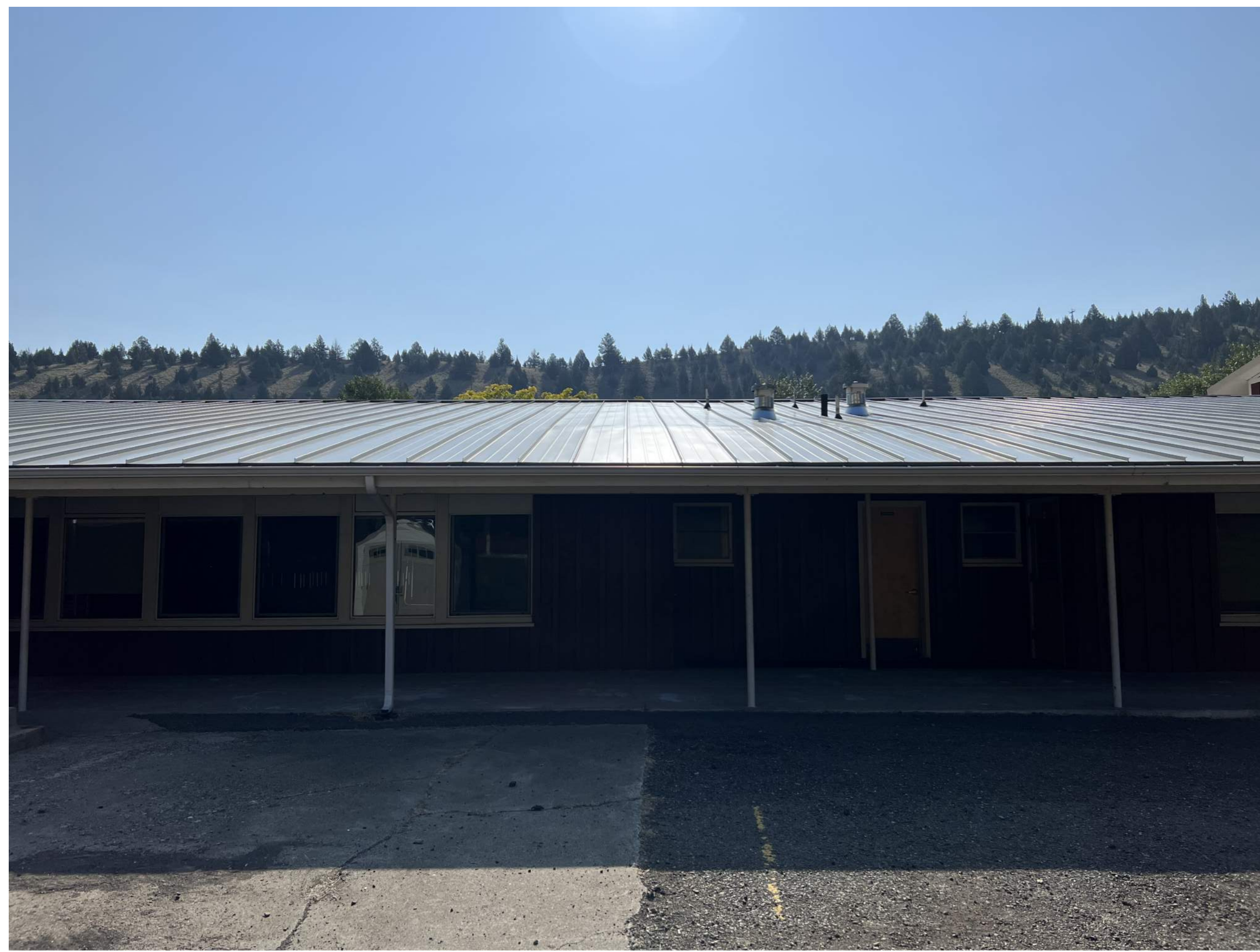
2 EXISTING PHOTO #1 A1.00
