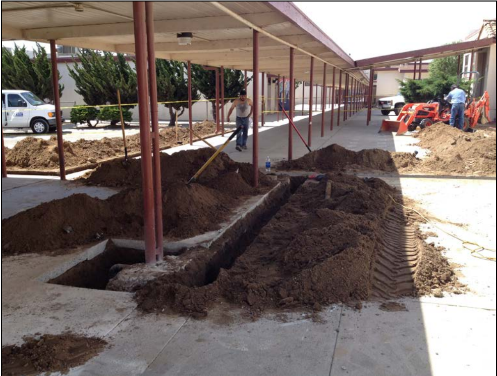
SMHS - José Placencia and Flavio Rodriguez Reroute a Natural Gas Line under the Covered Walkway
