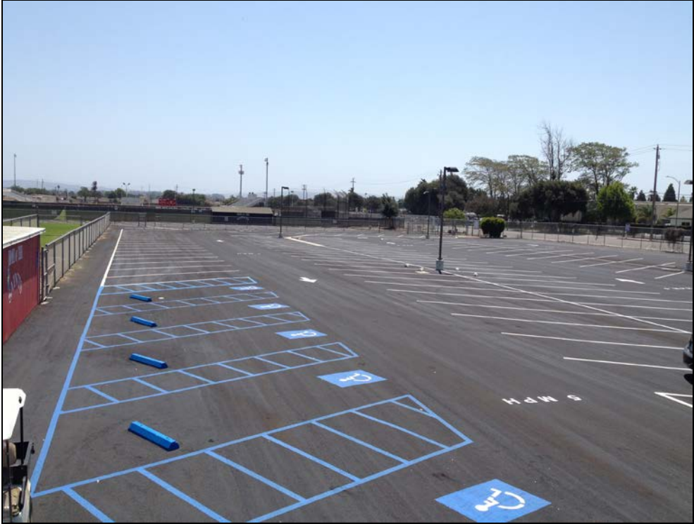
SMHS - Staff Parking Lot Slurry Sealed and Striped
