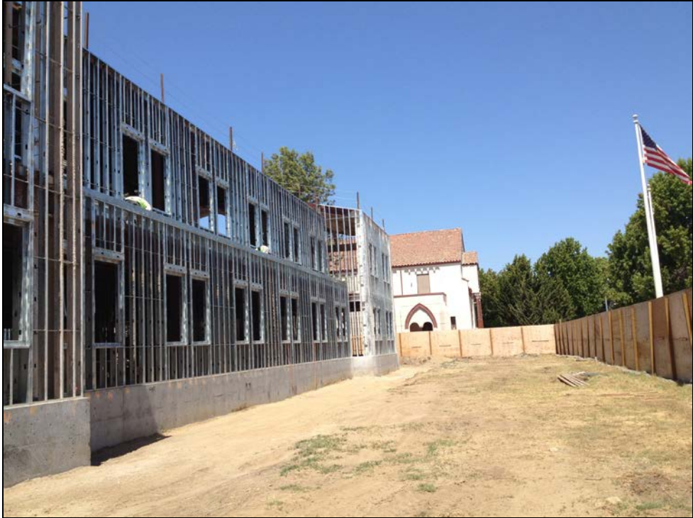
SMHS – 14 Classroom Building Metal Walls with Ethel Pope Auditorium in the Background
