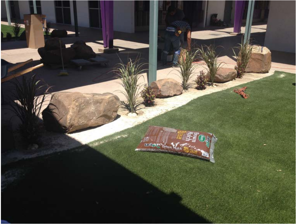
ERHS – Artificial Landscape Pilot Project is Complete
