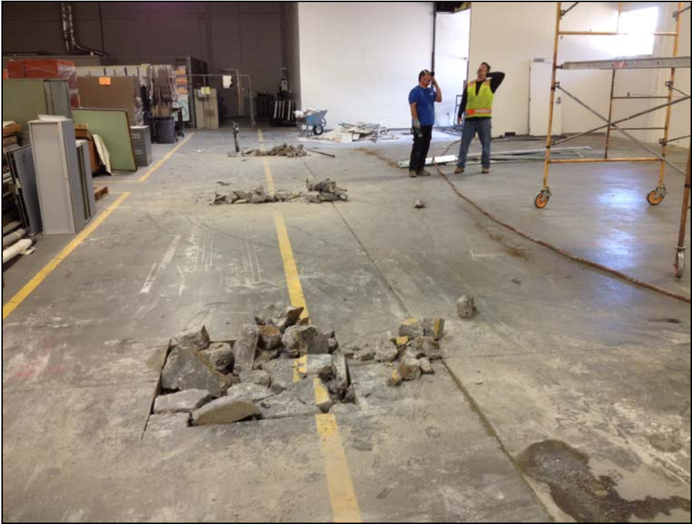
Support Services Center – Demolition begins for the Multipurpose Room
