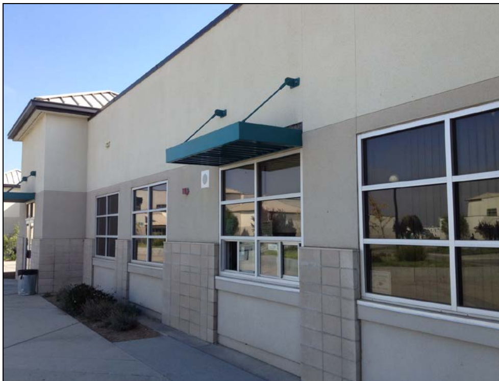
PVHS – New Canopies Installed over the Business Office and Attendance Office Windows
