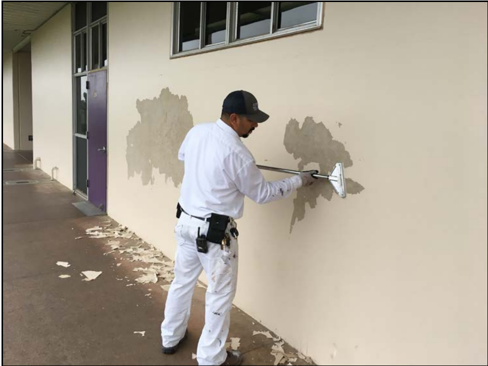
ERHS – Ernest Paz Prepares Classroom Exterior Walls for New Paint
