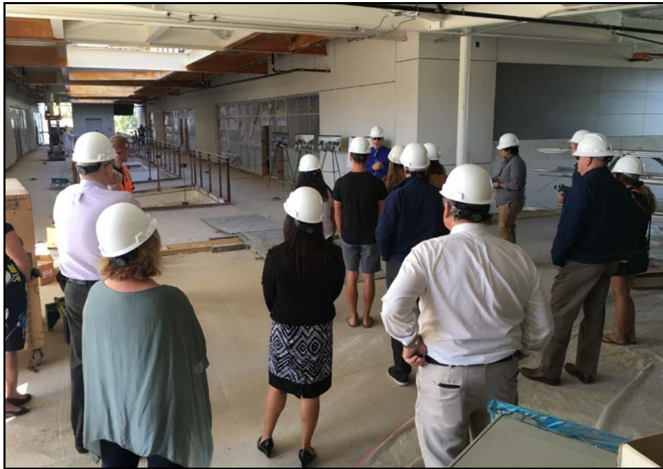
ERHS 38-Classroom Building – Gary Wuitschick Describes the Construction to School Board Members, Students, and the Press
