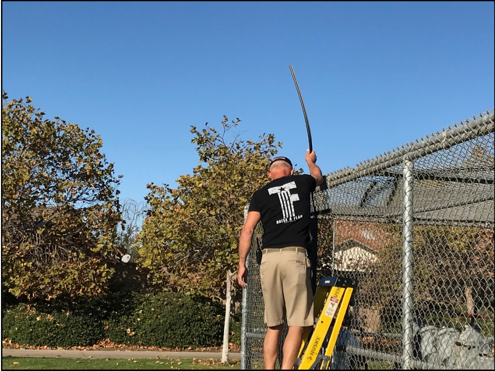
PVHS – Greg Parker Installs Privacy Slats at the Irrigation Well
