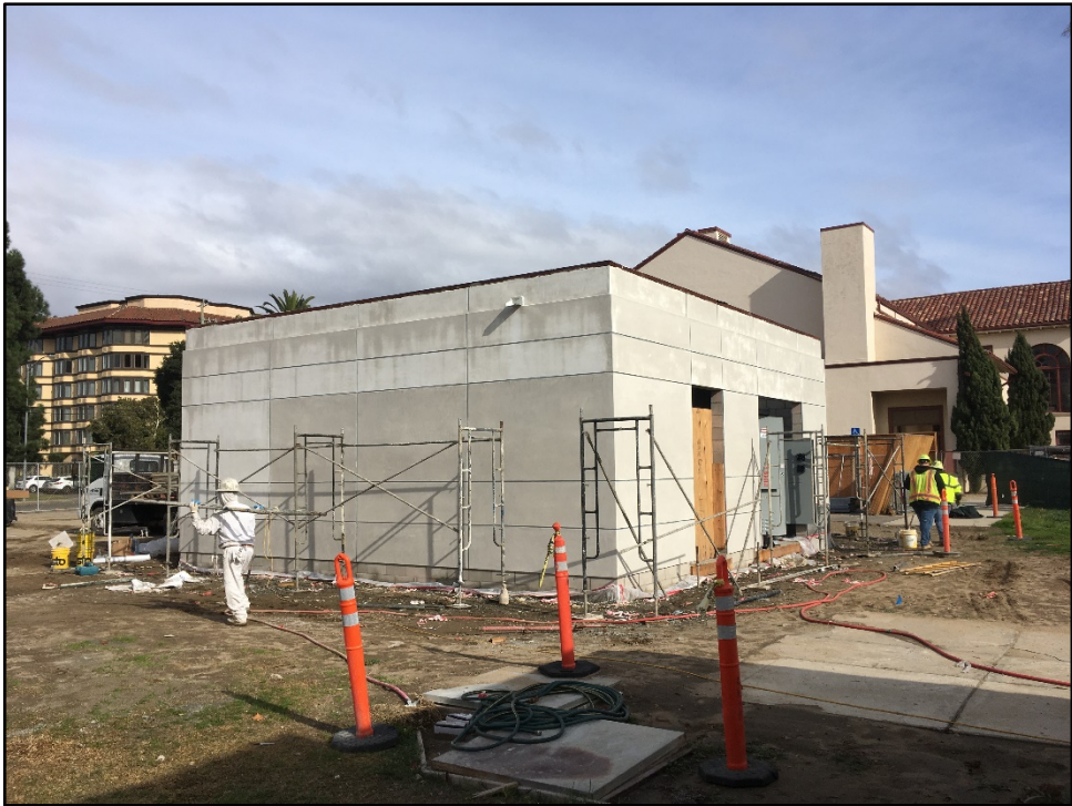
SMHS Reconstruction – Powerhouse Exterior Stucco In-progress
