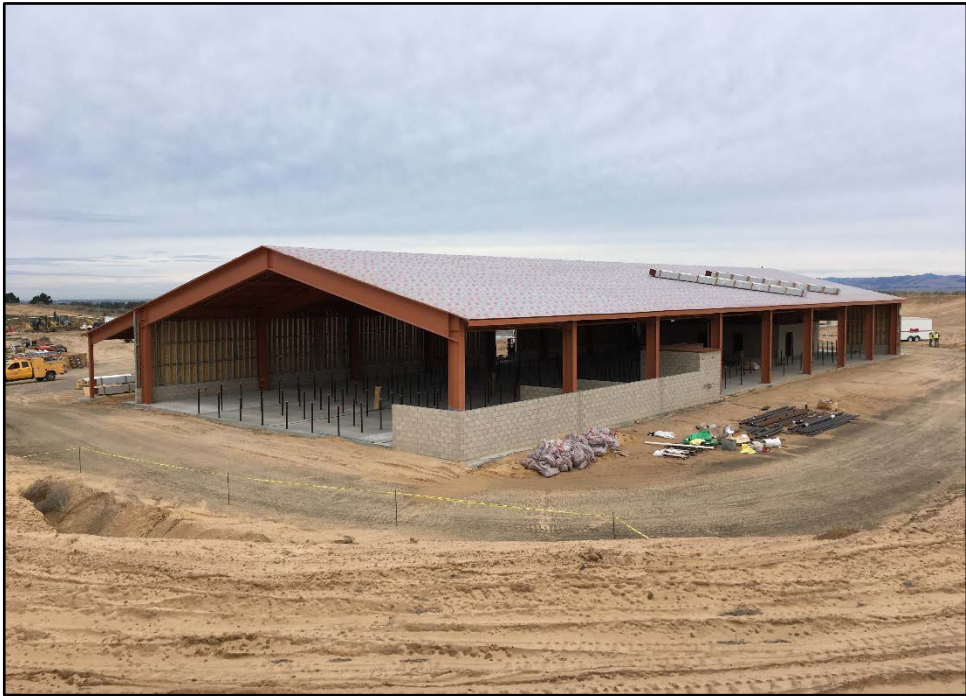
CTE Ag Center – View of the Barn from the South. Structural Metal is Painted and Metal Roofing Installation is In-progress
