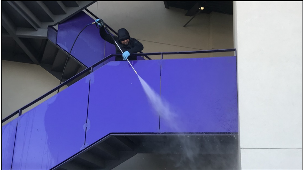
ERHS – Leo Avila Pressure Washes the Stairwell at the New Classroom Building
