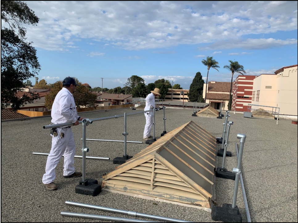
SMHS – Ernest Paz and Joel Amezcua Setup Skylight Protection on the Administration Building Roof
