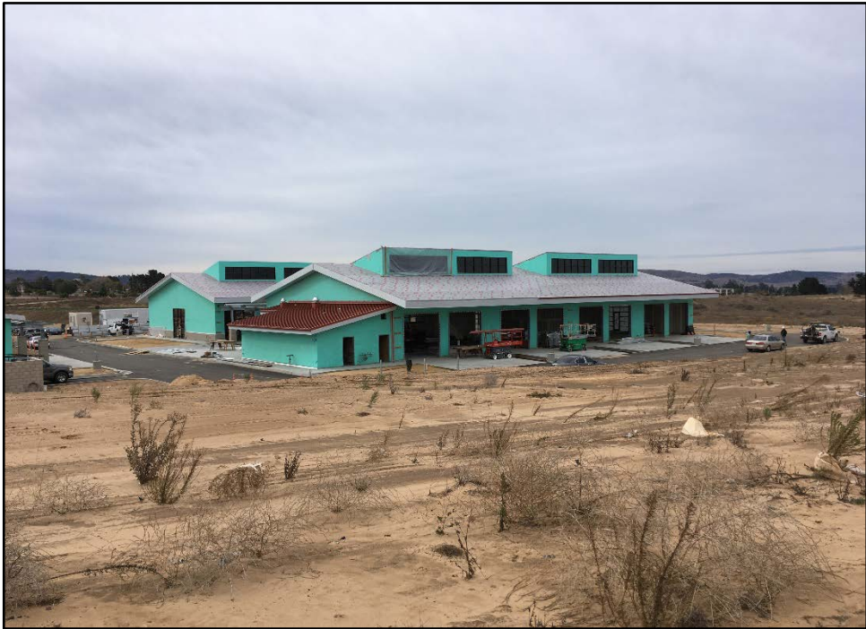
CTE Ag Center – Overview of Shop Buildings and Metal Roofing Installation Green Material is Fireproof and will be Covered by Metal and Masonry Siding
