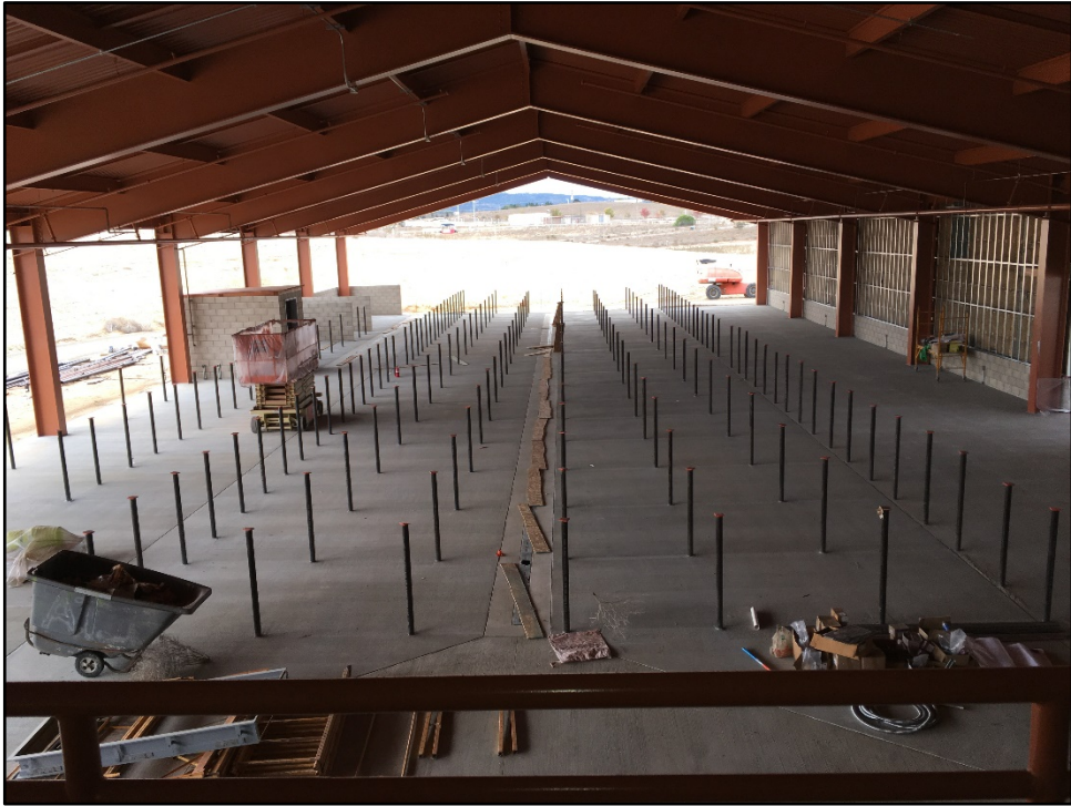
CTE Ag Center – Barn Interior: Livestock Pen Poles and Central Waste Drain are Visible
