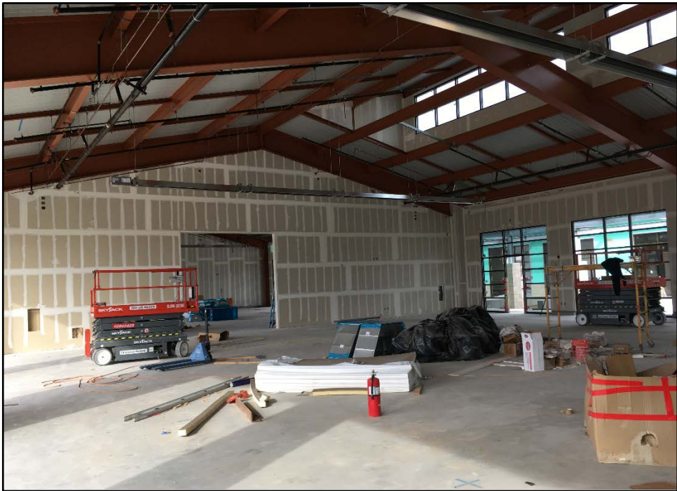
CTE Ag Center – Shop Interior Drywall Installation is Progressing
