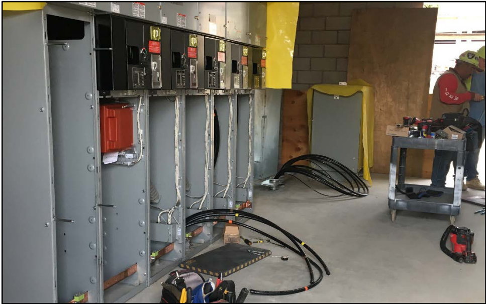
SMHS Reconstruction – Powerhouse Switchgear Installation Shows the Size and Complexity of the School 4160 Volt Power Distribution
