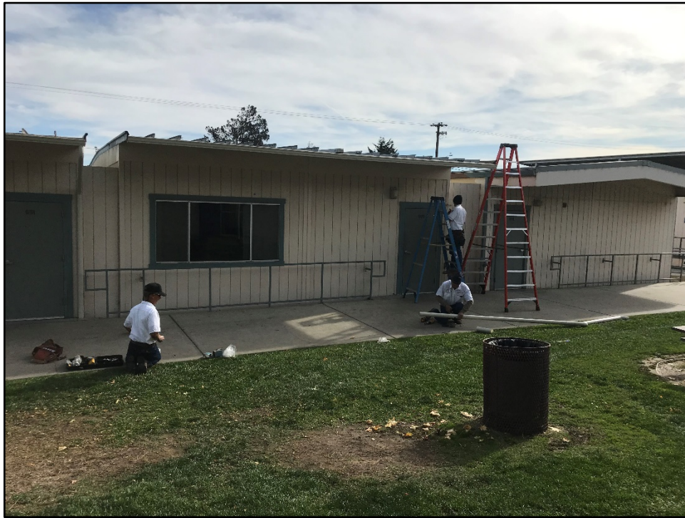
ERHS – Rain Gutter Replacement Underway on the Portable Classrooms
